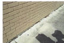
Left Side - Paving @ Building
