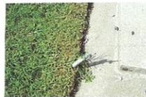
Rear - Cut Ground Wire
