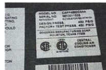
Air Handling Unit Plate
