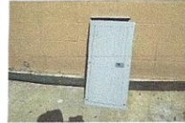
Rear - Removed Electrical Panel
