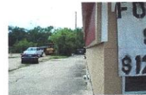
Left Side Cladding
