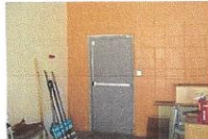
Rear Door - Interior
