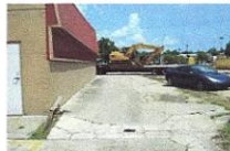
Left Paving with Drain Inlet
