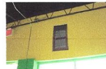
Front Wall - Opening
