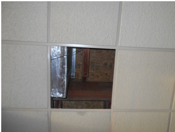
45. Wood frame and OSB decking
