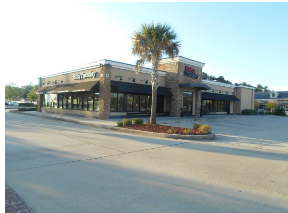
12. West side of the building
