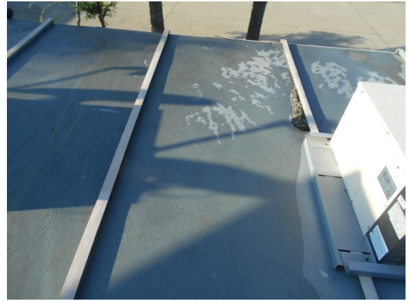
50. Metal roof above freezer
