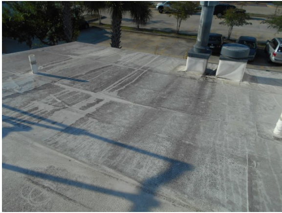
49. BUR modified bitumen roof with flood coat
