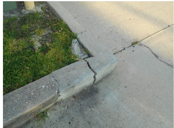
28. Cracked curbing
