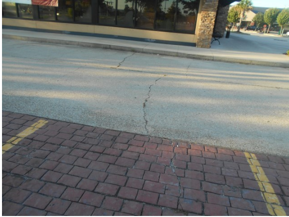
31. Cracked concrete
