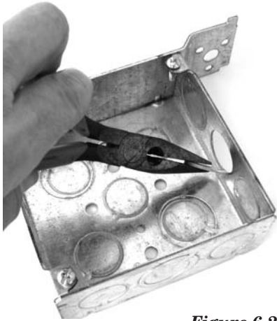
Figure 6-2 Removing knockout
