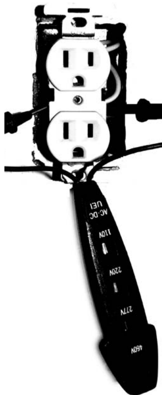
Figure 13-2 Testing receptacle at terminal screws with test light
