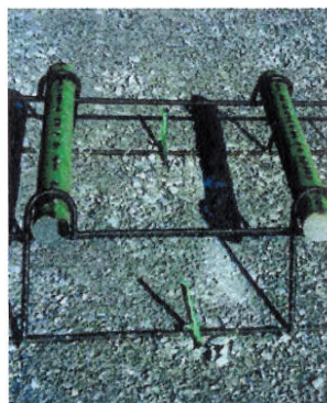
Staking dowel baskets (paver traveling ↓)
