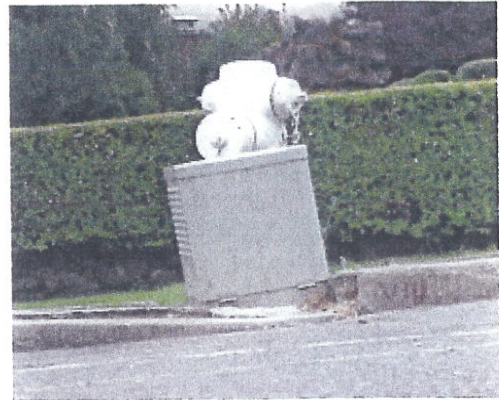
Wall added after hydrant installed
