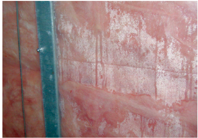
Photograph 9: Condensation on Polyethylene Vapor Barriers —Solar driven moisture out of reservoir claddings can lead to cavity side condensation on polyethylene vapor barriers in cold climates such as Chicago.
