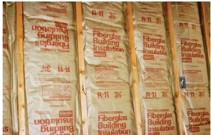
Photograph 11: Kraft-Faced Batt s—Bless old timers and common sense—the kraft facing breathes during the summer allowing inward drying—polyethylene vapor barriers do not.
