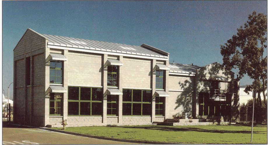
STRENGTH AND DURABILITY Split-face and standard concrete masonry units provide an attractive, strong, durable and cost-effective exterior for this pump station maintenance and storage building, San Diego, California. Kenniston & Mosher Architects, San Diego, used concrete masonry to achieve a deliberate expression for this utilitarian building.
