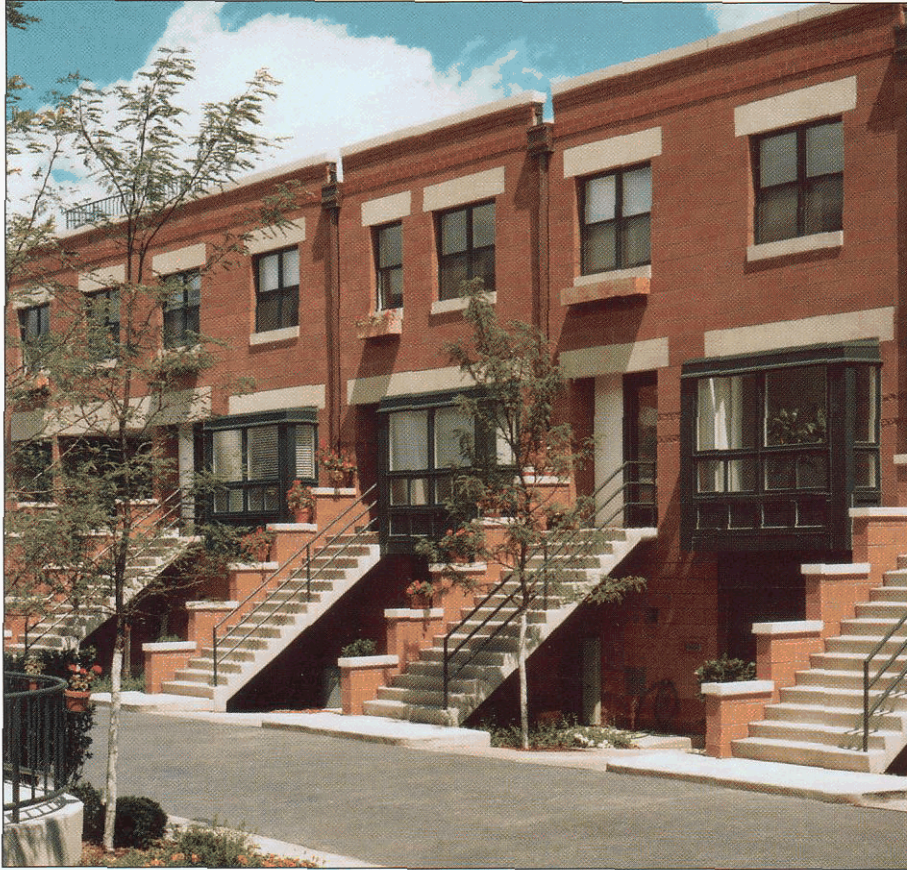
FIRE RESISTANCE The City Commons townhomes, Chicago, Illinois, has concrete masonry load bearing exterior and party walls for superior fire resistant construction. Architect Pappageorge/Haymes Ltd. selected integrally colored concrete masonry with accents of brick and limestone to give these townhomes the level of detail, scale, and warmth consistent with the surrounding neighborhood.
