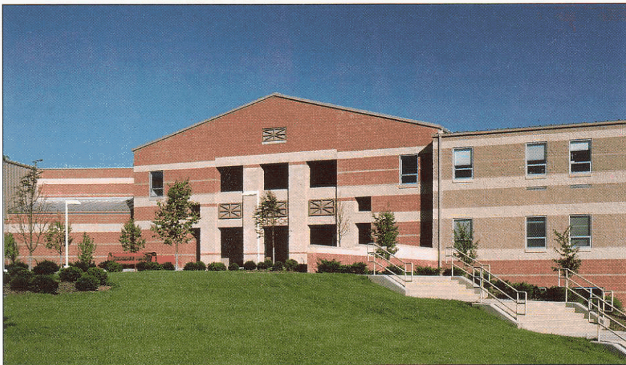
AESTHETIC APPEAL Concrete masonry was used for the exterior and interior walls of Big Walnut High School in Sunbury, Ohio for its structural capabilities, aesthetic appeal, durability, and reasonable cost. Architect Schooley Caldwell Associates, Columbus, Ohio, was able to achieve its design intent by integrating color, size, and texture into traditional forms.
