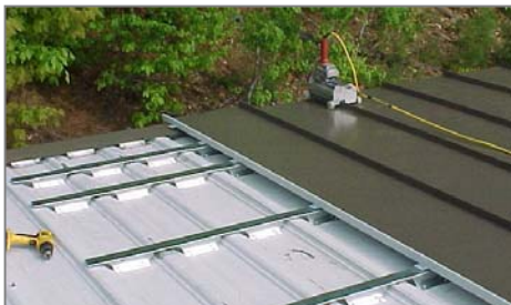
Courtesy of RoofHugger™, Inc.
