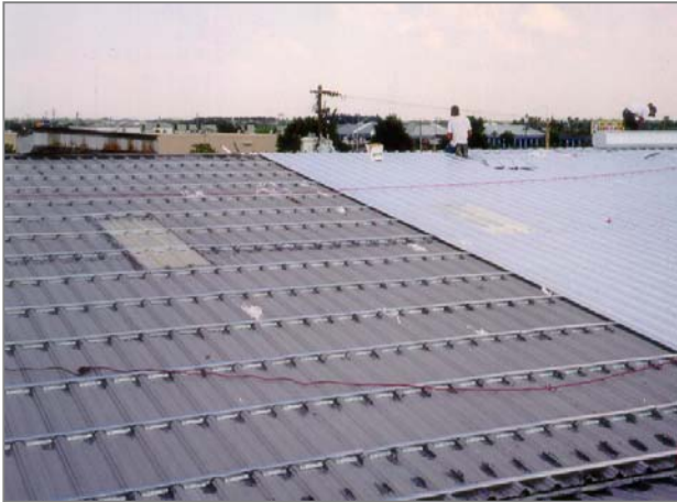
Courtesy of RoofHugger™, Inc.
