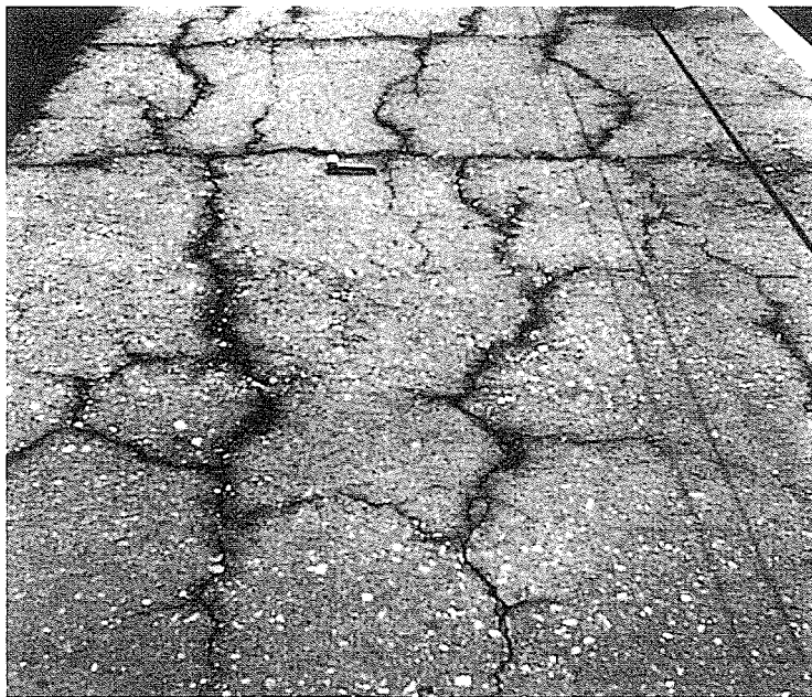
FIGURE 3.2.2.5(1). Mapping Cracking
