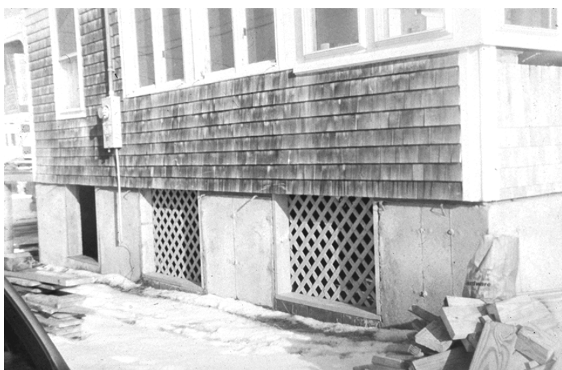
Figure 5-10: Building elevated on crawlspace with openings.
