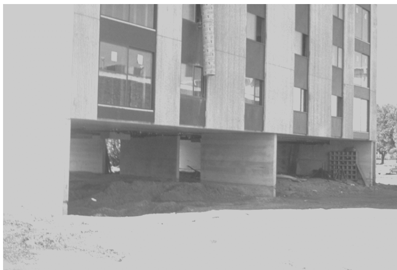
Figure 5-9: Building elevated on parallel stem walls.
