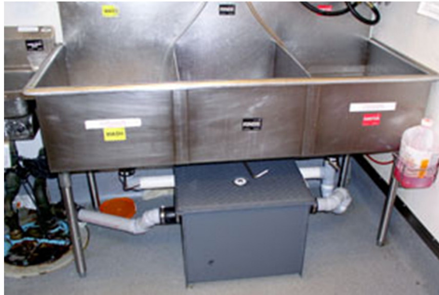
A 20 GPM, 40 lb hydro mechanical grease interceptor
