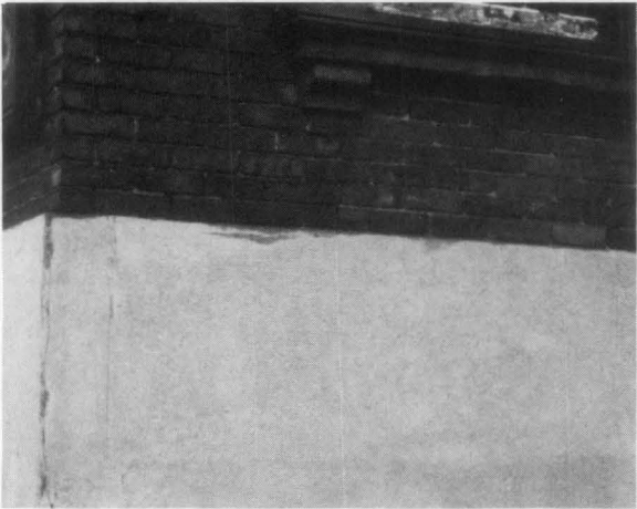
Parging over brick. Photograph: National Park Service.
