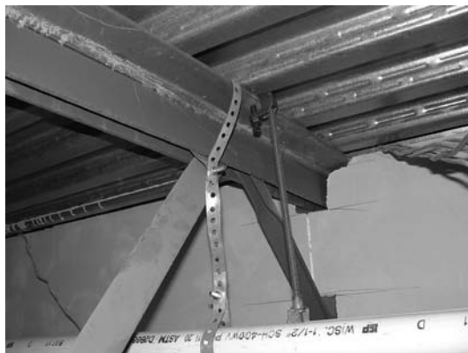
Fig. 7. Joist with crimped web members.
