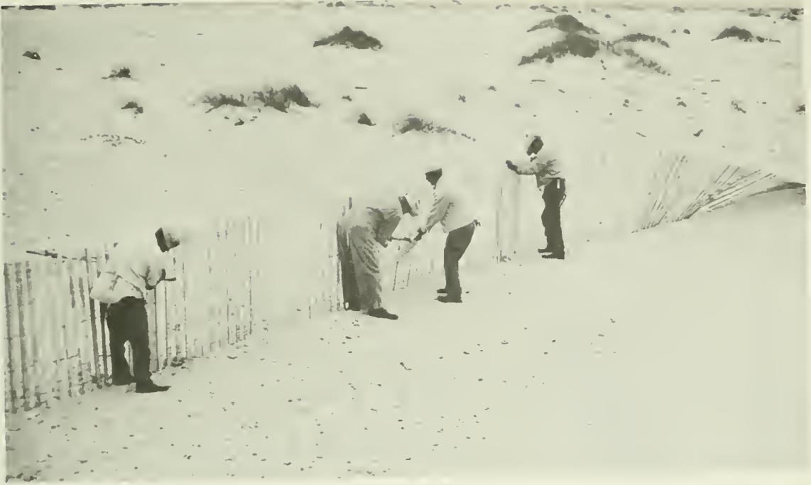
Figure 6-26. Erecting snow-type sand fencing.
