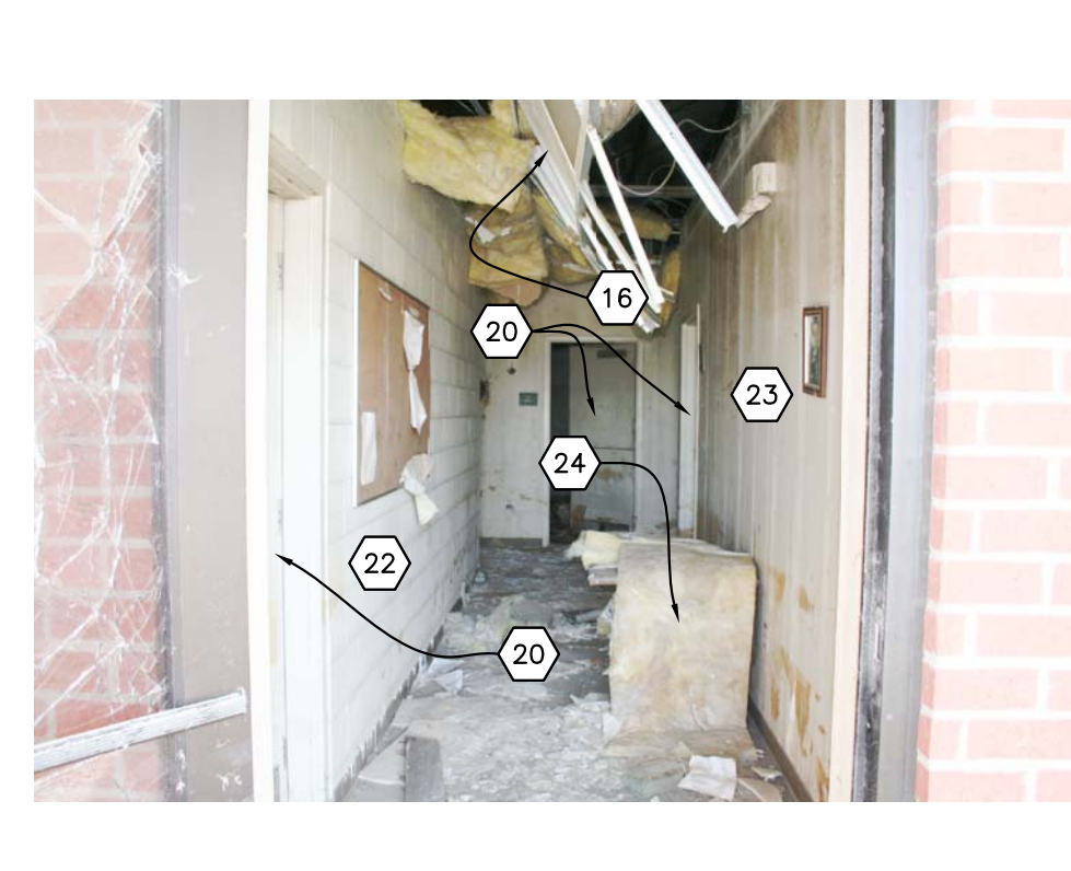
124 OMS 12 - CORRIDOR 114 INTERIOR PHOTOGRAPH
