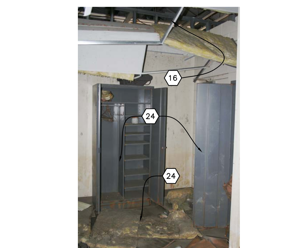
117 OMS 12 - LOCKER ROOM 107 INTERIOR PHOTOGRAPH
