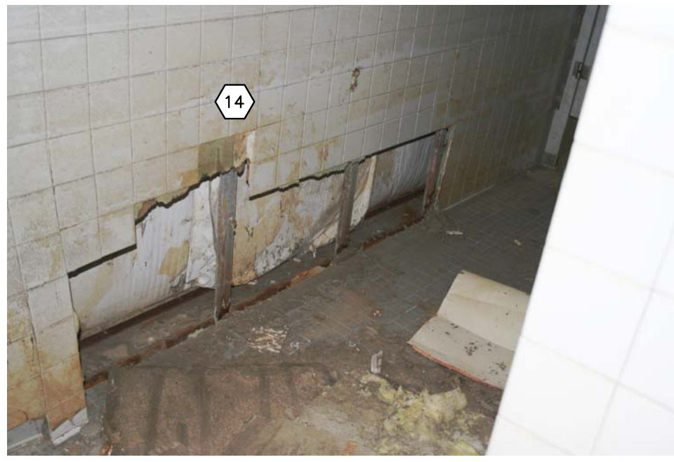
105 OMS 12 - MEN 101 INTERIOR PHOTOGRAPH
