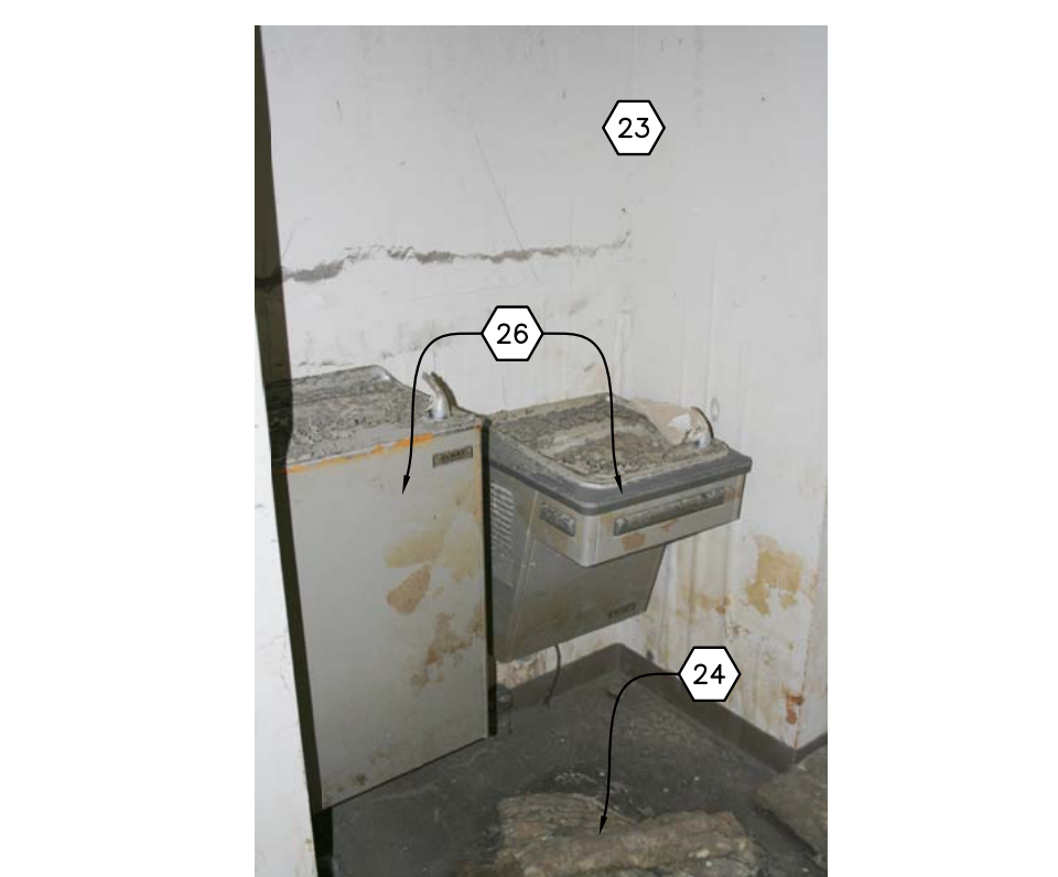
120 OMS 12 - CORRIDOR 111 INTERIOR PHOTOGRAPH
