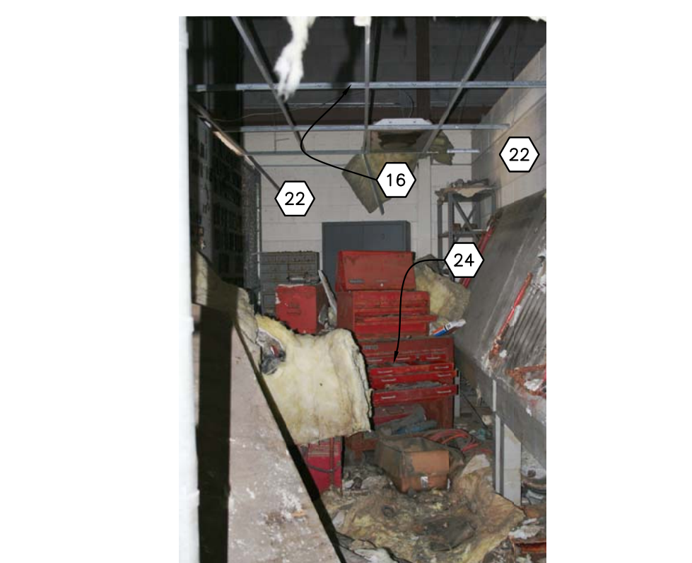
123 OMS 12 - TOOL ROOM 109 INTERIOR PHOTOGRAPH
