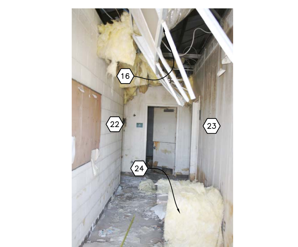
125 OMS 12 - CORRIDOR 111 INTERIOR PHOTOGRAPH
