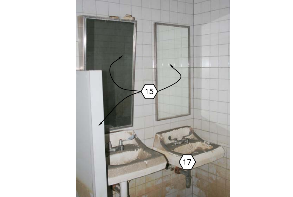
109 OMS 12 - MEN 101 INTERIOR PHOTOGRAPH
