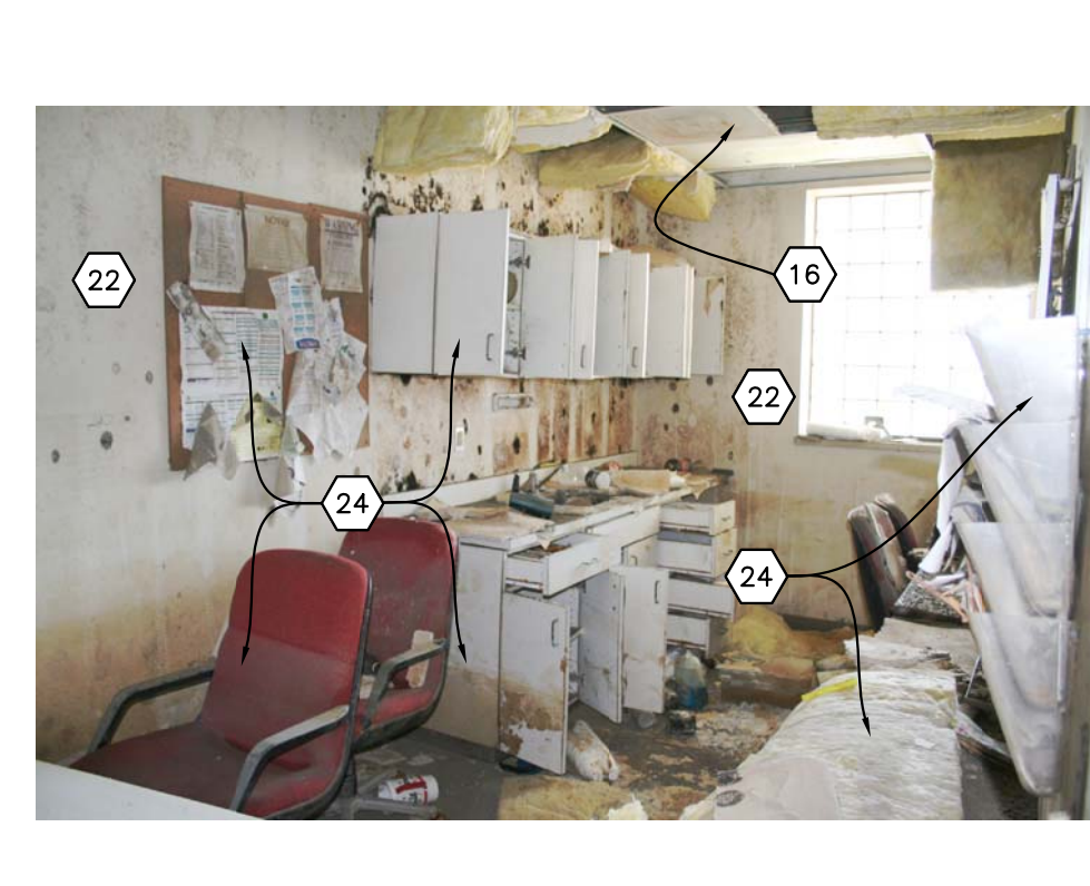
128 OMS 12 - BREAK ROOM 110 INTERIOR PHOTOGRAPH
