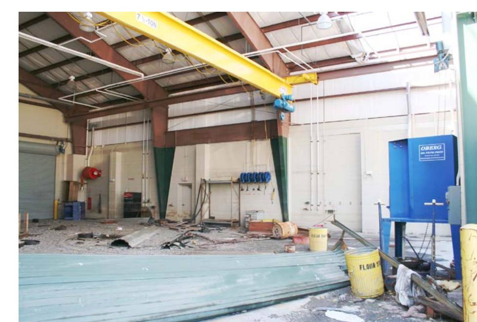
153 OMS 12 - WORK SHOP 121 INTERIOR PHOTOGRAPH
