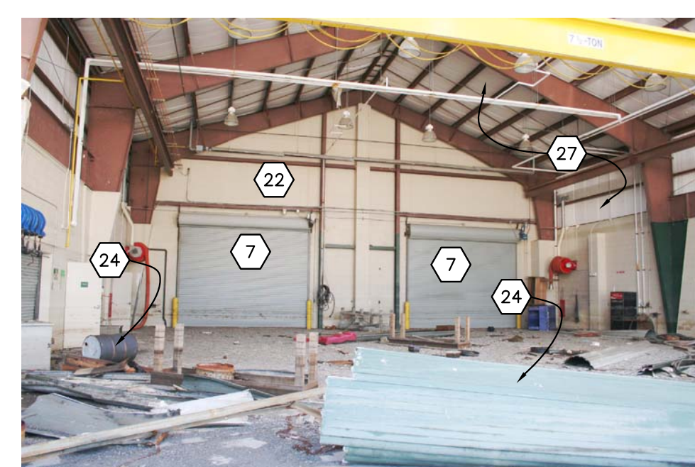
157 OMS 12 - WORK SHOP 121 INTERIOR PHOTOGRAPH
