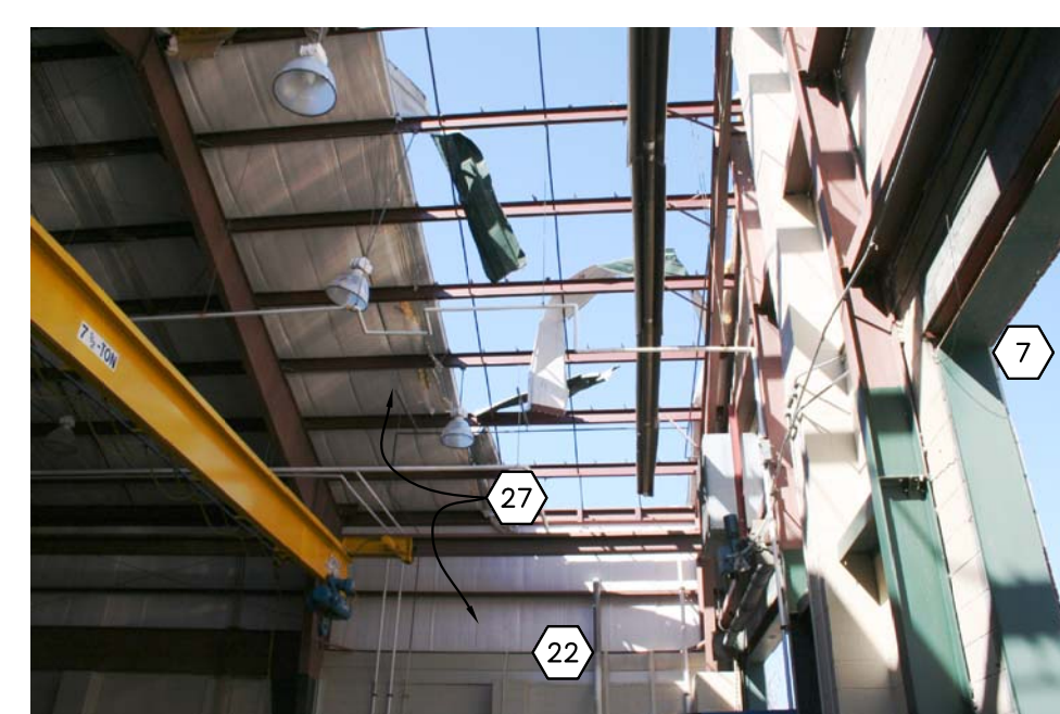
156 OMS 12 - WORK SHOP 121 INTERIOR PHOTOGRAPH
