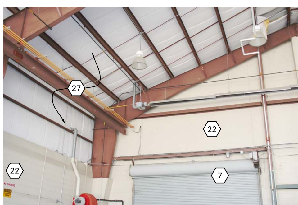
150 OMS 12 - WORK SHOP 121 INTERIOR PHOTOGRAPH
