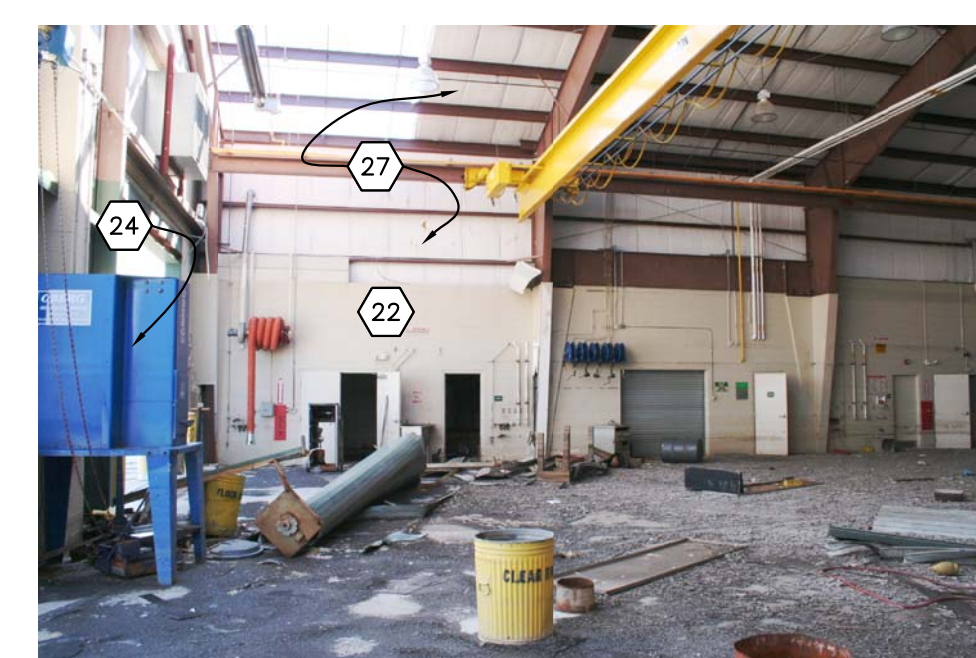
158 OMS 12 - WORK SHOP 121 INTERIOR PHOTOGRAPH
