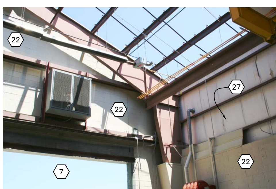
155 OMS 12 - WORK SHOP 121 INTERIOR PHOTOGRAPH
