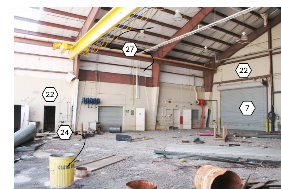
159 OMS 12 - WORK SHOP 121 INTERIOR PHOTOGRAPH
