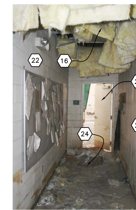
138 OMS 12 - CORRIDOR 117 INTERIOR PHOTOGRAPH
