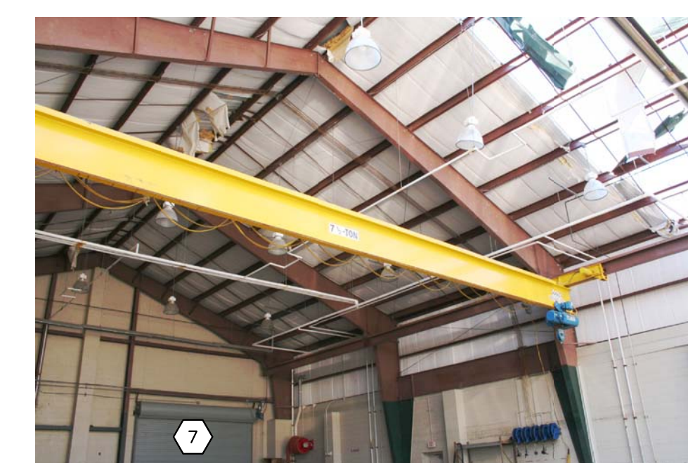
154 OMS 12 - WORK SHOP 121 INTERIOR PHOTOGRAPH
