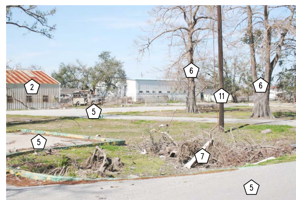
028 SITE DEMOLITION PHOTO
