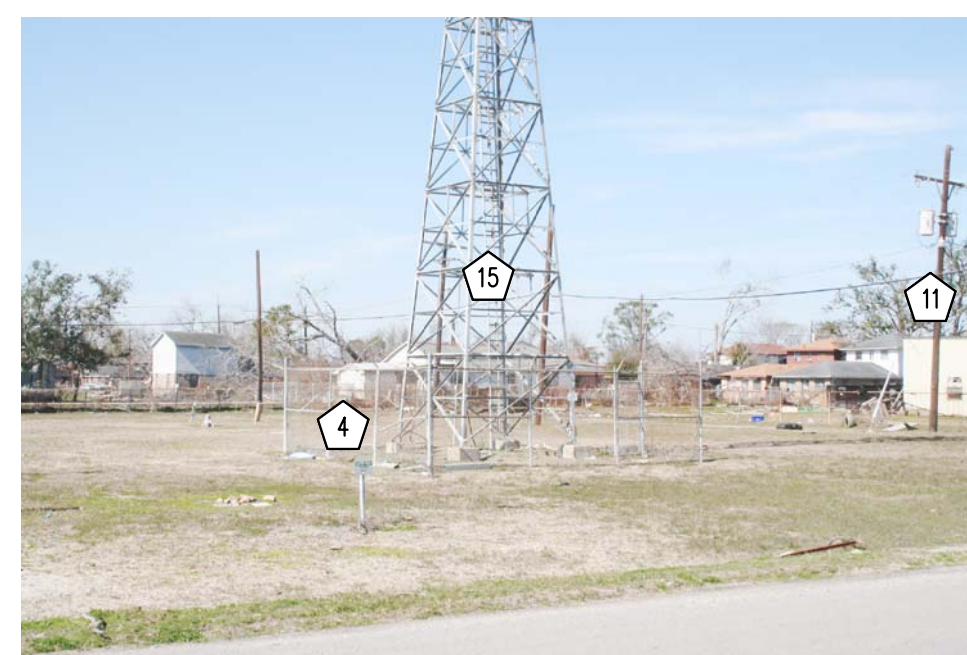
032 SITE DEMOLITION PHOTO
