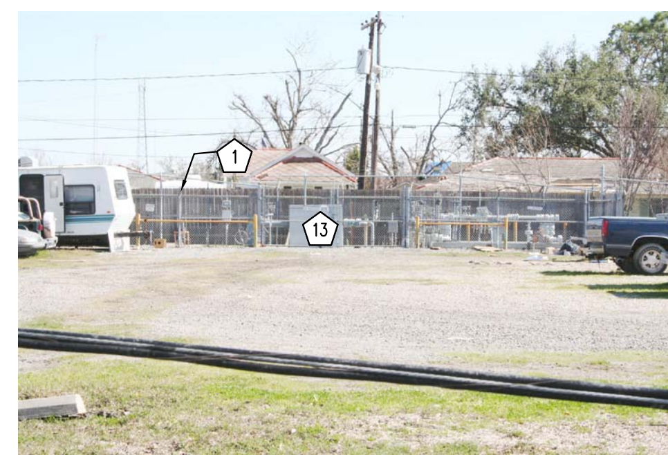
010 SITE DEMOLITION PHOTO
