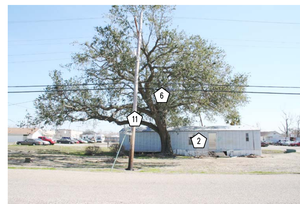
004 SITE DEMOLITION PHOTO BUILDING #285
