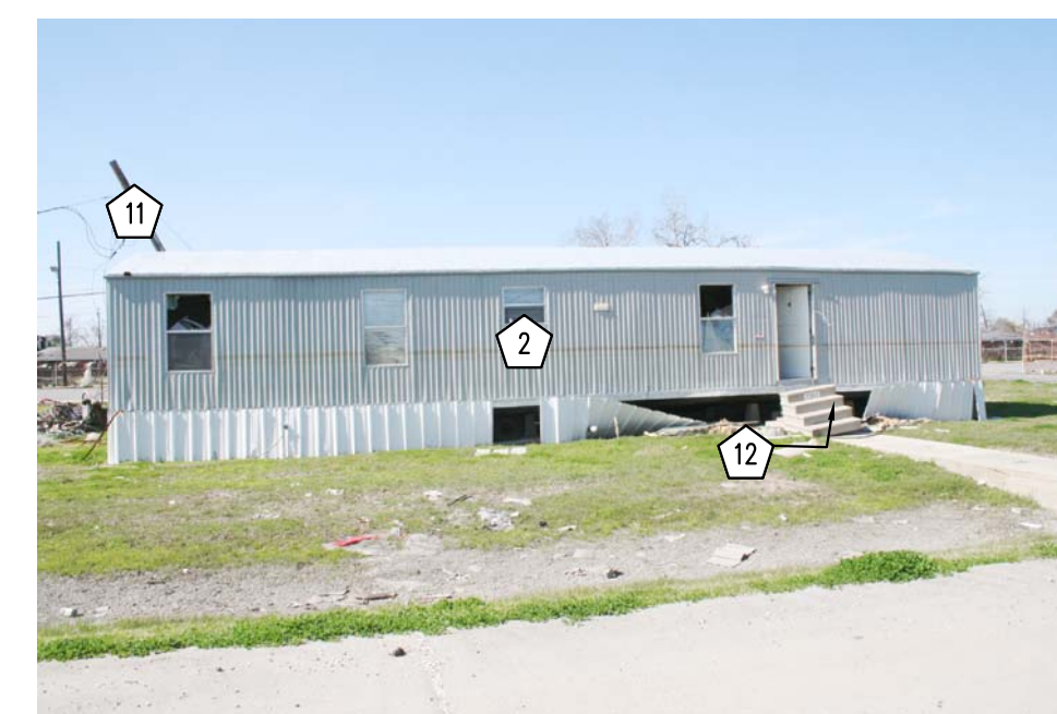
048 SITE DEMOLITION PHOTO BUILDING #361
