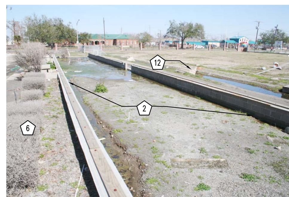
019 SITE DEMOLITION PHOTO FOUNDATION OF BUILDING #233
