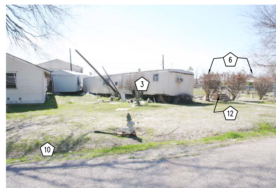
009 SITE DEMOLITION PHOTO BUILDINGS #212, 1259, & 1258 (LEFT TO RIGHT)
