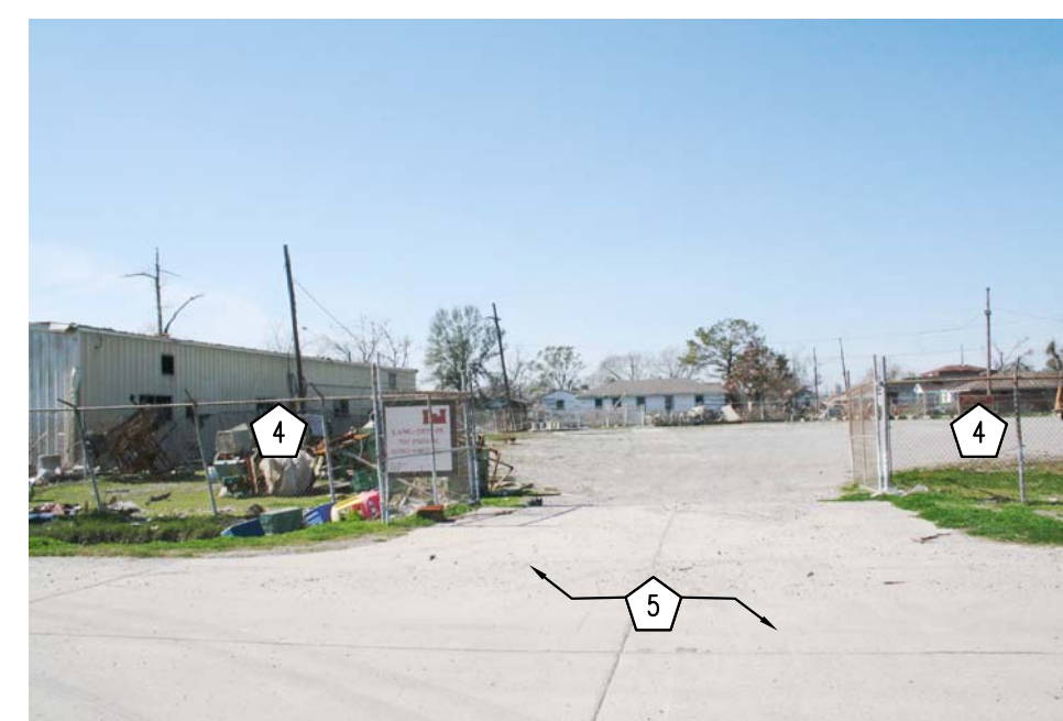
044 SITE DEMOLITION PHOTO BUILDING #310 (N.I.C.)
