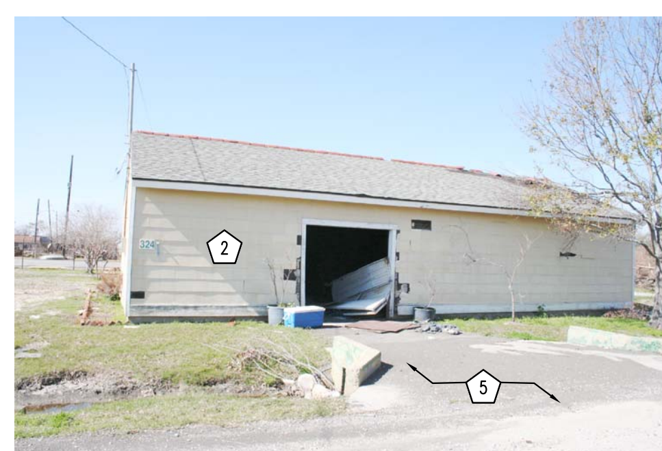
056 SITE DEMOLITION PHOTO BUILDING #324
