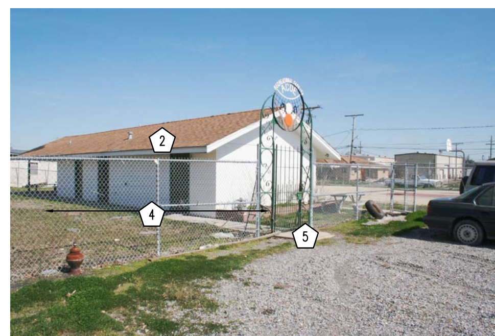
015 SITE DEMOLITION PHOTO BUILDING #224
