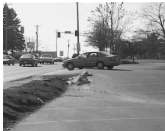
High-grade driveway on an older-configuration arterial route in Des Moines, Iowa—grade change forces the motorist to reduce speed to negotiate driveway
