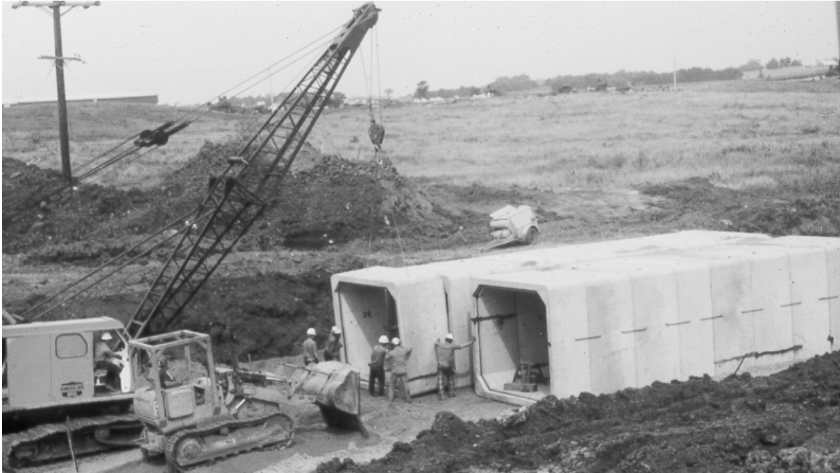
Figure VI-25--Precast Double Barrel Box Culvert
