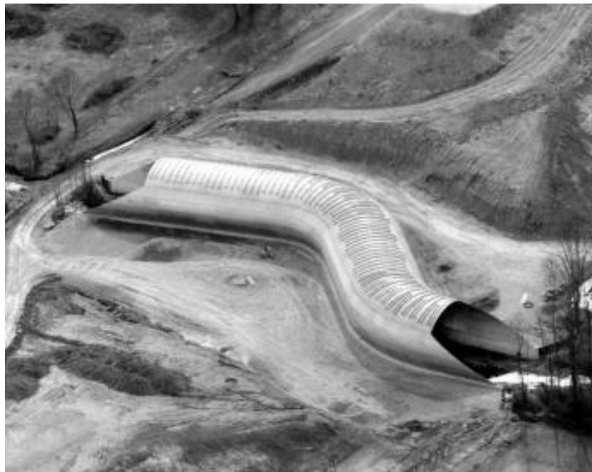
Figure VI-4--Culvert with a Horizontal Bend (Contech)
