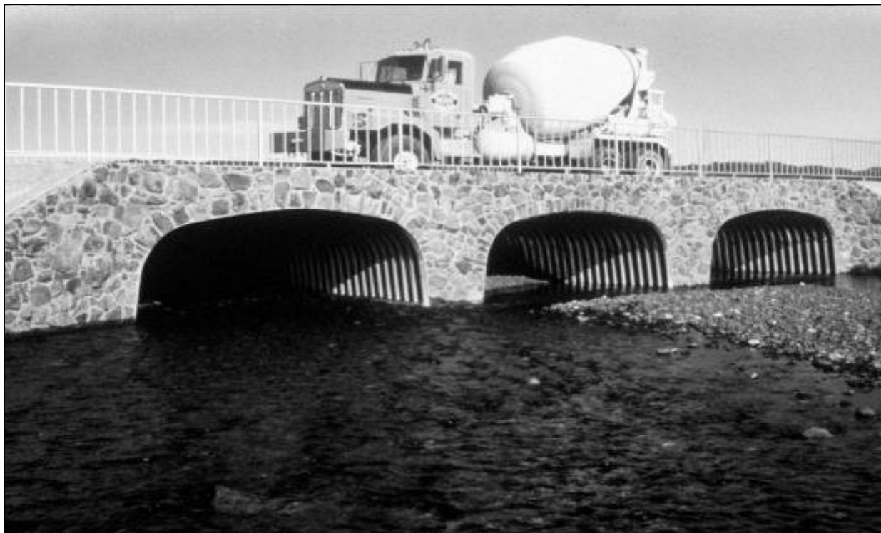
Figure VI-24--Corrugated Metal Box Culvert (Contech)
