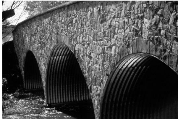
Figure I-6--Corrugated Metal Arch (Contech)
