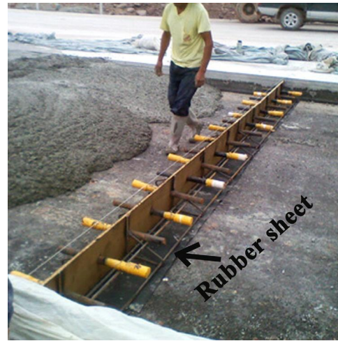
FIG. 3 Rubber sheet installed at the concrete pavement joint as interlayer.
