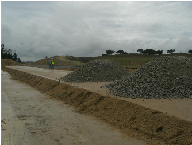
FIG. 6 General overview of SC trial layer.
