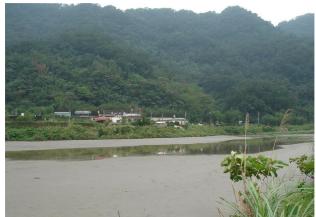
FIG. 2 Retention pond has been fully filled with dredged reservoir siltation.
