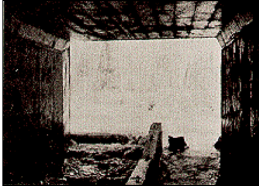
Figure VI-7--Fish Baffles in Culvert
