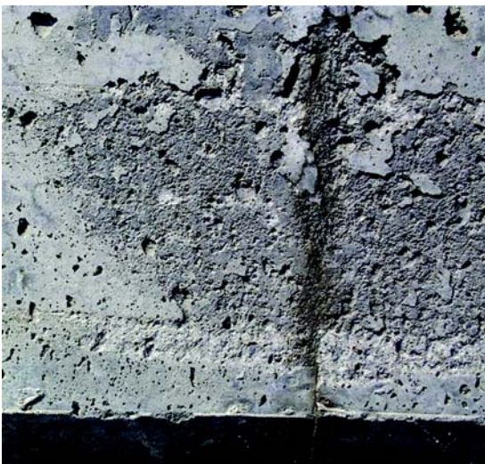
Fig. 2.2.19.2—Medium scaling.
