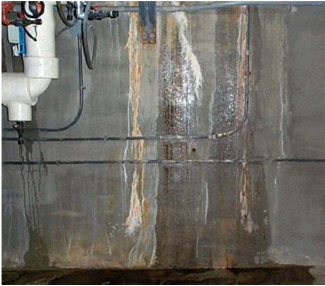
Fig. 2.2.14.1—Leakage, liquid.
