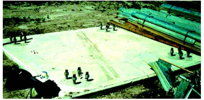
Fig. 2.1.2.12—Temperature cracking.
