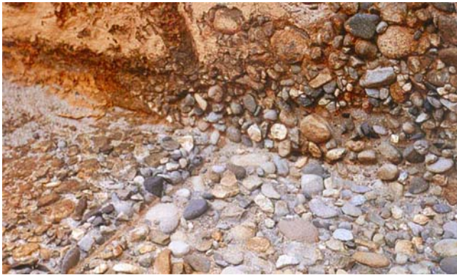
Fig. 2.2.6(b)—Disintegration from chemical attack.
