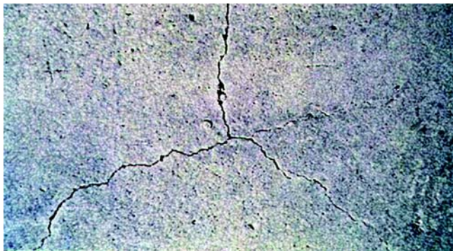
Fig. 2.1.2.11—Shrinkage cracking.
