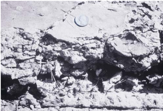
Fig. 2.2.6(a)—Disintegration.
