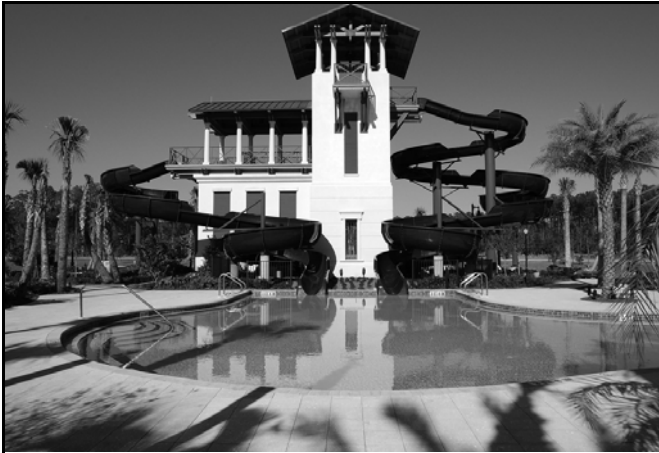
FIGURE 202(8) CLASS D-3, CATCH POOL (Photo courtesy of Tolomato Community Development District—Novatee)
