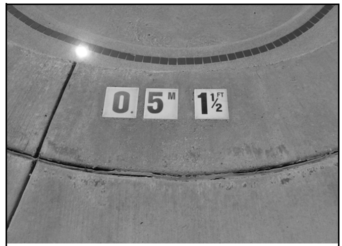
FIGURE 409.3 DEPTH MARKER ON POOL DECK
