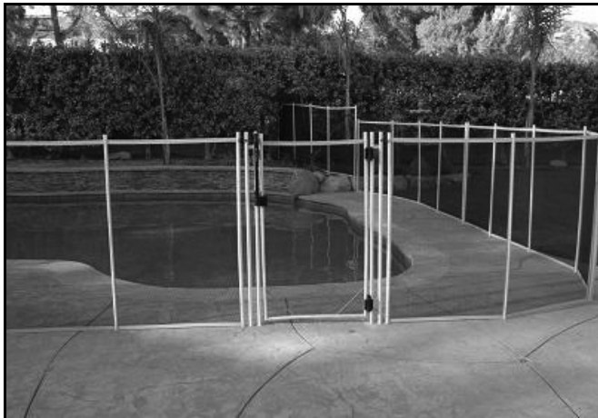
FIGURE 305.2.4 MESH FENCE AS A STRUCTURE- TO-POOL BARRIER
