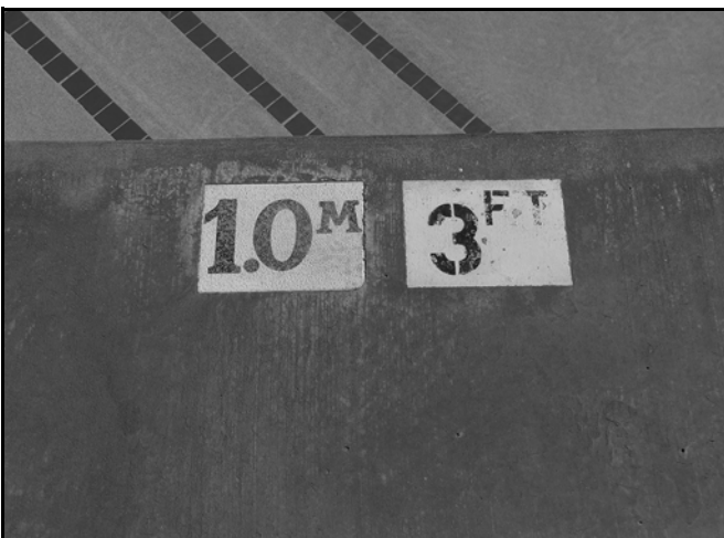
FIGURE 409.2.5 DEPTH MARKER ON POOL DECK
