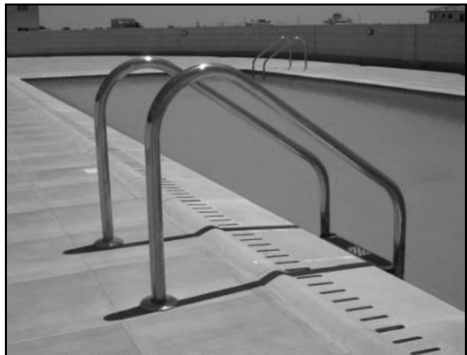
FIGURE 322.3.2(1) LADDER AS VIEWED ABOVE THE WATERLINE
