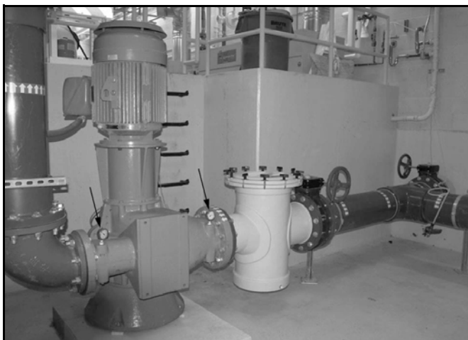
FIGURE 311.6 LOCATION OF PRESSURE GAUGES
