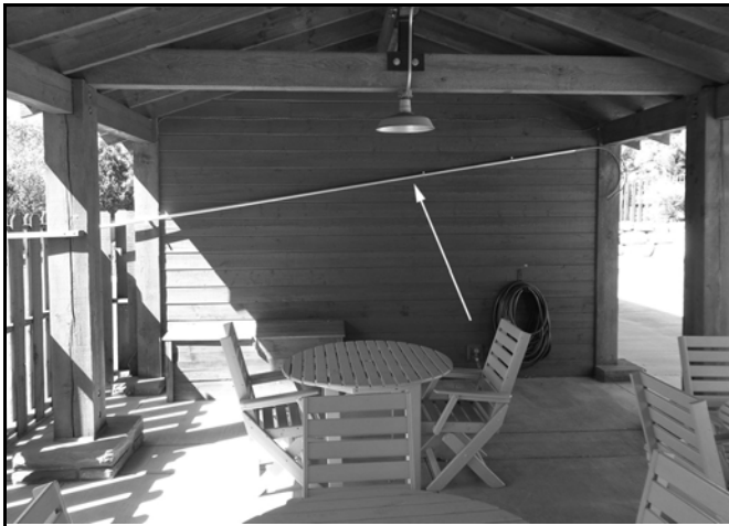
FIGURE 409.4.1 BODY HOOK HANGING ON POOL BUILDING WALL
