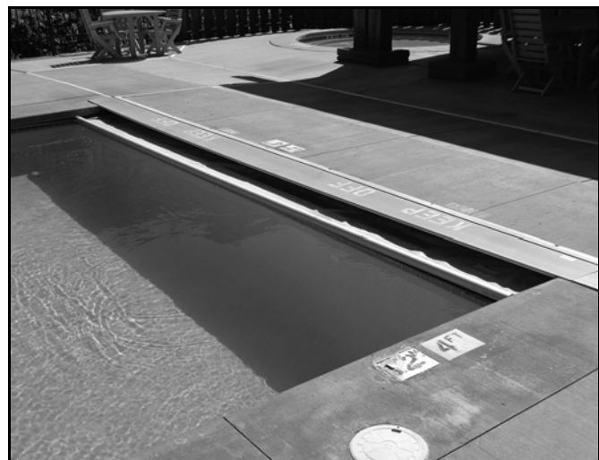
FIGURE 305.1(2) INTEGRAL-TYPE POWERED SAFETY COVER FOR PUBLIC POOL
