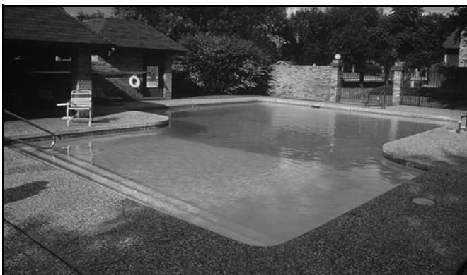
FIGURE 101.2(1) TYPICAL INGROUND POOL (Photo courtesy of Hamilton & Associates Architecture, Engineering, Technical Services)
