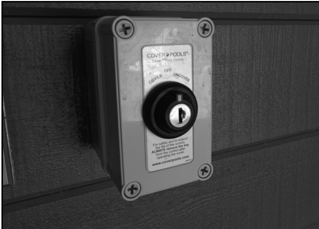
FIGURE 305.1(3) KEY SWITCH FOR POWERED POOL COVER OPERATION
