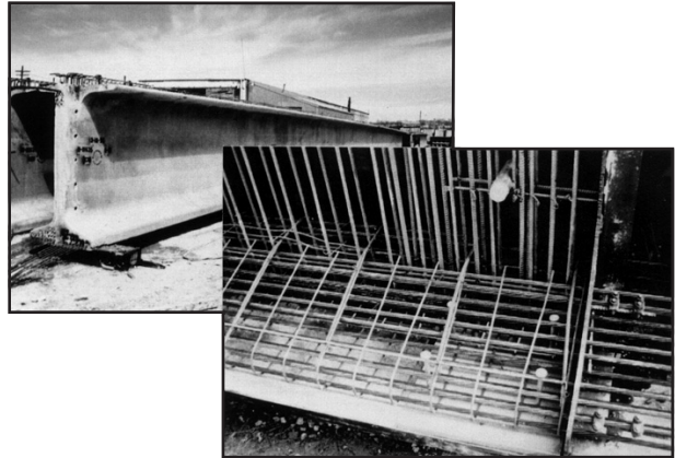
Bridge "I" girders have WWR shear reinforcement the full length.
