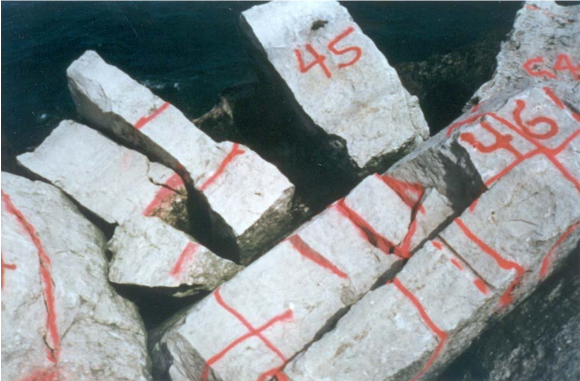
Figure V-2-13. Cracked stone - - Cleveland East breakwater, Ohio, 1990. Note continuing degradation compared to 1989 (stone is dolomitic limestone)
