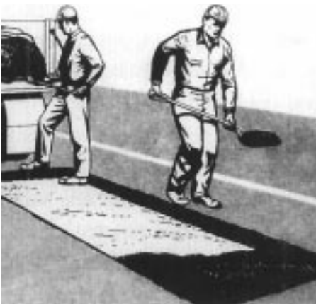
Backfilling Holes with Plant Mix
