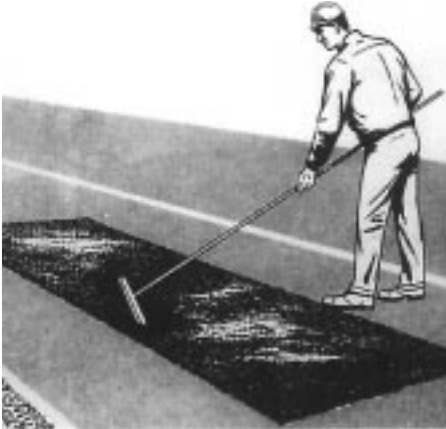
Spreading the Mix
