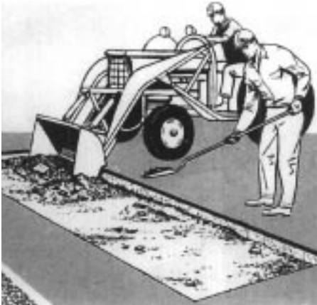
Removing Surface & Base
