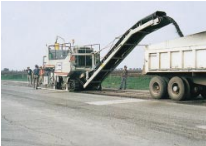
Removal by Cold Milling
