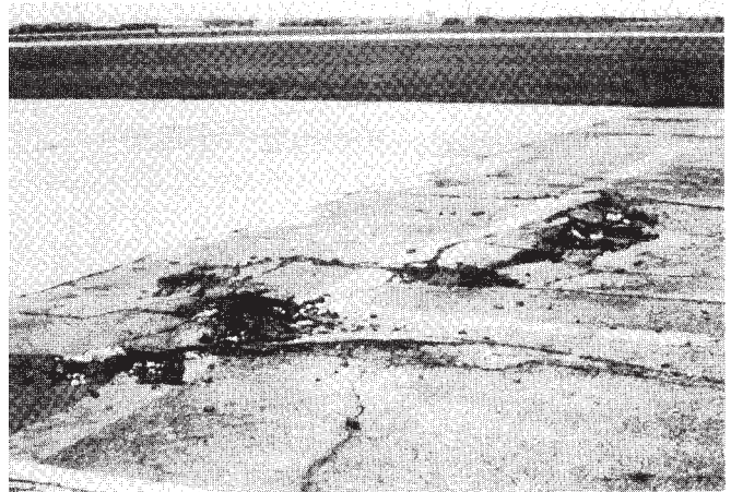
FIG. X1.72 High-Severity Shoving
