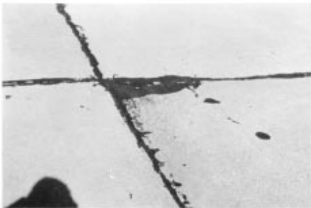
FIG. X2.19 Low-Severity "D" Cracking Approaching Medium Severity
