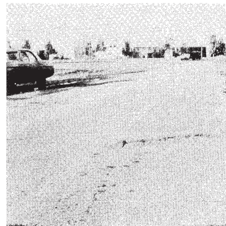
FIG. X1.77 High-Severity Swell
