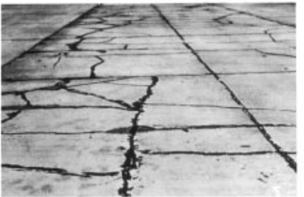
FIG. X2.58 Shattered Slab
