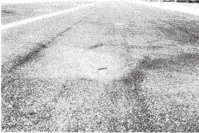
FIG. X1.26 Medium-Severity Depression
