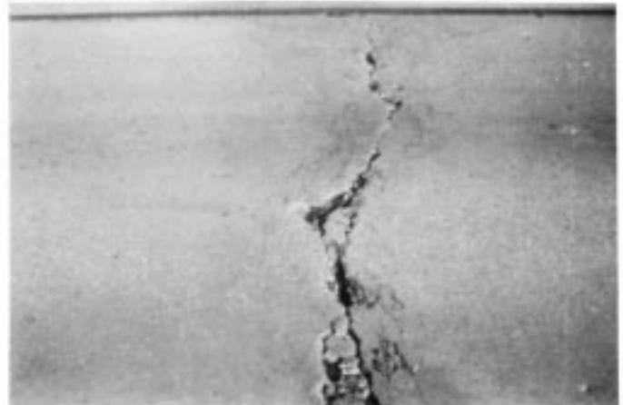
FIG. X2.15 High-Severity Crack
