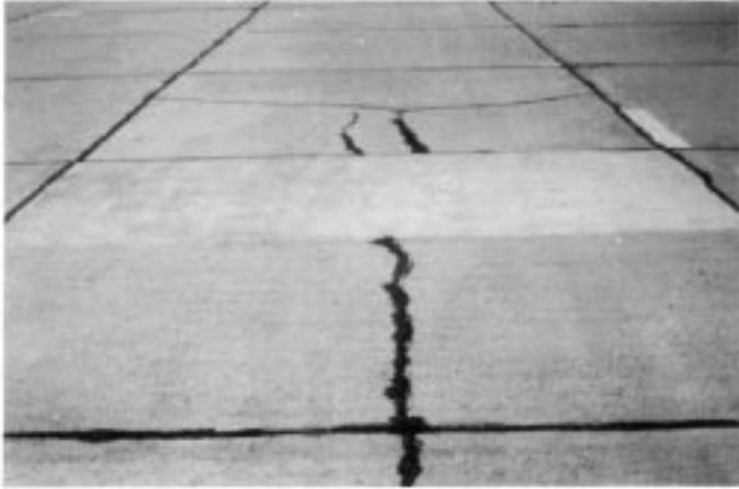
FIG. X2.34 Low-Severity Patch
