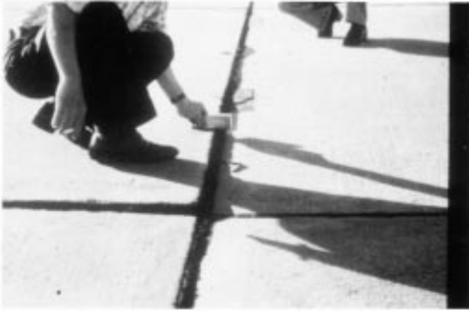
FIG. X2.53 High-Severity Settlement
