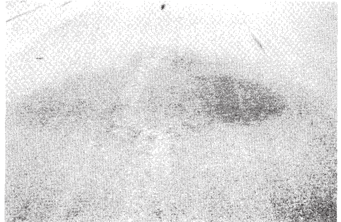
FIG. X1.24 Low-Severity Depression
