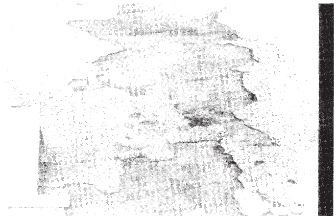
FIG. X1.59 High-Severity Raveling/Weathering
