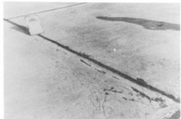
FIG. X2.22 High-Severity "D" Cracking
