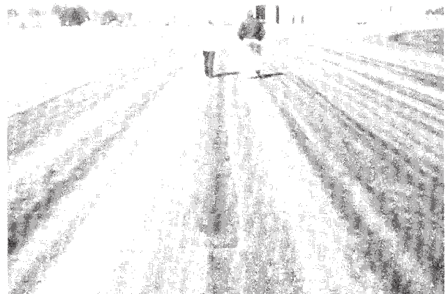
FIG. X1.48 Low-Severity Patch
