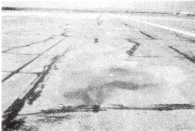
FIG. X1.27 High-Severity Depression (2 in. (50 mm))
