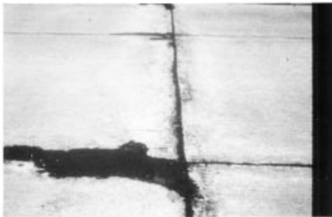
FIG. X2.45 Medium-Severity Scaling
