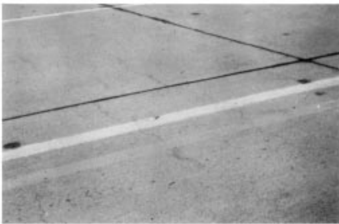
FIG. X2.60 Shrinkage Cracks
