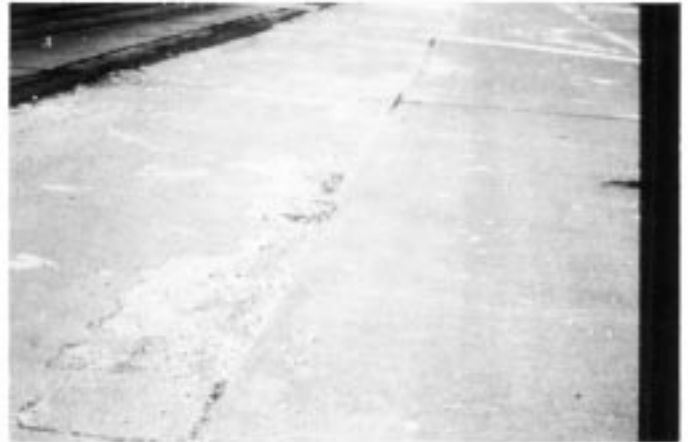
FIG. X2.46 High-Severity Scaling
