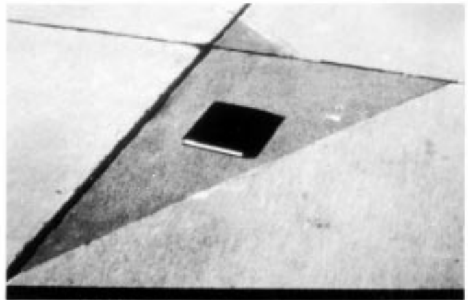
FIG. X2.33 Low-Severity Patch
