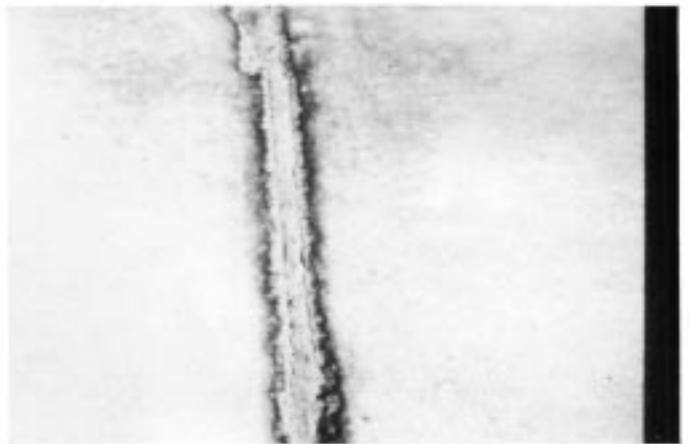
FIG. X2.41 Pumping (Close-Up of Fine Materials Collecting in the Joint)
