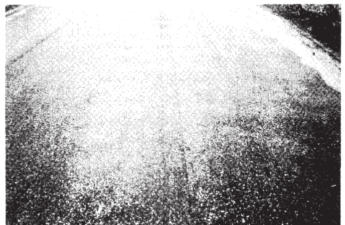
FIG. X1.21 Low-Severity Corrugation in the Foreground, Changing to Medium and High in the Background
