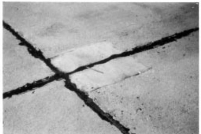
FIG. X2.28 Low-Severity Small Patch
