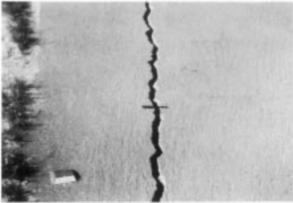
FIG. X2.17 High-Severity Crack
