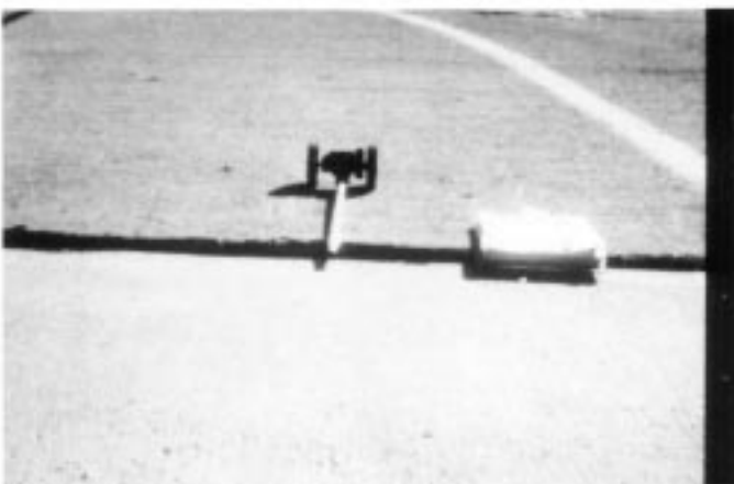
FIG. X2.52 High-Severity Settlement on Taxiway/Runway (3/4 in. (18 mm))
