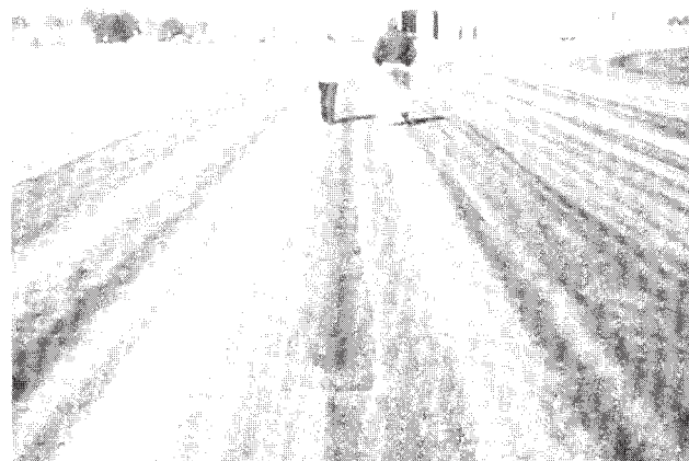
FIG. X1.48 Low-Severity Patch
