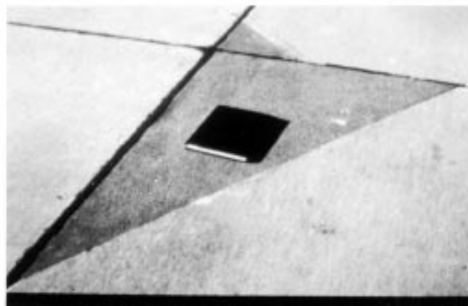
FIG. X2.33 Low-Severity Patch
