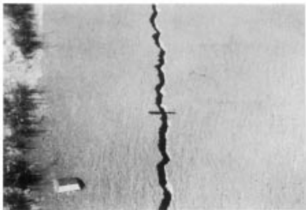
FIG. X2.17 High-Severity Crack
