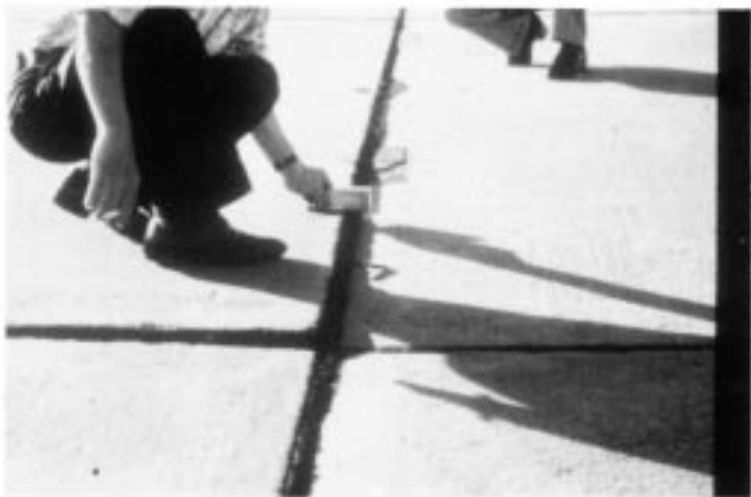
FIG. X2.53 High-Severity Settlement
