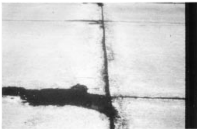
FIG. X2.45 Medium-Severity Scaling
