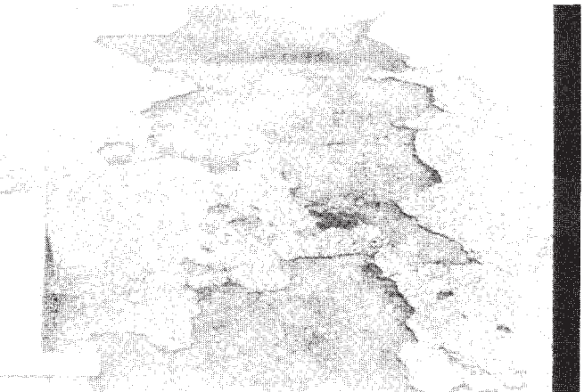
FIG. X1.59 High-Severity Raveling/Weathering
