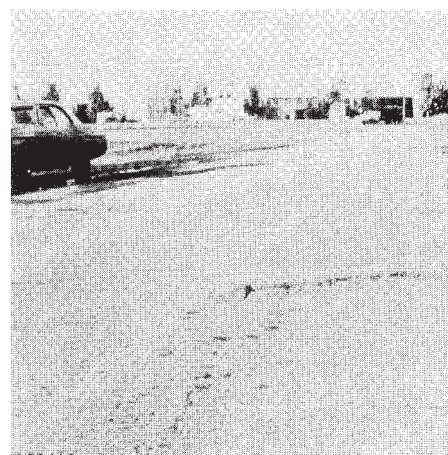
FIG. X1.77 High-Severity Swell
