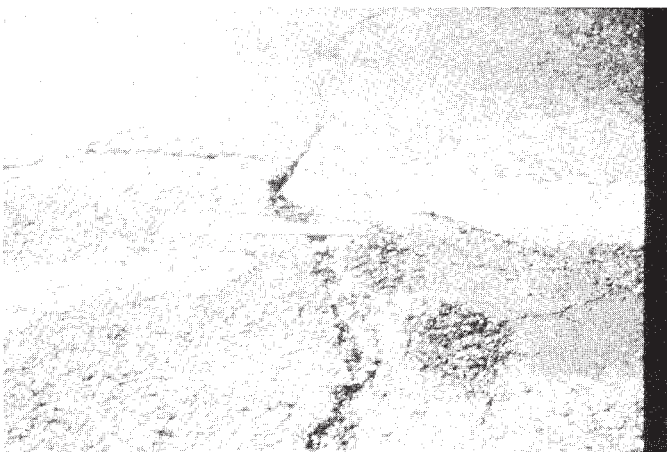
FIG. X1.42 High-Severity Longitudinal Crack
