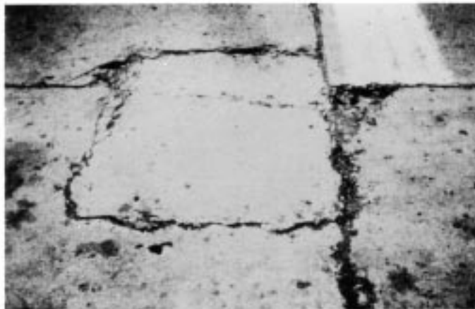
FIG. X2.37 High-Severity Patch
