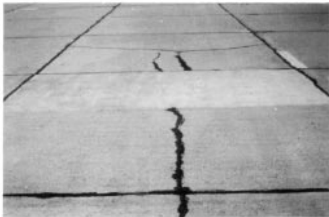
FIG. X2.34 Low-Severity Patch
