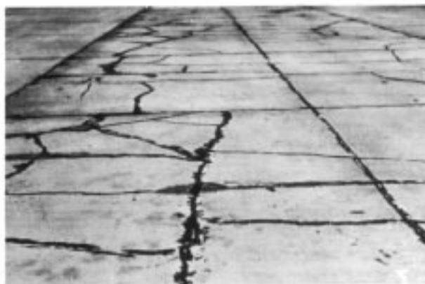
FIG. X2.58 Shattered Slab
