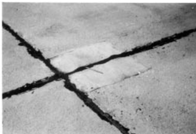
FIG. X2.28 Low-Severity Small Patch
