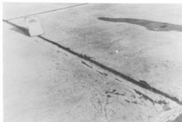
FIG. X2.22 High-Severity "D" Cracking
