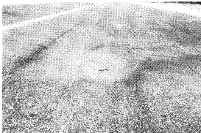
FIG. X1.26 Medium-Severity Depression
