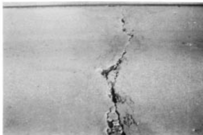
FIG. X2.15 High-Severity Crack
