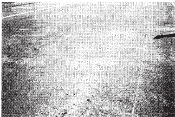
FIG. X1.22 Medium-Severity Corrugation
