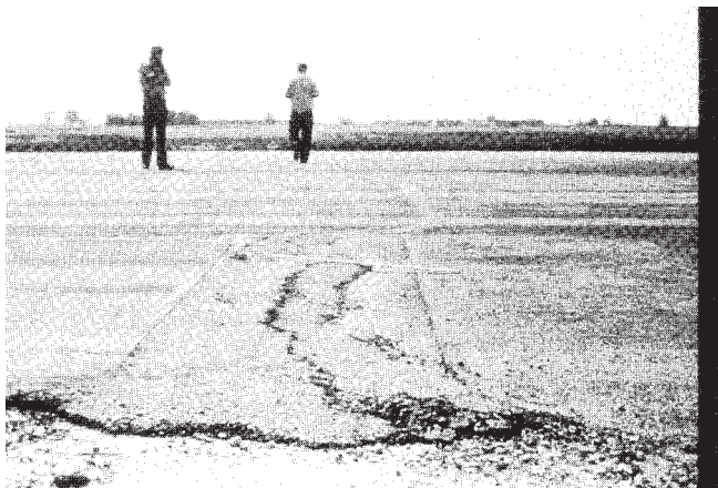
FIG. X1.52 High-Severity Patch
