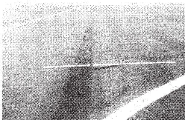
FIG. X1.70 High-Severity Rutting
