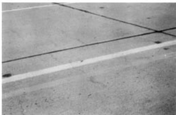
FIG. X2.60 Shrinkage Cracks
