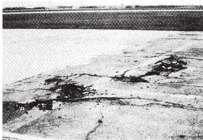
FIG. X1.72 High-Severity Shoving
