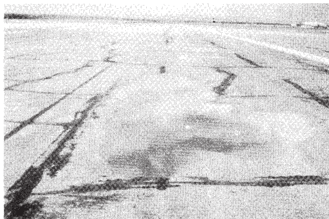
FIG. X1.27 High-Severity Depression (2 in. (50 mm))
