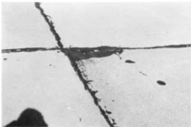
FIG. X2.19 Low-Severity "D" Cracking Approaching Medium Severity
