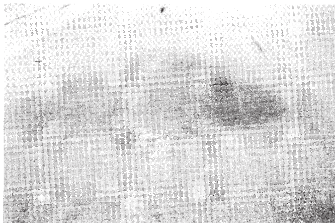
FIG. X1.24 Low-Severity Depression
