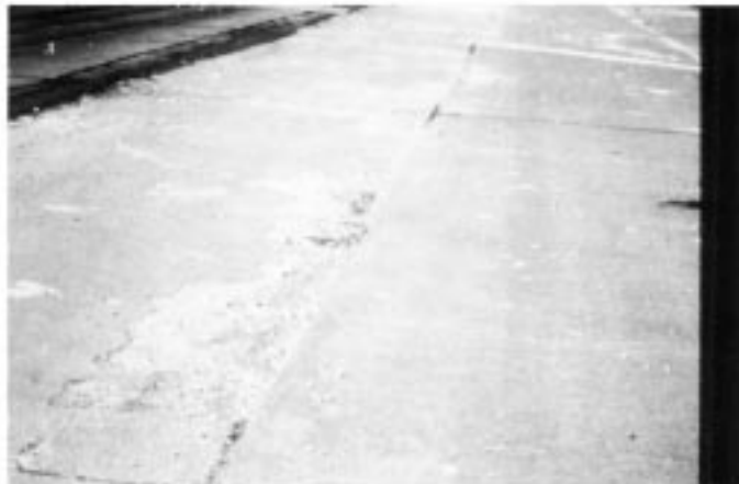
FIG. X2.46 High-Severity Scaling
