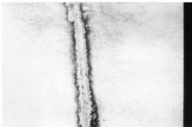
FIG. X2.41 Pumping (Close-Up of Fine Materials Collecting in the Joint)
