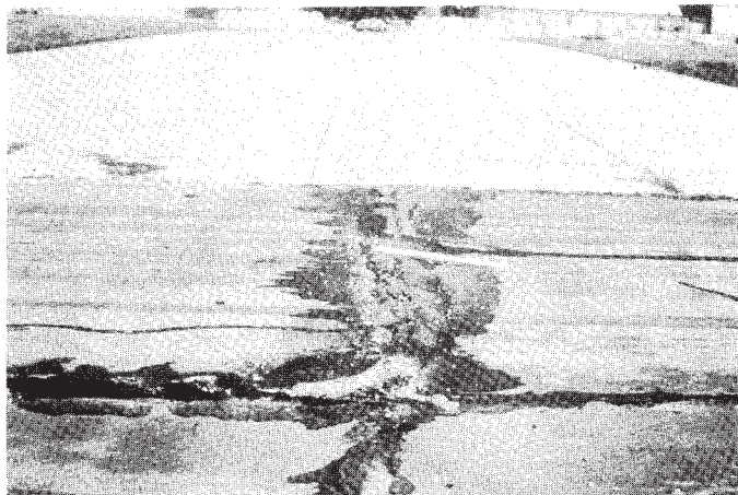
FIG. X1.78 High-Severity Swell
