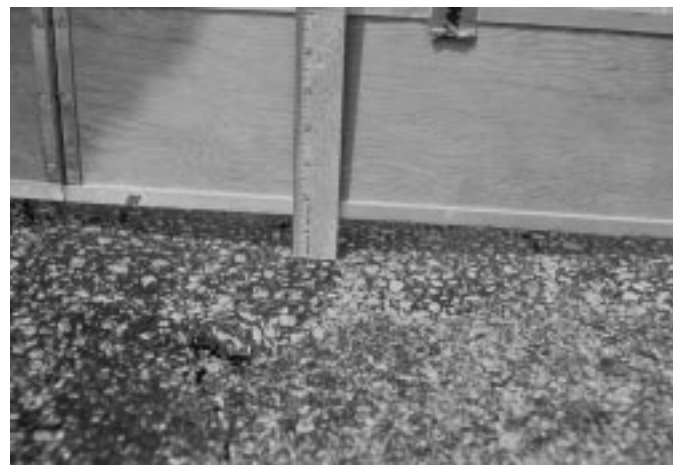
FIG. X1.43 High-Severity Rutting
