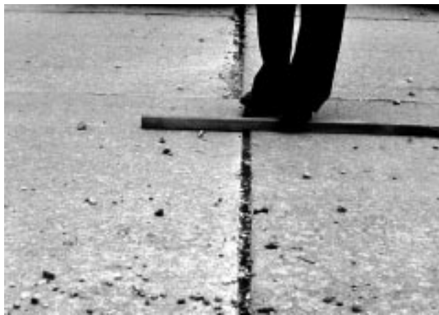
FIG. X2.13 Low-Severity Faulting
