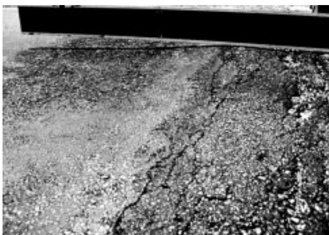
FIG. X1.12 High-Severity Bumps and Sags
