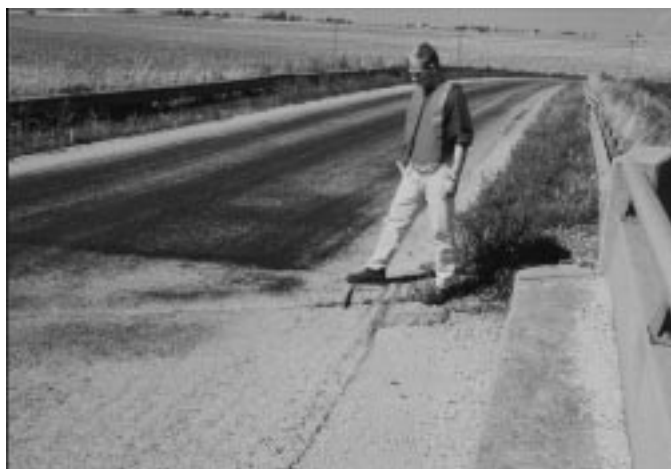
FIG. X1.44 Low-Severity Shoving
