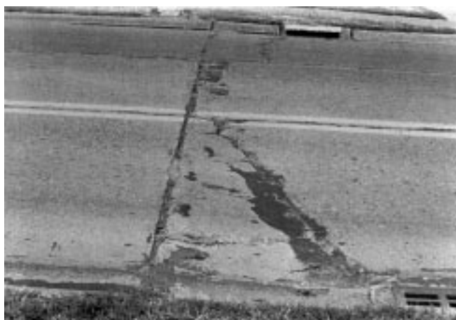
FIG. X2.36 Medium-Severity Punchout
