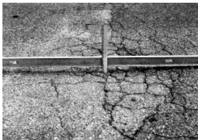
FIG. X1.18 High-Severity Depression
