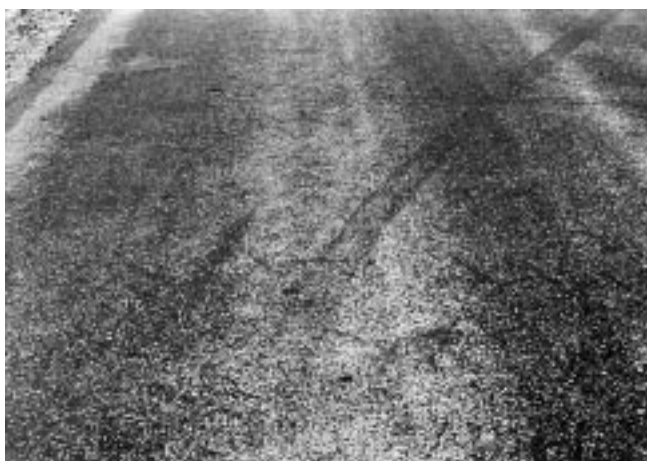
FIG. X1.4 Low-Severity Bleeding
