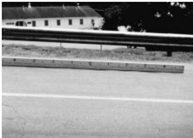
FIG. X1.13 Low-Severity Corrugation
