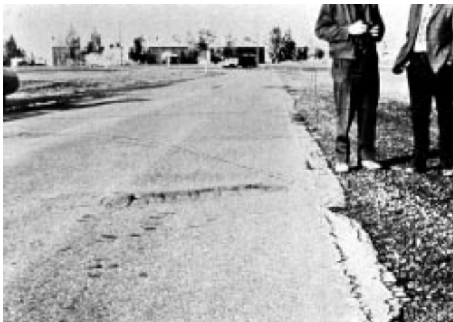
FIG. X1.11 Medium-Severity Bumps and Sags
