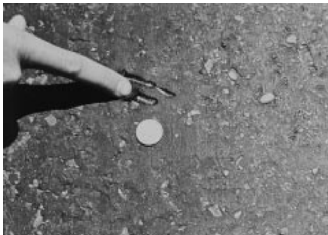
FIG. X1.5 Medium-Severity Bleeding
