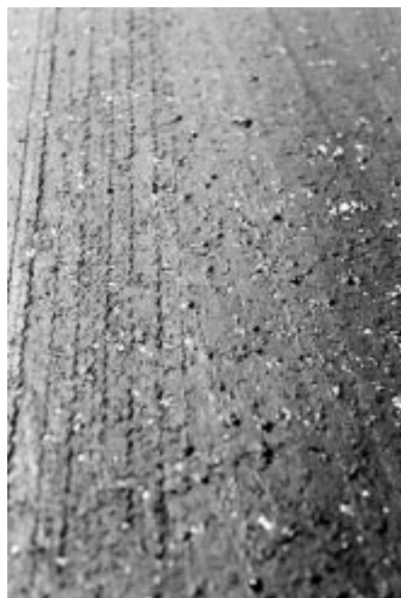
FIG. X1.6 High-Severity Bleeding
