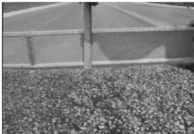
FIG. X1.42 Medium-Severity Rutting
