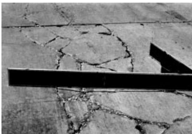
FIG. X2.37 High-Severity Punchout
