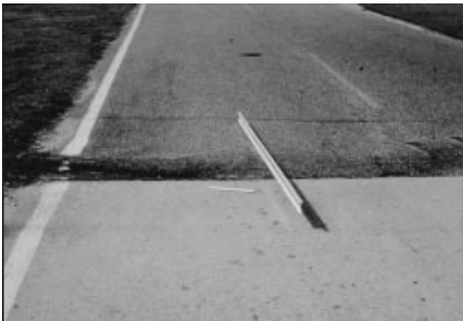
FIG. X1.46 High-Severity Shoving
