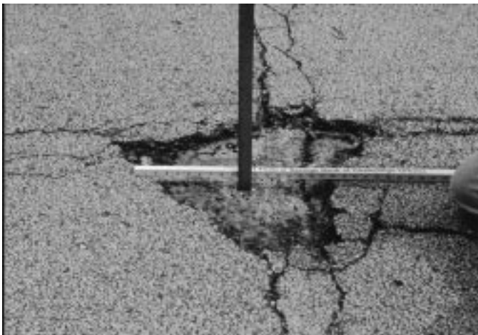
FIG. X1.36 Medium-Severity Pothole
