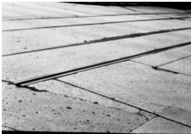
FIG. X2.38 Low-Severity Railroad Crossing
