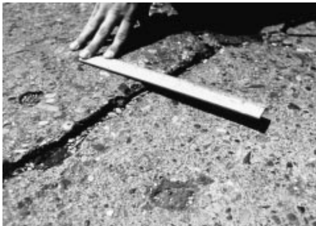
FIG. X2.14 Medium-Severity Faulting
