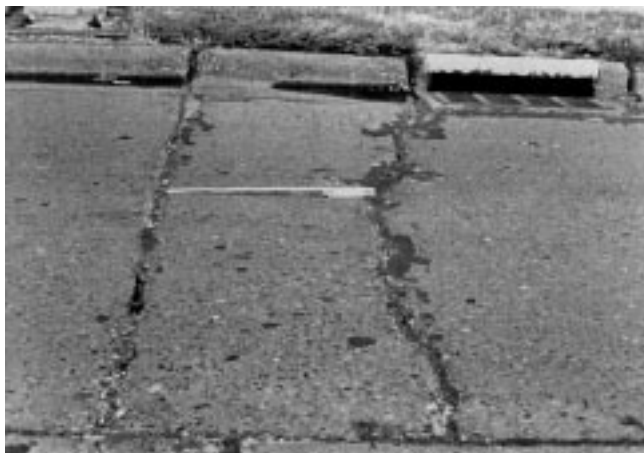
FIG. X2.35 Low-Severity Punchout
