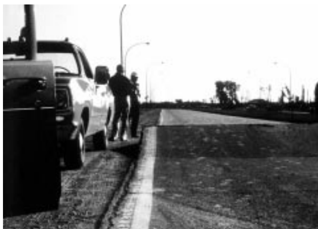
FIG. X2.3 High-Severity Blowup/Buckling
