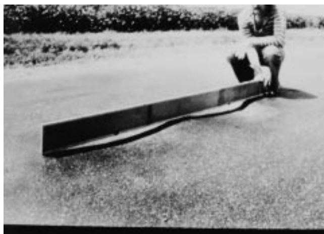
FIG. X1.15 High-Severity Corrugation
