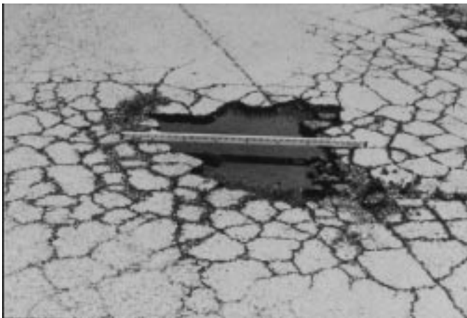
FIG. X1.37 High-Severity Pothole
