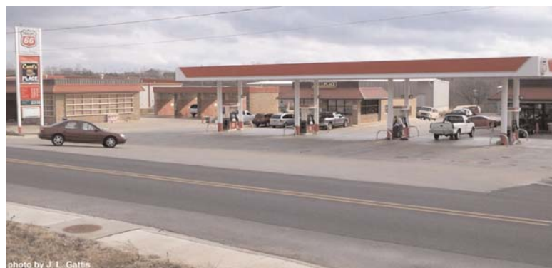
Exhibit 5-17. Undesirable wide-open driveway.
