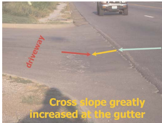
Exhibit 5-73. Increased gutter cross slope.
