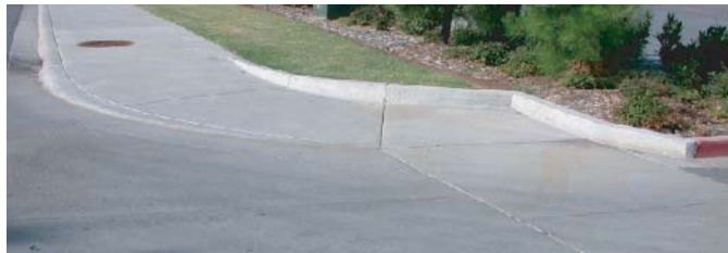
Exhibit 5-10. Unacceptable vertical curb where sidewalk crosses driveway.
