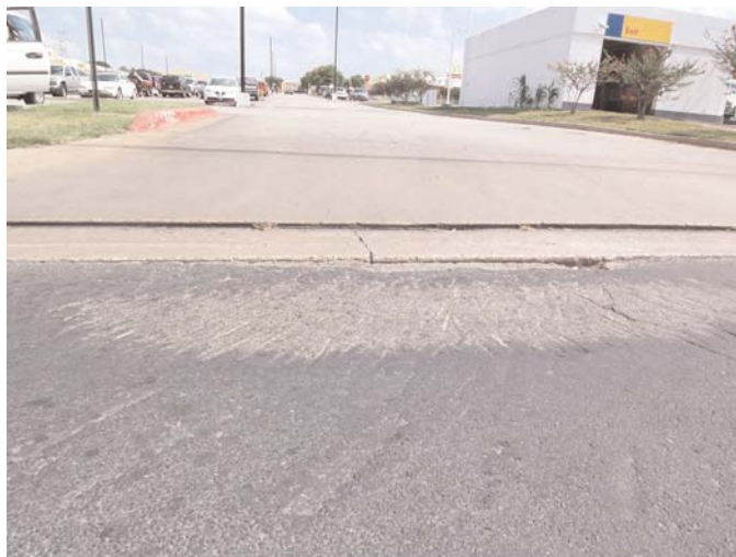
Exhibit 5-66. Driveway with multiple scrapes from underside dragging.
