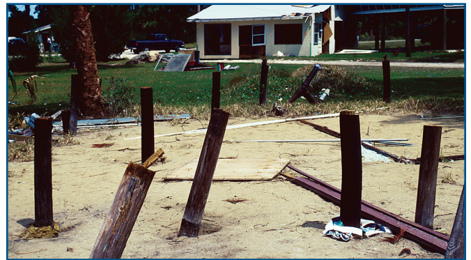
Insufficient pile embedment and failure of connections at tops of piles allowed elevated building to be floated off its foundation.
