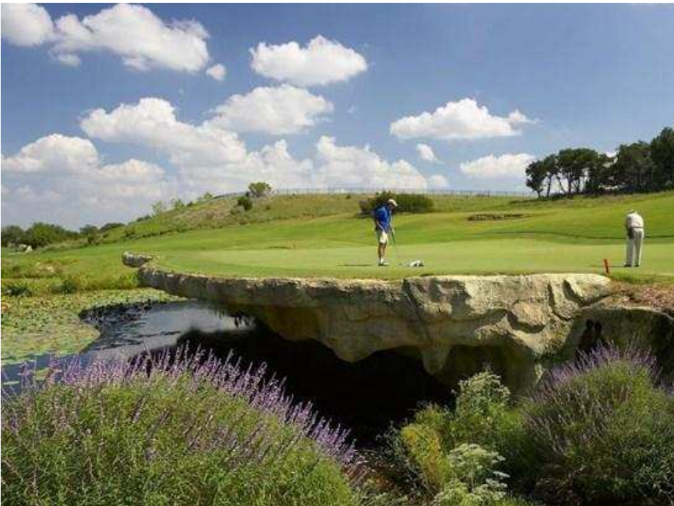
This cantilevered golf course green is actually a post-tensioned concrete slab. Suncoast Post-Tension
