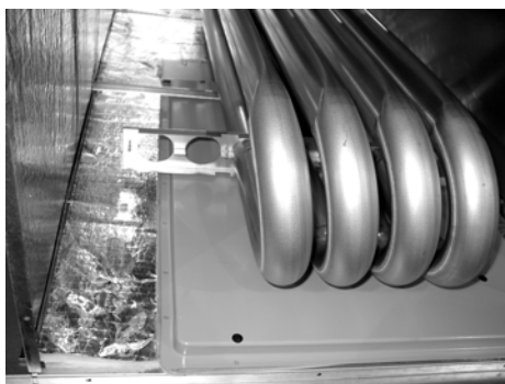
FIGURE 15 - DISCHARGE PANEL IN PLACE
