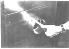
Figure H-Collar in duct min. 2"
