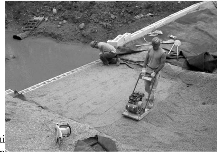
Figure 8.34 Construction of a geotextile-reinforced retaining wall (Courtesy of Jonathan T. H. Wu, University of Colorado at Denver, Denver, Colorado)
