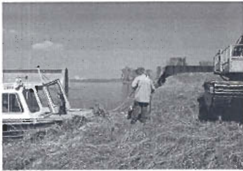
Levee Breach at Bienvenue Flood Gate
