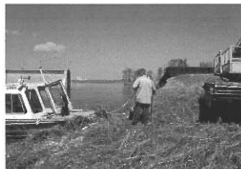
Levee Breach at Bienvenue Flood Gate
