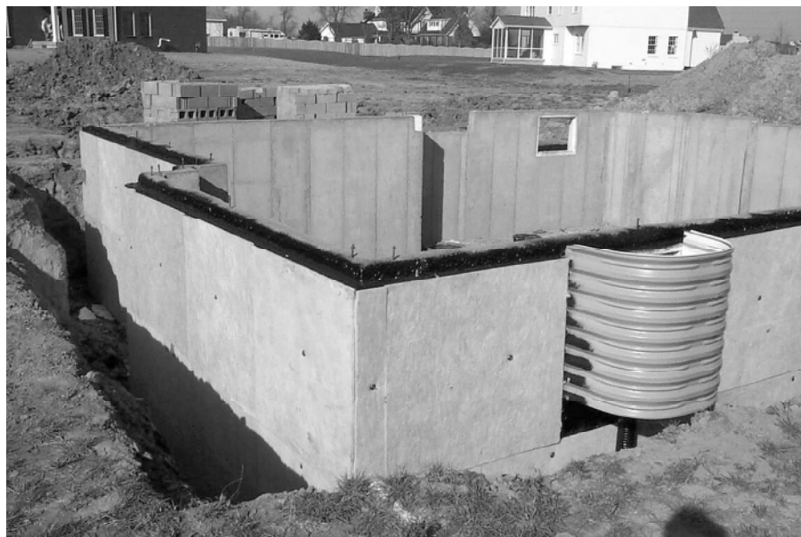
Figure N1102.2.8(2) WALK-OUT BASEMENT
