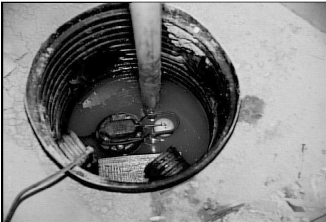
Figure R202(16) SUMP PUMP
