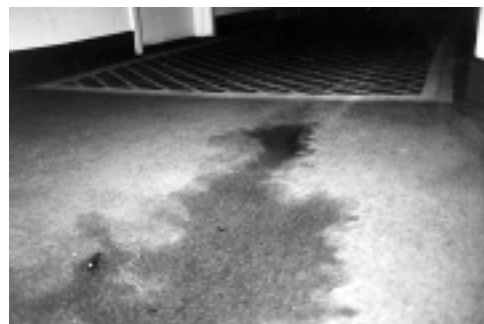
FIGURE 4.17.7.2(b) Irregularly shaped pattern on floor carpeting resulting from poured ignitable liquid. Burned match can be seen at lower left.
