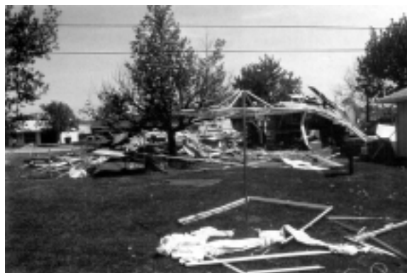
FIGURE 18.3.2 High-order damage shown by shattered and splintered remains of a four-bedroom house.
