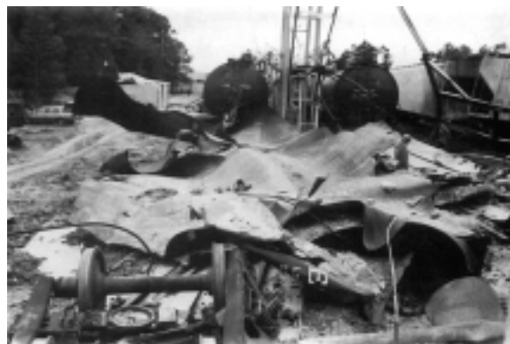
FIGURE 18.2.2(b) A railroad tank car of butadiene that suffered a BLEVE as a result of heating created by an internal chemical reaction.
