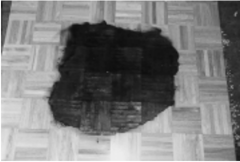
FIGURE 4.17.7.2(c) “Pool-shaped” burn pattern produced by a cardboard box burning on an oak parquet floor.
