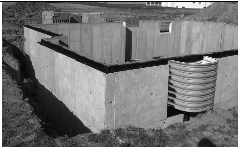
Figure R402.2.9(2) EXTERIOR BASEMENT INSULATION
