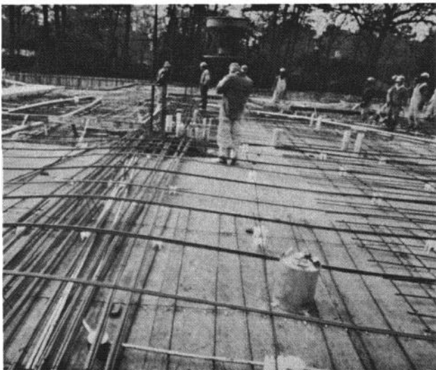
Fig. 6.11 — Flat plate banded tendon distribution.
