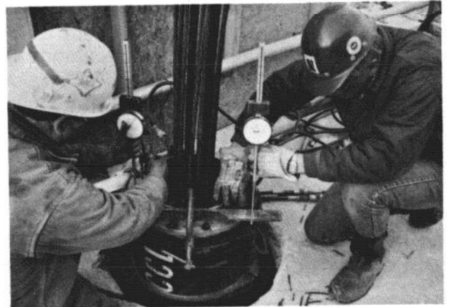
Stressing test Wanaque Dam, Wanaque, New Jersey
