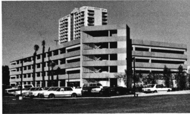
One Columbus Parking Garage, Phoenix, Arizona
