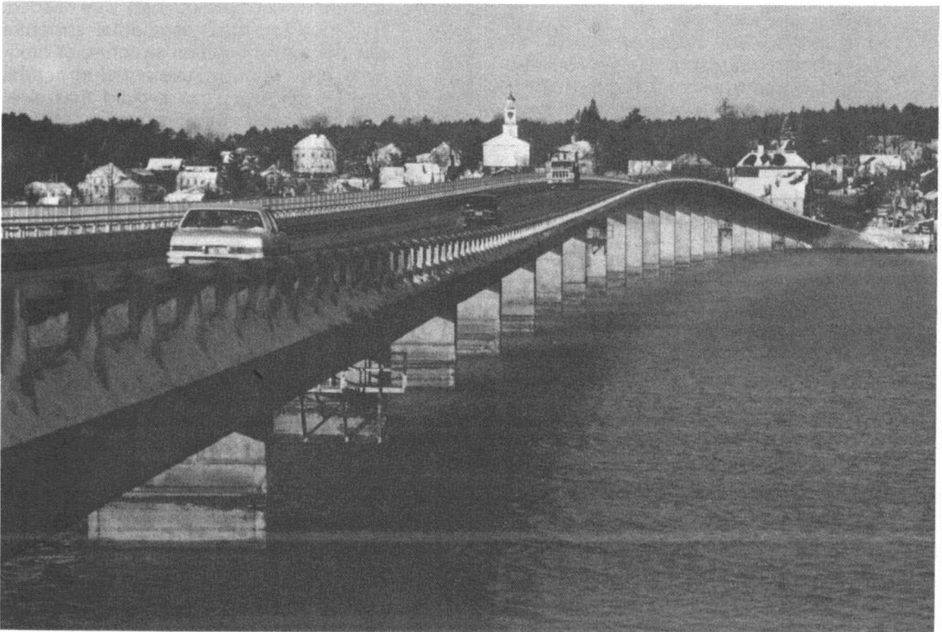
Fig. 1.52 The Wiscasset Bridge, Maine
