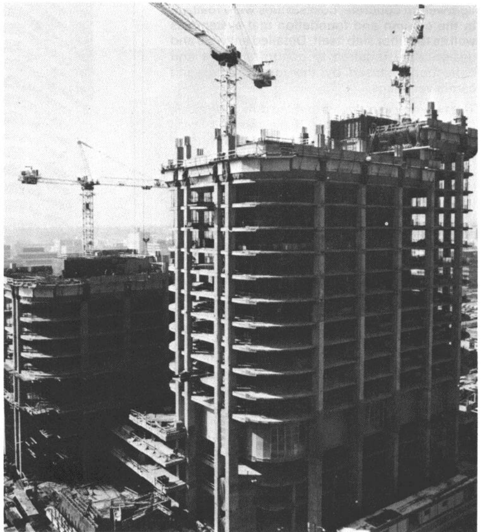
Fig. 1.11— Winter Construction of Western Canadian Place, Calgary, Alberta, Canada.
