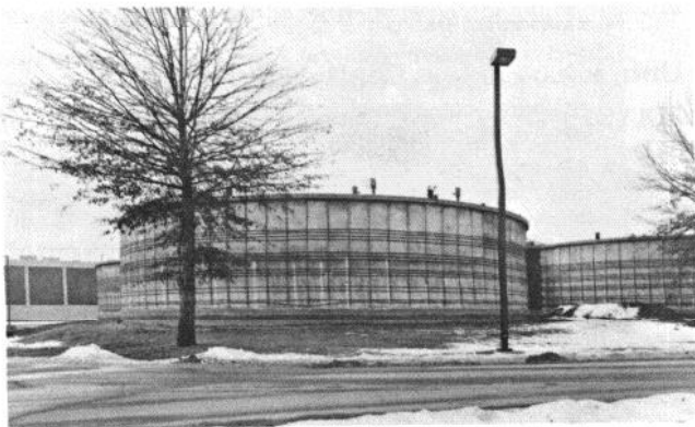
Hoops for sewage tank repair, Bergen County, NJ
