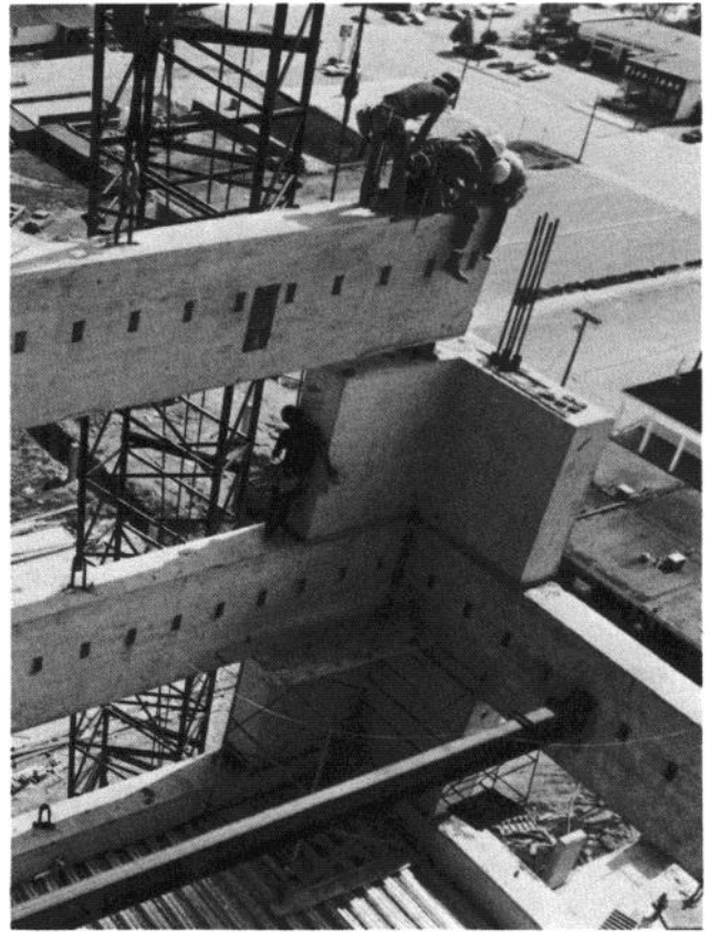
Fig. 1.24 — Assembly of Exterior Framing. Citizen's Bank Center, Richardson, Texas.
