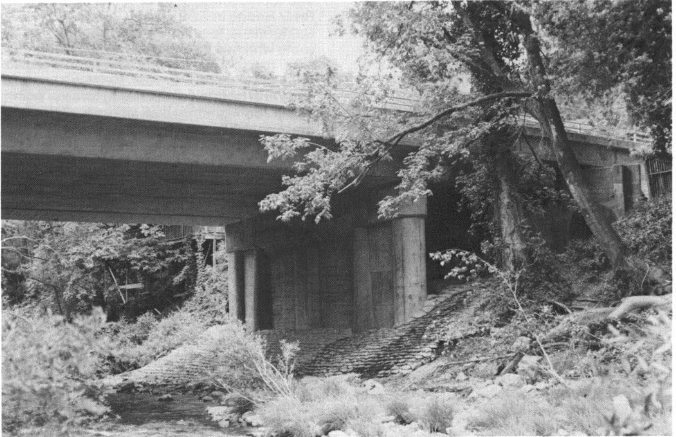
Fig 1 63 — San Lorenzo River Bridge| Santa Cruz County, California
