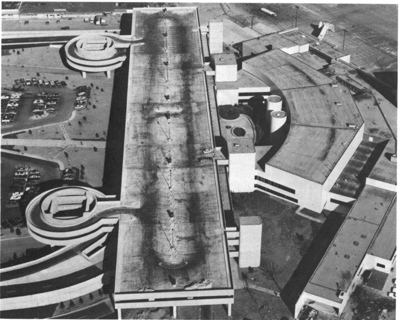
Fig 1.20 — Port Columbus International Airport Parking Structure, Columbus, Ohio
