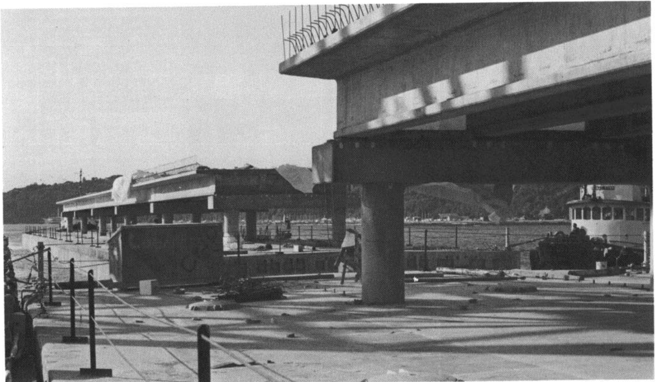
Fig. 1.74 Pontoon Placement. Hood Canal Floating Bridge, Washington
