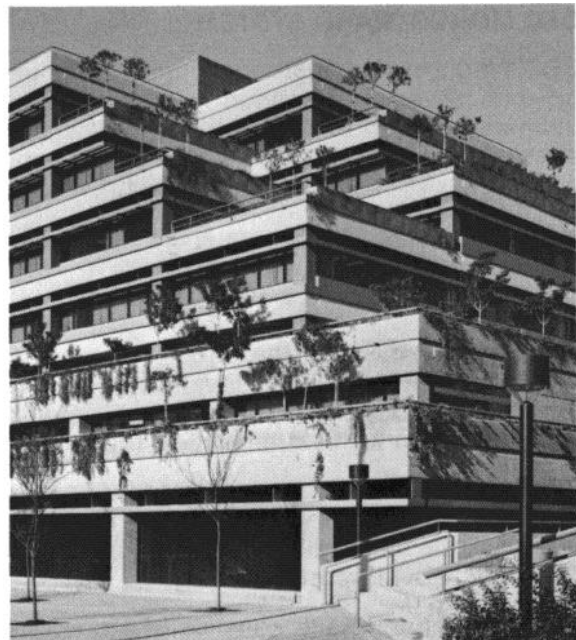
Walnut Creek Center No. 1, a CEC project located in Walnut Creek, California. Low-rise office and underground-parking structure using a two-way grid with post-tensioned ductile frame.
