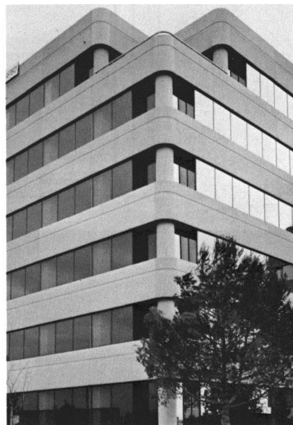
Airport Plaza, a CEC project in Concord, California. A medium-rise office building using post-tensioned beams precast and erected on site. Post-tensioning was employed in order to control long-span deflection.
