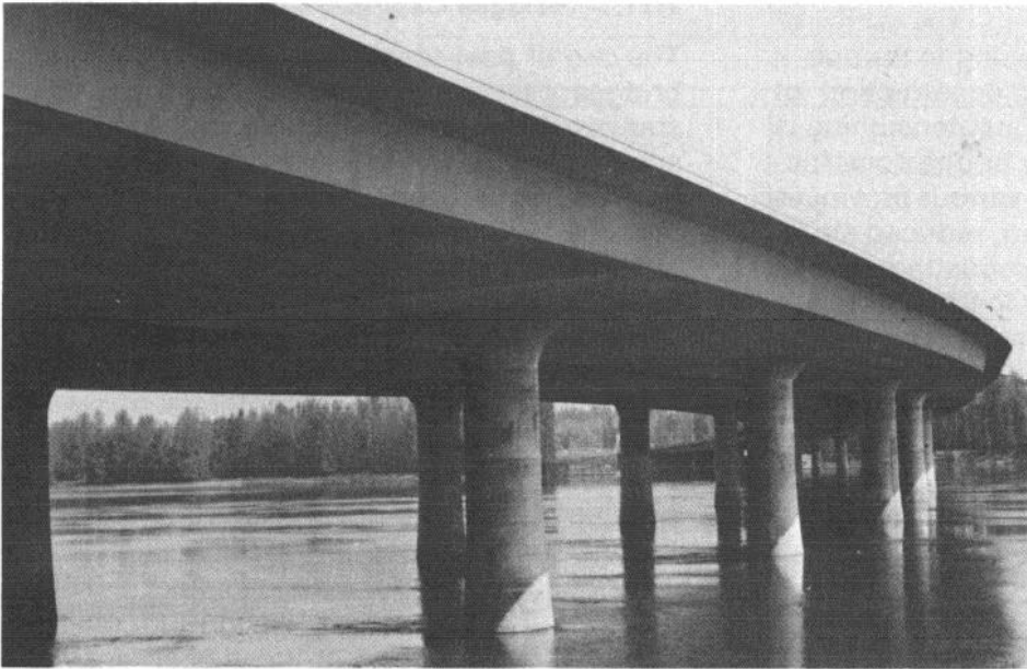
Fig 1.44 — Columbia River South Channel Bridge I-205 at Portland, Oregon Seventeen spans ranging from 120ft to 200 ft Overall length of 3,114 ft.
