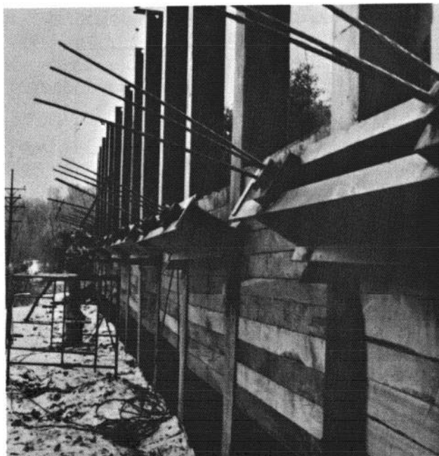
Anchor wall Consolidation Coal Arkwright Mine
