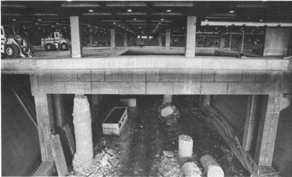
Fig. 1.71 Excavation Under Transfer Girders Supported on Original Caissons.
