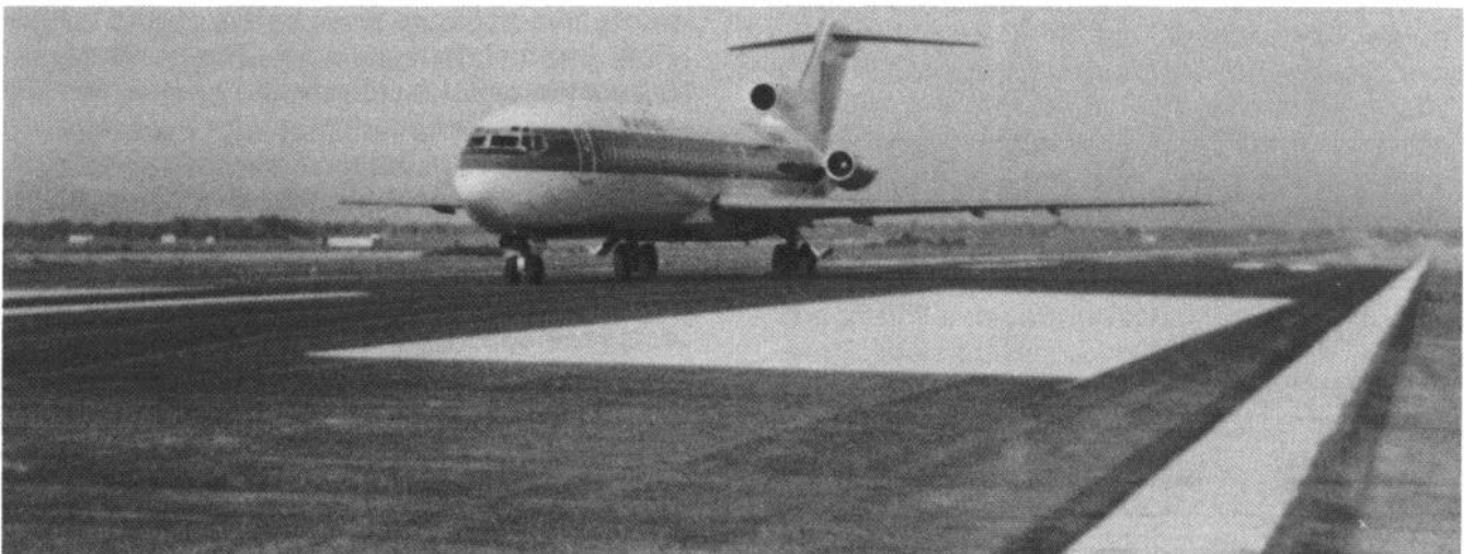
Fig. 1.42 — Post-Tensioned Runway, O'Hare International Airport, Chicago, Illinois
