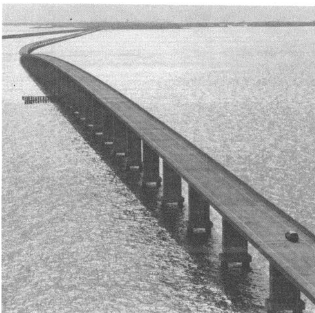
Fig 1.50 — Seven Mile Bridge Florida Keys
