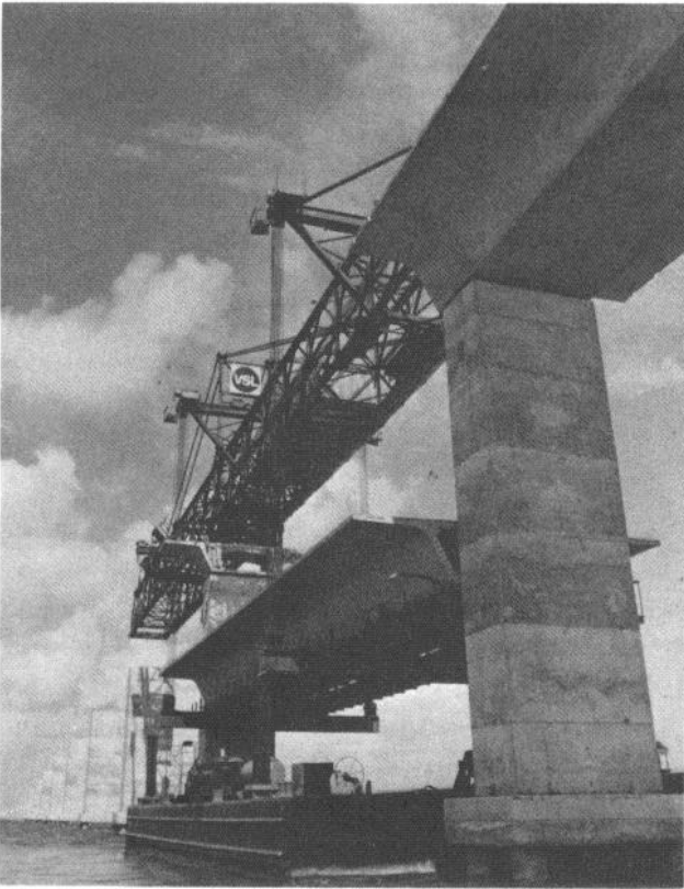
Fig. 1.51 Overhead Gantry, Seven Mile Bridge, Florida, Keys
