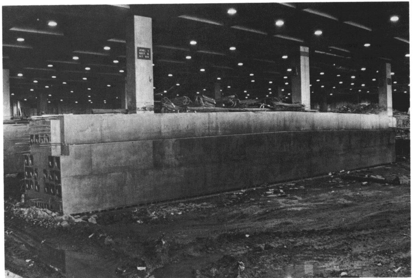
Fig. 1.70 — Completed Transfer Girder| O'Hare international Airport| Chicago.
