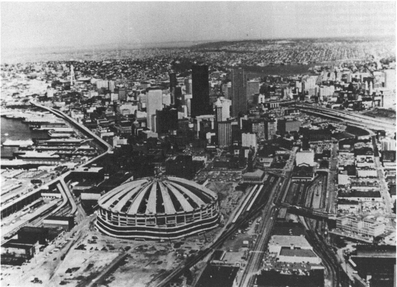
Seattle's Kingdome boasts the largest concrete dome in the world. This unique structure has a 660 foot clear span. The
