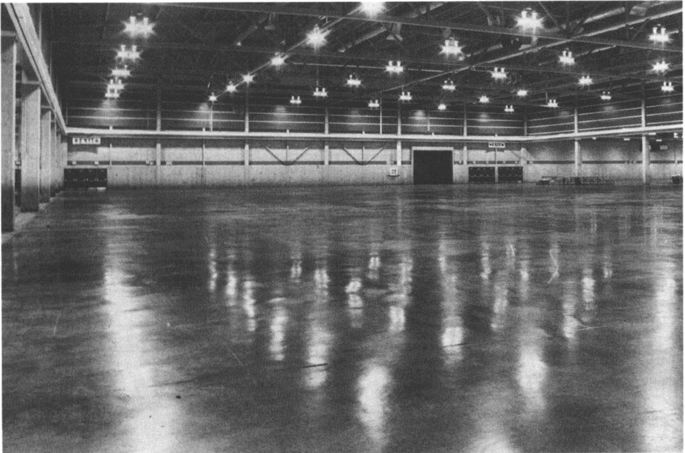
Fig. 1.40 — Post-Tensioned Floor Slab, Roundup Centre, Calgary, Alberta, Canada.
