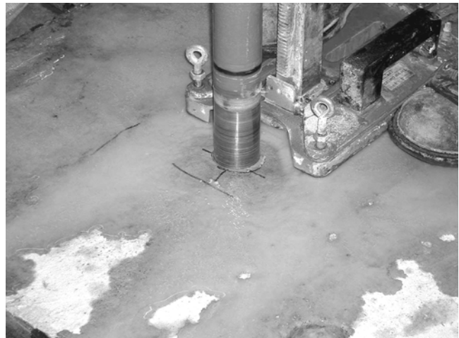
Fig. 10—Coring hole for anode.
