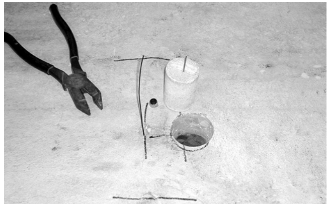
Fig. 11—Secondary hole with reinforcing steel connection.
