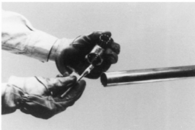
FIG. 11 Fluxing: Fitting
