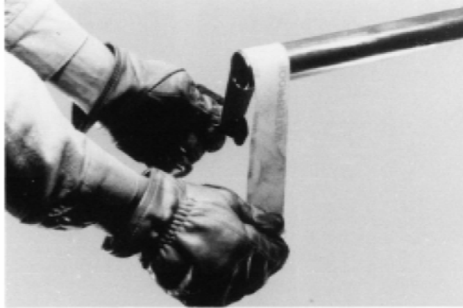
FIG. 6 Cleaning: Sand Cloth
