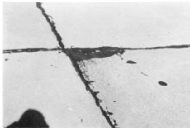
FIG. X2.19 Low-Severity "D" Cracking Approaching Medium Severity
