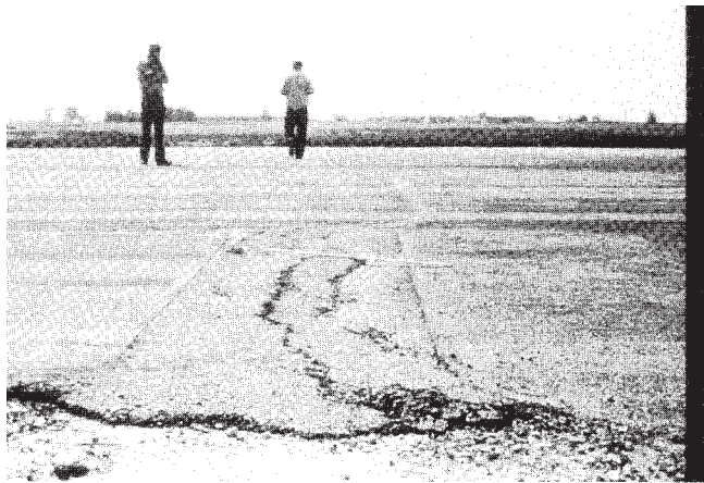
FIG. X1.52 High-Severity Patch
