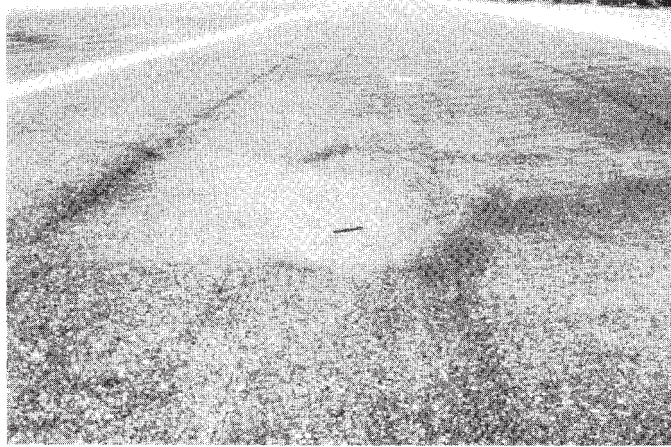
FIG. X1.26 Medium-Severity Depression
