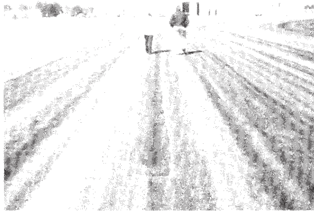
FIG. X1.48 Low-Severity Patch
