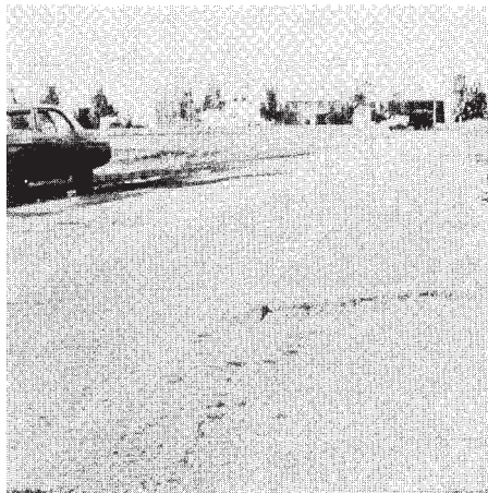
FIG. X1.77 High-Severity Swell
