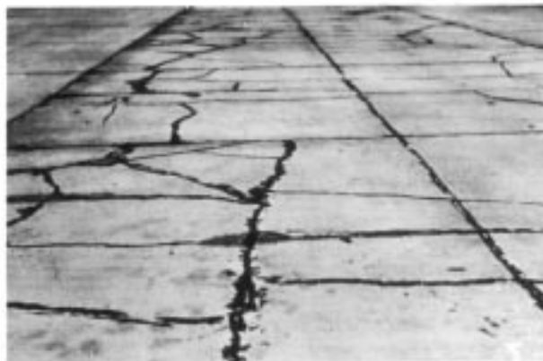
FIG. X2.58 Shattered Slab
