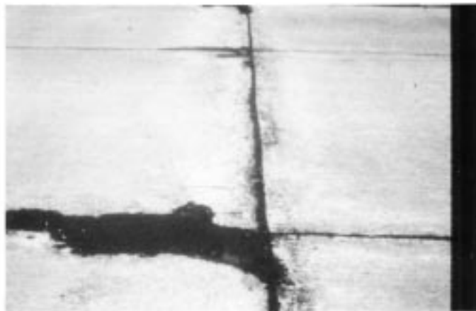
FIG. X2.45 Medium-Severity Scaling
