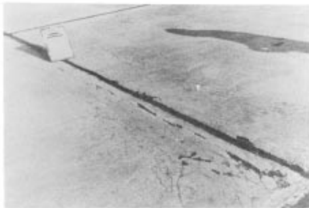
FIG. X2.22 High-Severity "D" Cracking
