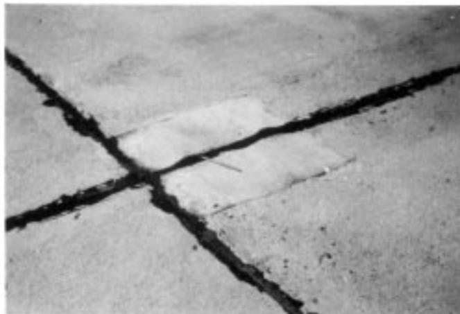
FIG. X2.28 Low-Severity Small Patch
