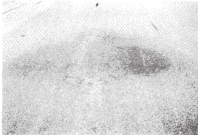
FIG. X1.24 Low-Severity Depression
