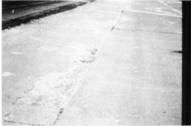
FIG. X2.46 High-Severity Scaling
