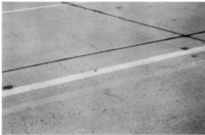
FIG. X2.60 Shrinkage Cracks
