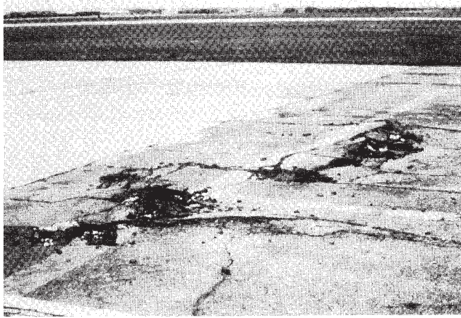
FIG. X1.72 High-Severity Shoving
