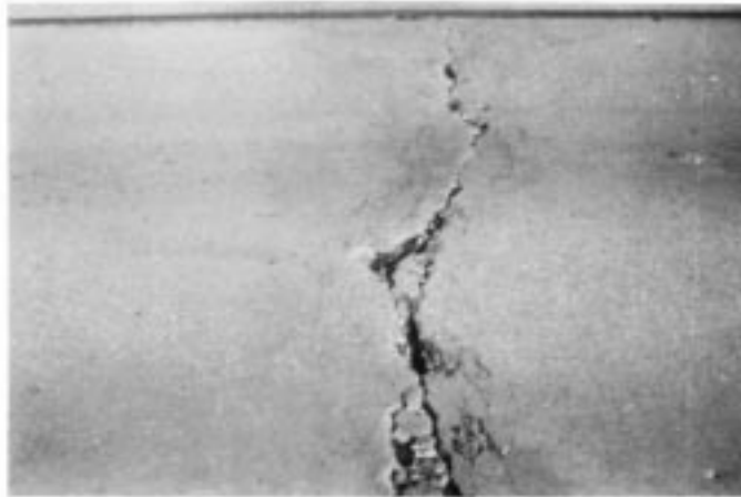
FIG. X2.15 High-Severity Crack
