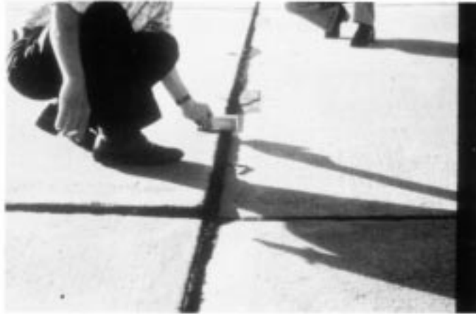
FIG. X2.53 High-Severity Settlement
