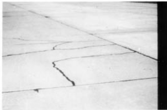
FIG. X2.55 Low-Severity Intersecting Cracks
