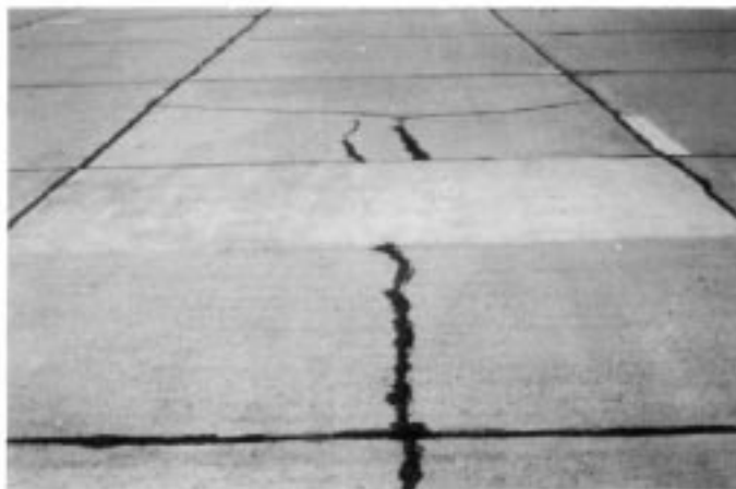
FIG. X2.34 Low-Severity Patch
