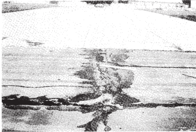
FIG. X1.78 High-Severity Swell
