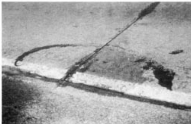
FIG. X2.39 Pumping (Note Fine Material on Surface That has Been Pumped Out Causing Corner Break)
