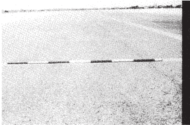
FIG. X1.66 Low-Severity Rutting
