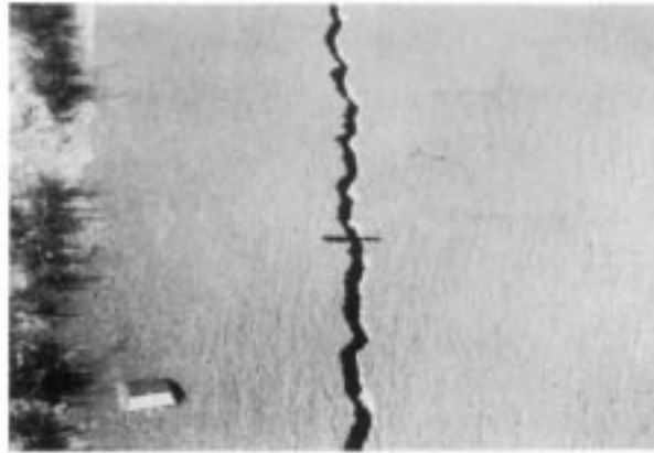
FIG. X2.17 High-Severity Crack
