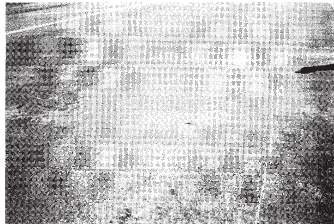
FIG. X1.22 Medium-Severity Corrugation
