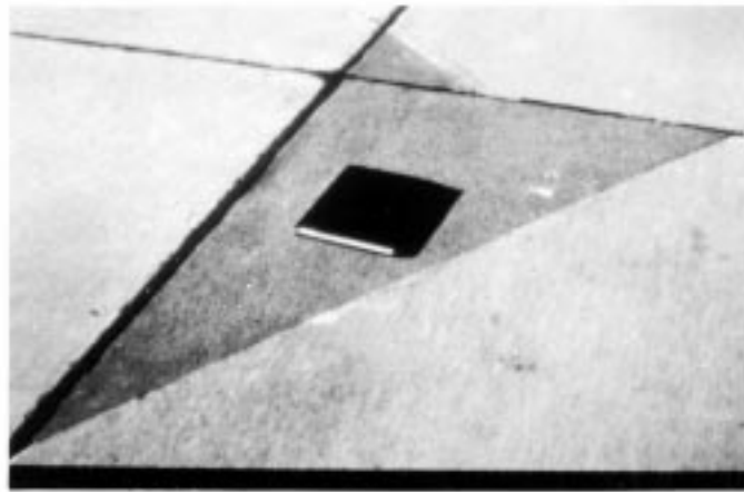
FIG. X2.33 Low-Severity Patch
