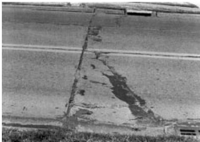
FIG. X2.36 Medium-Severity Punchout
