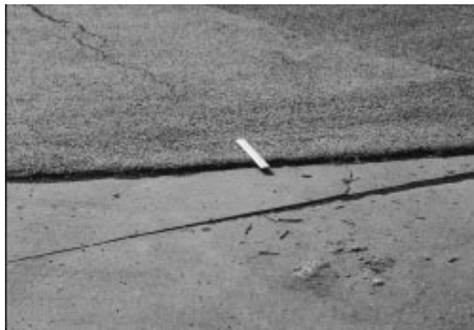
FIG. X1.45 Medium-Severity Shoving
