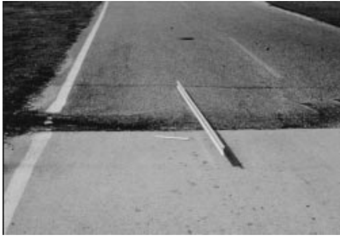
FIG. X1.46 High-Severity Shoving
