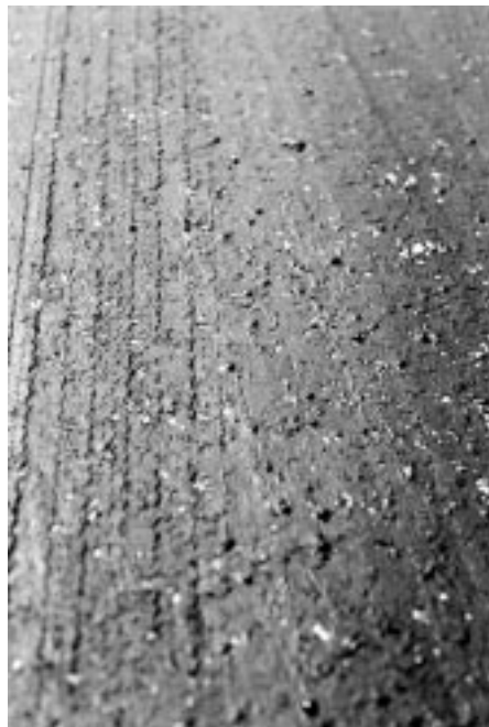
FIG. X1.6 High-Severity Bleeding
