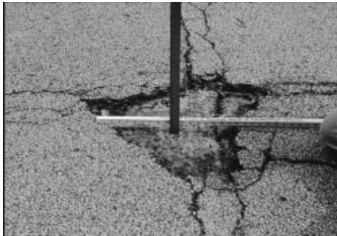
FIG. X1.36 Medium-Severity Pothole
