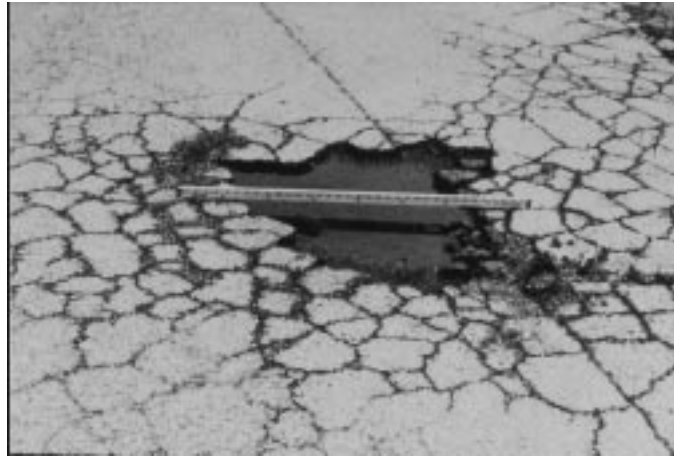
FIG. X1.37 High-Severity Pothole
