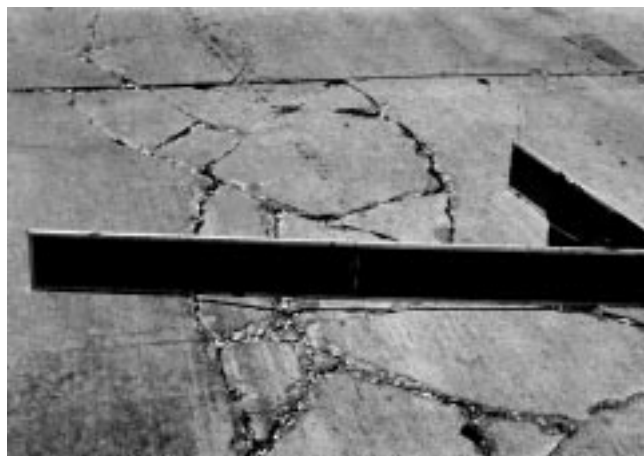
FIG. X2.37 High-Severity Punchout
