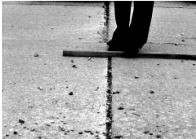
FIG. X2.13 Low-Severity Faulting
