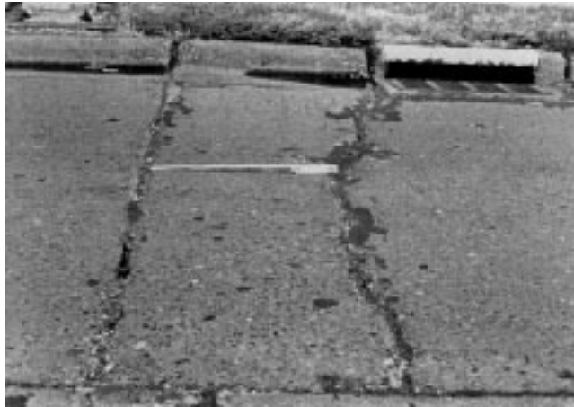
FIG. X2.35 Low-Severity Punchout
