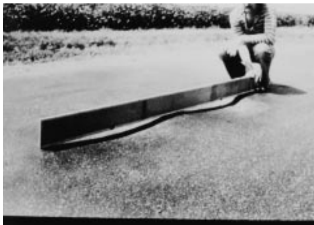
FIG. X1.15 High-Severity Corrugation
