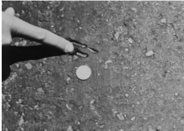
FIG. X1.5 Medium-Severity Bleeding
