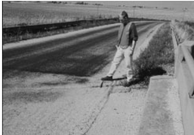
FIG. X1.44 Low-Severity Shoving
