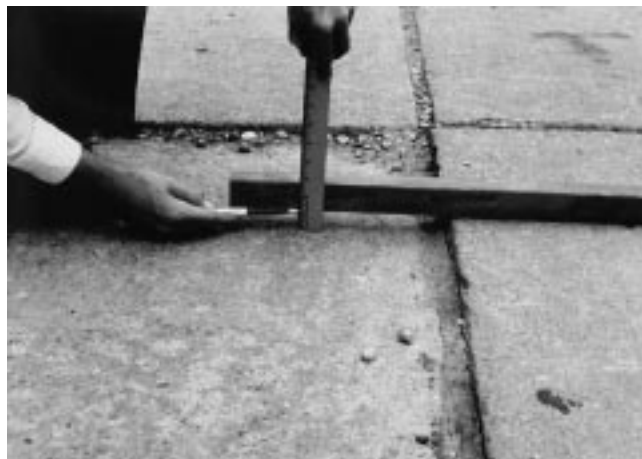
FIG. X2.15 High-Severity Faulting
