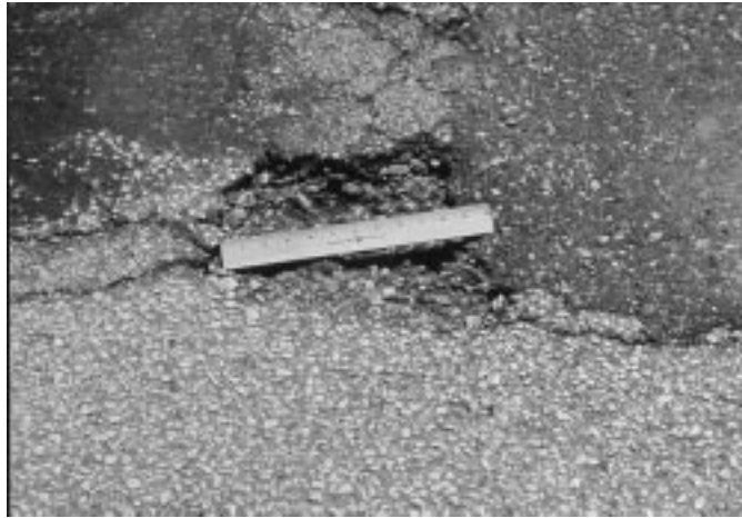
FIG. X1.35 Low-Severity Pothole
