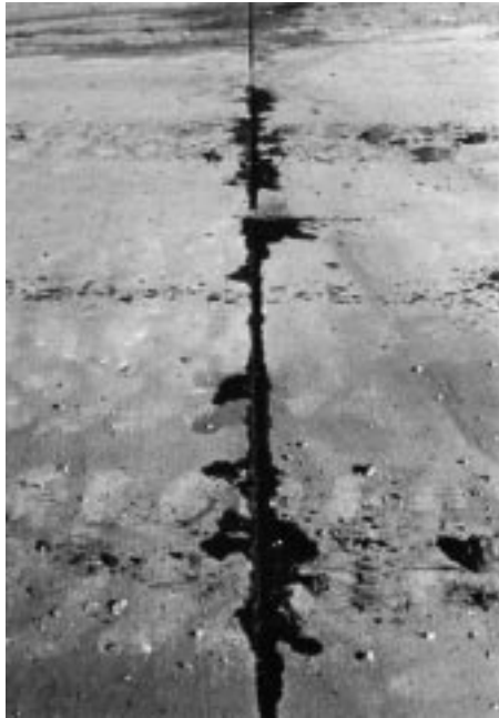
FIG. X2.33 Pumping
