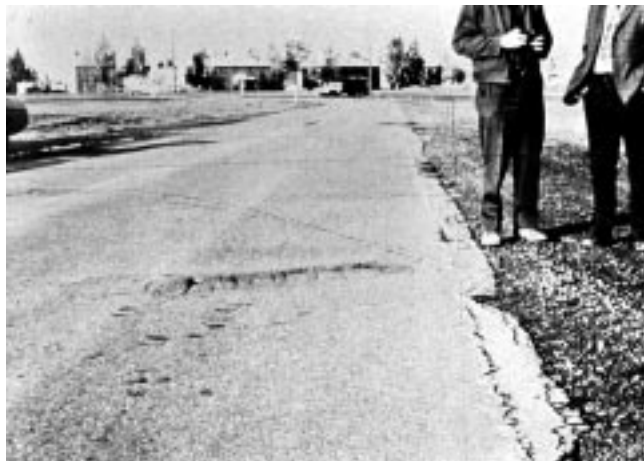
FIG. X1.11 Medium-Severity Bumps and Sags
