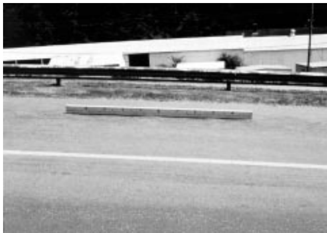
FIG. X1.14 Medium-Severity Corrugation
