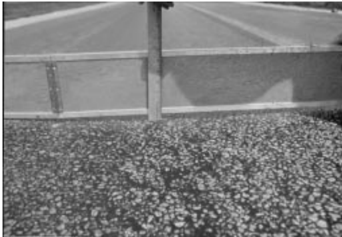
FIG. X1.42 Medium-Severity Rutting
