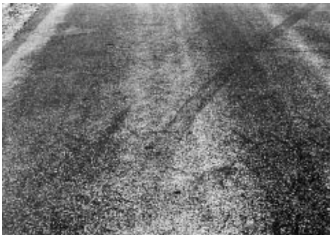
FIG. X1.4 Low-Severity Bleeding
