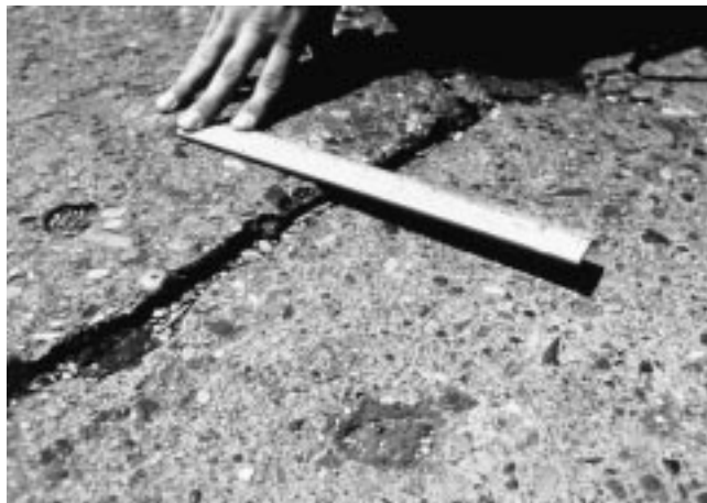
FIG. X2.14 Medium-Severity Faulting
