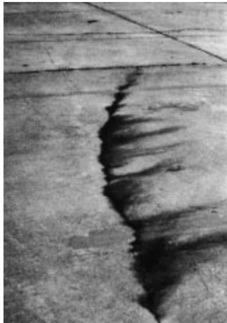
FIG. X2.34 Pumping
