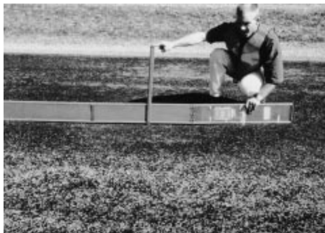
FIG. X1.16 Low-Severity Depression
