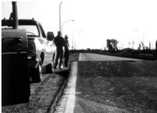
FIG. X2.3 High-Severity Blowup/Buckling
