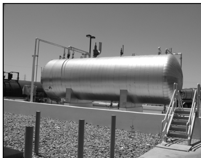
Figure 202-P1 INSULATED HORIZONTAL PRESSURE VESSEL
