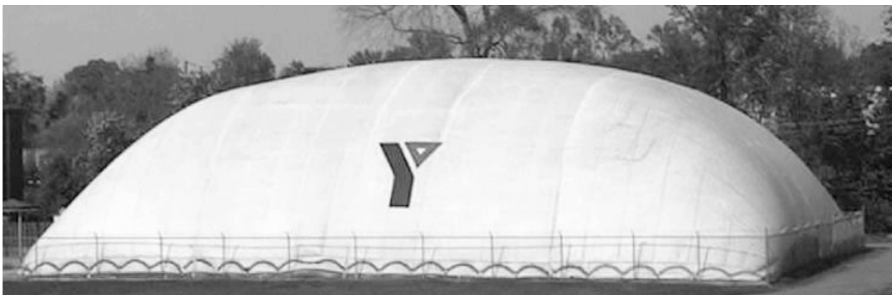
Figure 202-A2 AIR-SUPPORTED MEMBRANE STRUCTURE—SWIMMING POOL COVER
