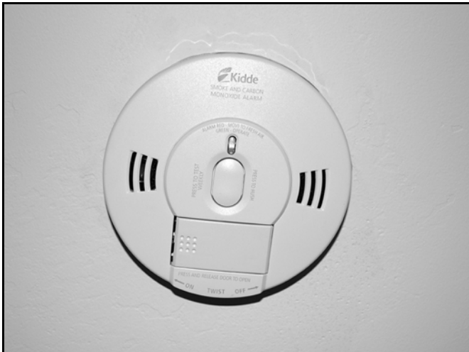
Figure 915.4.3 COMBINATION CARBON MONOXIDE AND SMOKE ALARM
