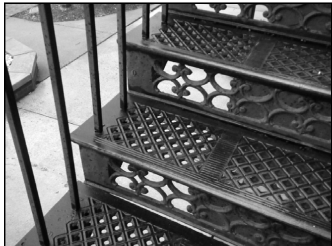
Figure 1011.7.1 OPEN TREAD IN ACCORDANCE WITH EXCEPTION 1
