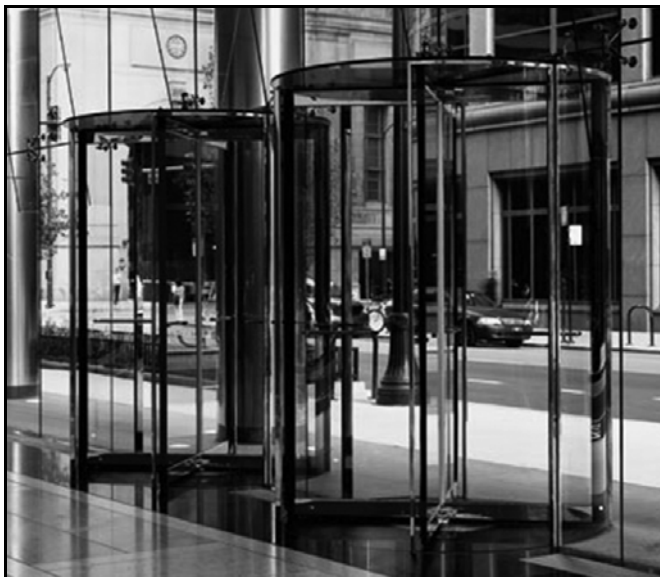
Figure 1010.1.4.1(3) EXAMPLE OF MANUAL REVOLVING DOOR (7-FOOT DIAMETER)
