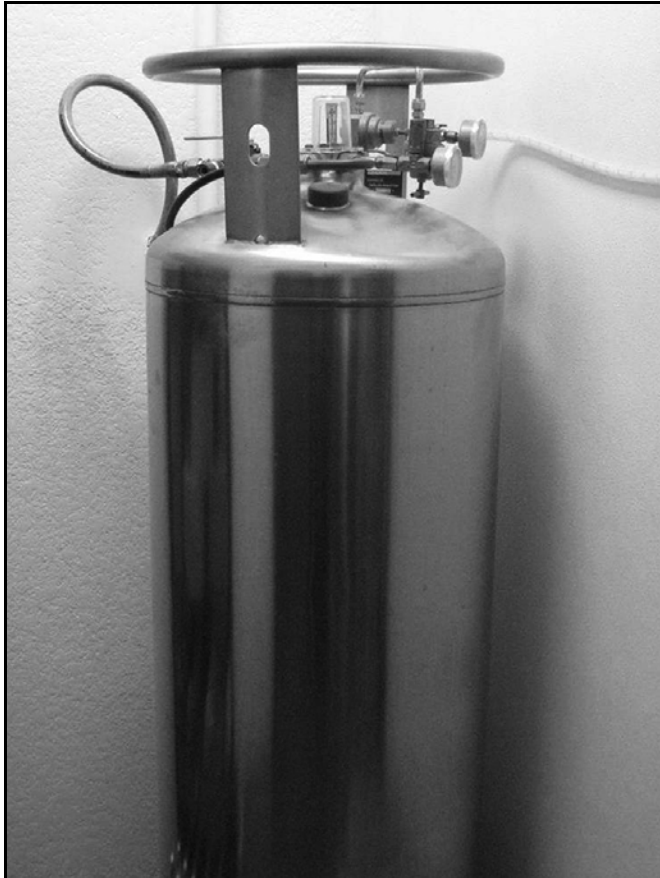
Figure 5307.3(2) BULK CO 2 CYLINDER IN A CARBONATED BEVERAGE DISPENSING SYSTEM
