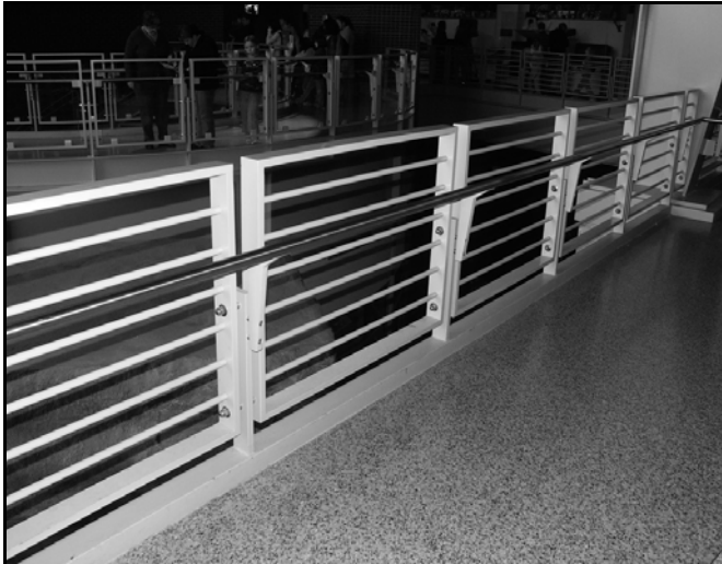
Figure 1015.4(3) EXAMPLE OF GUARD WITH HORIZONTAL MEMBERS
