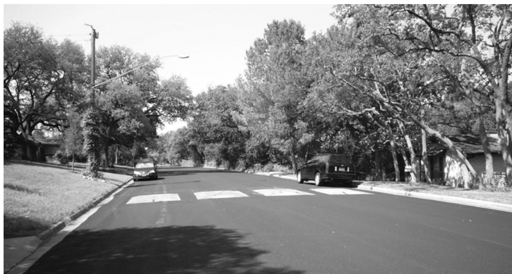
Figure 202-T2 SPEED PILLOW TRAFFIC CALMING DEVICE
