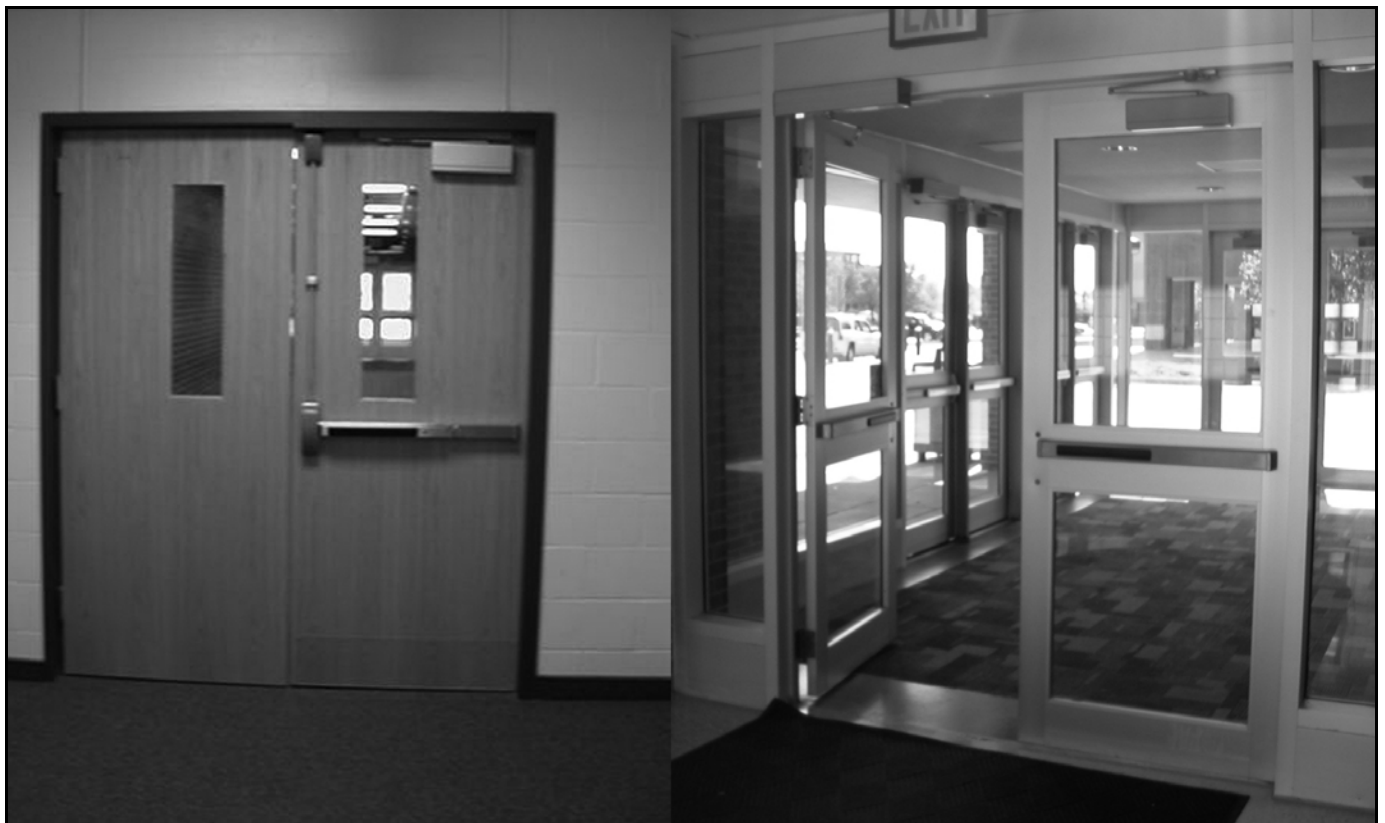
Figure 1010.1.10.1(2) EXAMPLES OF TYPICAL PANIC HARDWARE
