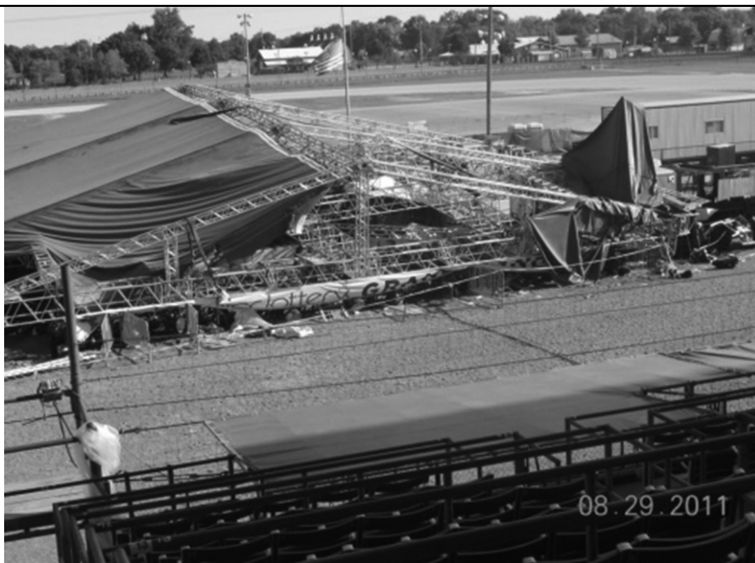
Figure 3105.1(2) TEMPORARY STAGE CANOPY AFTER STRUCTURAL COLLAPSE AT THE INDIANA STATE FAIR—AUGUST 13, 2011 (Photo courtesy of Anne vonWeller)
