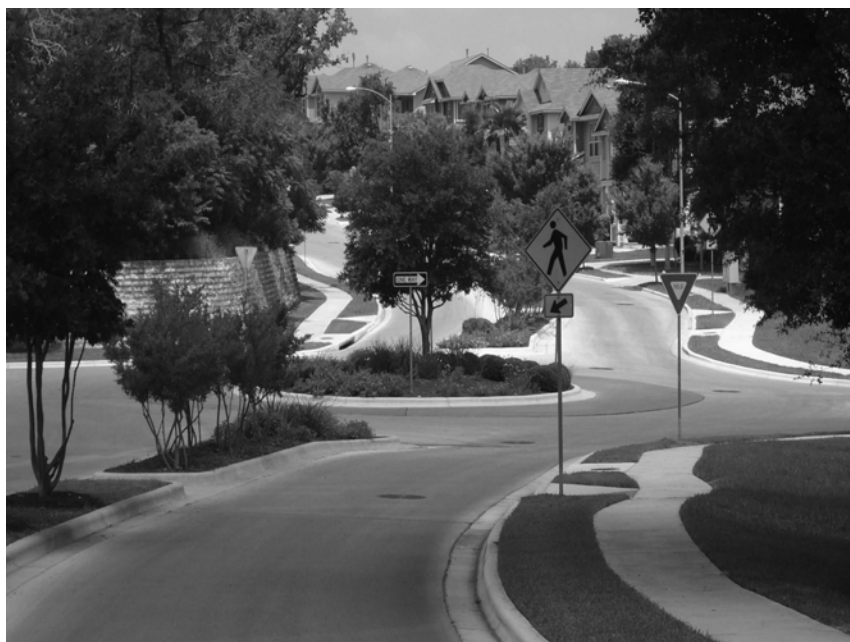
Figure 202-T3 ROUNDBOUT TRAFFIC CALMING DEVICE
