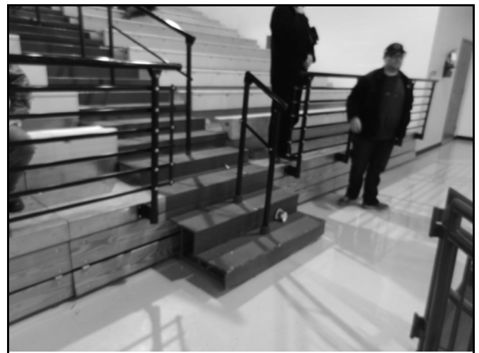
Figure 1029.9.7(2) EXAMPLE OF A CONTINUATION OF A STEPPED AISLE DOWN TO A FLOOR
