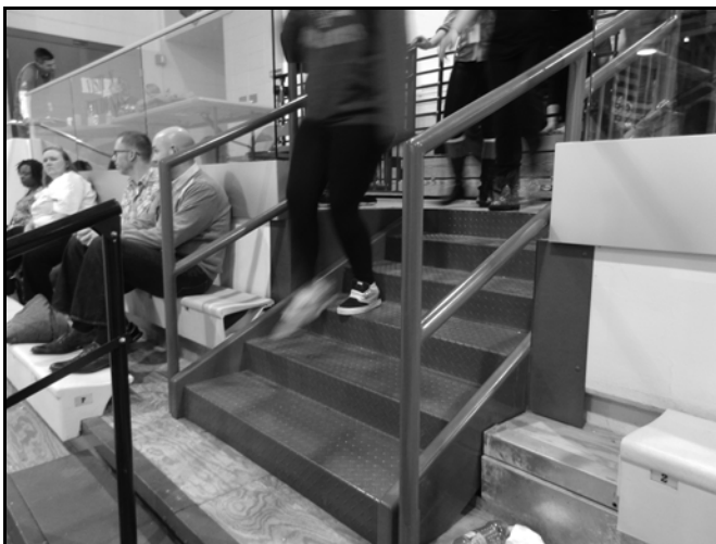
Figure 1029.9.7(1) EXAMPLE OF A CONTINUATION OF A STEPPED AISLE UP TO A CROSS AISLE
