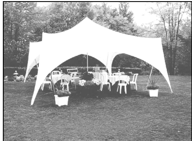
Figure 202-C1 EXAMPLE OF A FREE-STANDING MEMBRANE-COVERED CANOPY
