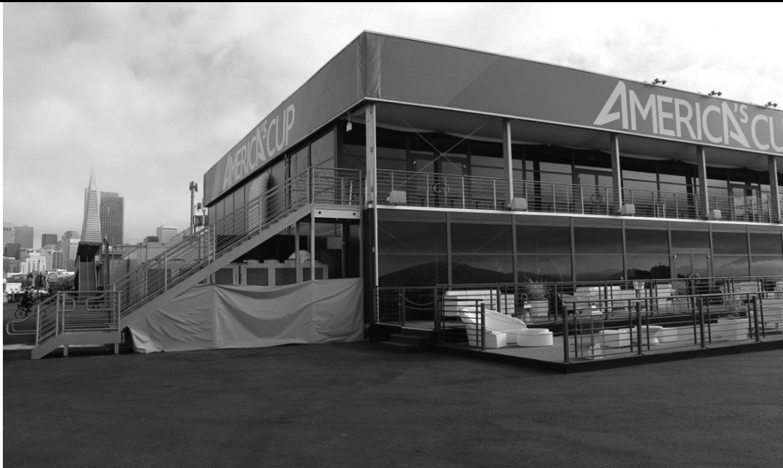
Figure 3103.9.1(1) TWO-STORY MEMBRANE STRUCTURE AT THE AMERICA'S CUP RACE (Photo courtesy of HTS-USA)
