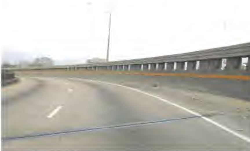
Figure 7-6. Texas Type TT Railing
