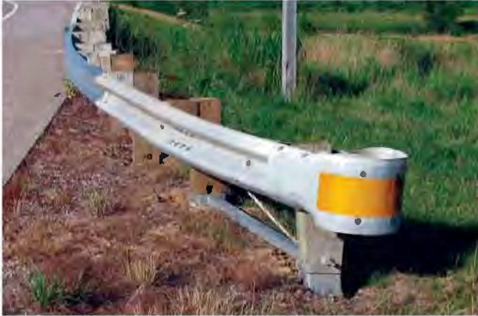
Figure 8-8. Modified Eccentric Loader Terminal (MELT)
