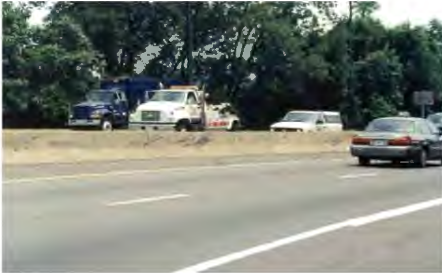
Figure 6-13. Concrete Safety-Shape Median Barrier
