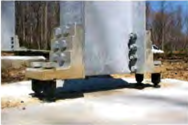
Figure 4-4. Multidirectional Coupler
