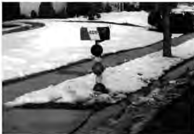
Figure 11-2. Examples of Hazardous Single Mailbox Installations
