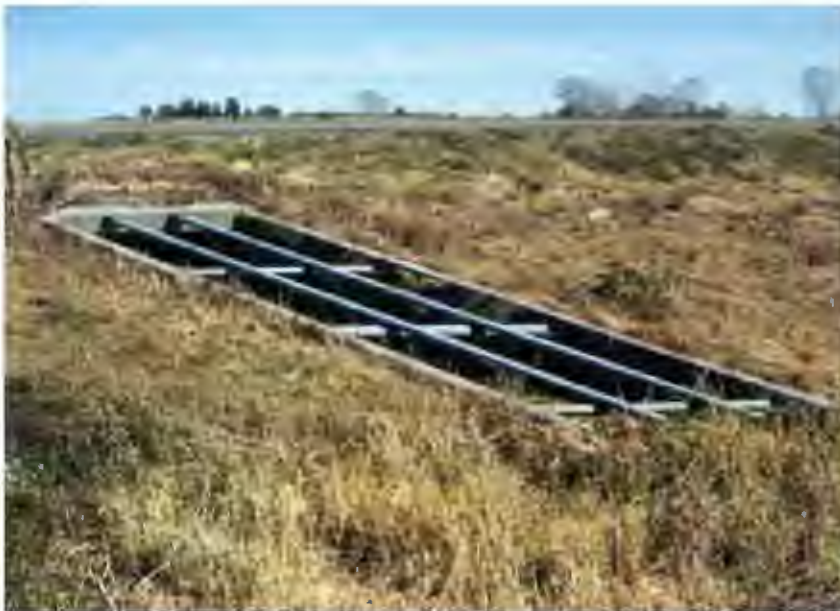
Figure 3-9. Safety Treatment for Cross-Drainage Culvert
