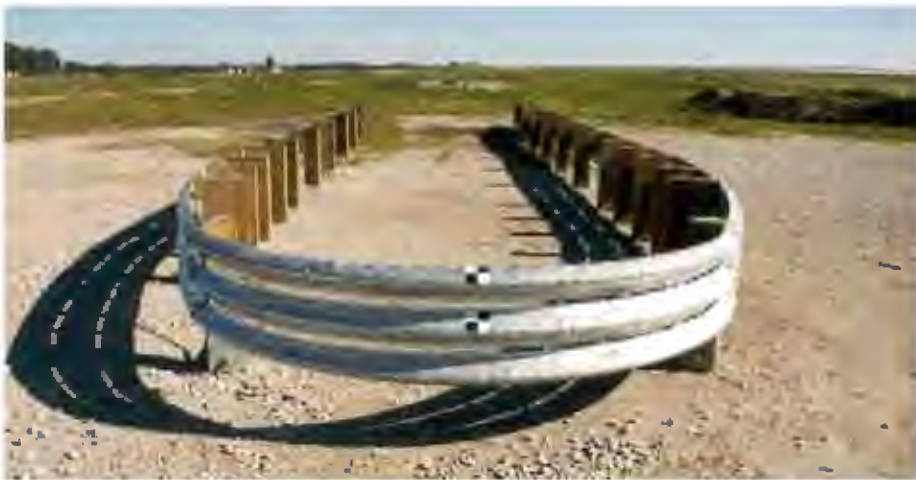
Figure 8-20. Bullnose Guardrail System
