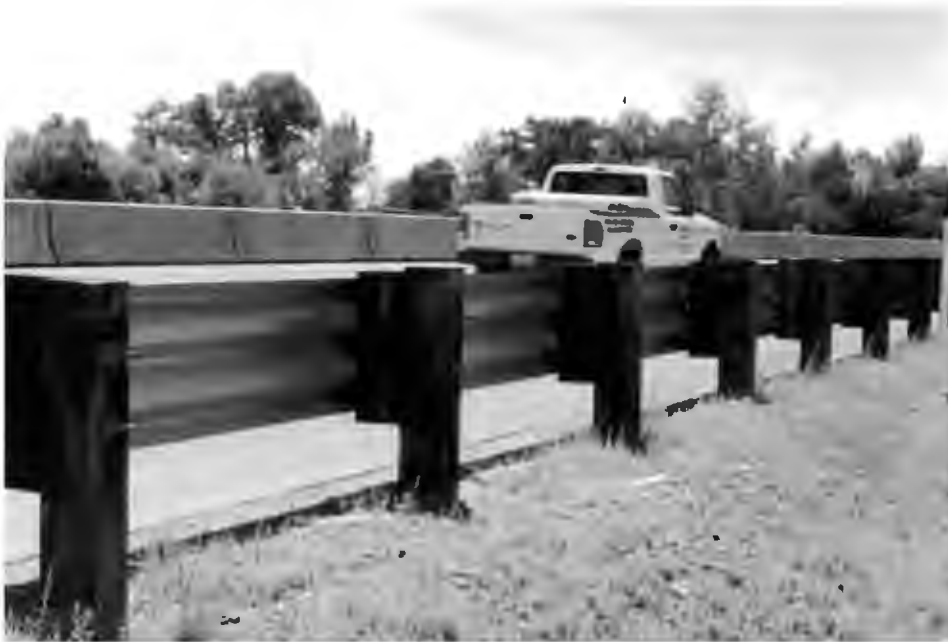
Figure 5-14. Wood-Post Thrie-Beam Guardrail
