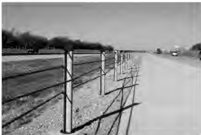
Figure 6-4. Brifen Wire Rope Safety Fence
