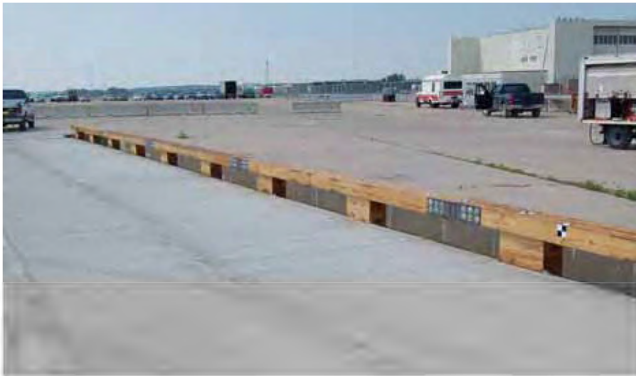
Figure 7-1. Curb Type Glu-Lam Timber Railing
