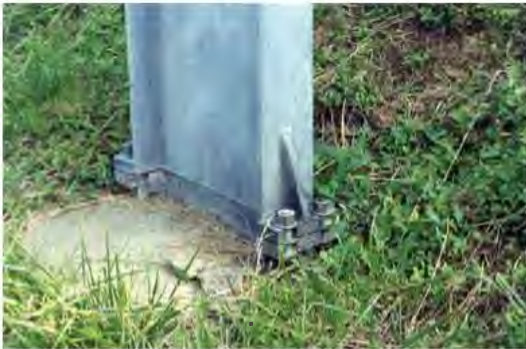
Figure 4-5. Typical Unidirectional Slip Base
