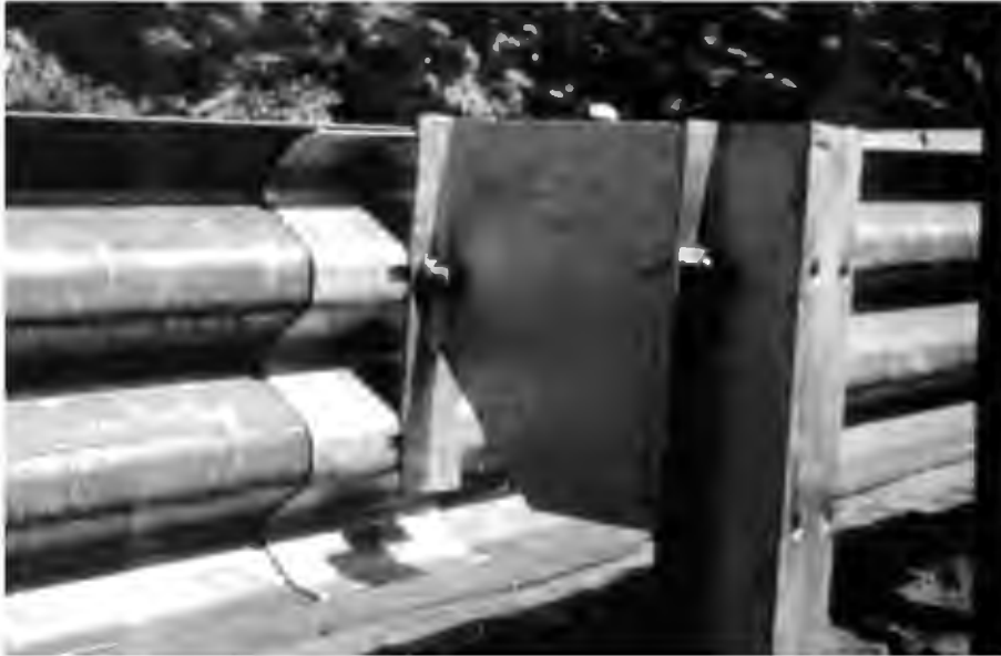
Figure 5-15. Modified Thrie-Beam Guardrail
