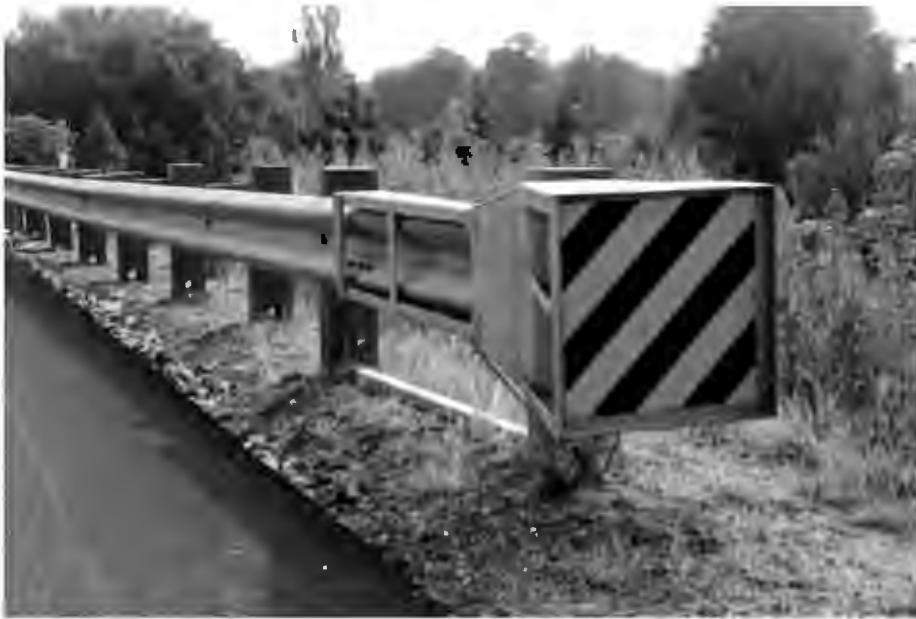
Figure 8-13. Sequential Kinking Terminal (SKT-350™)
