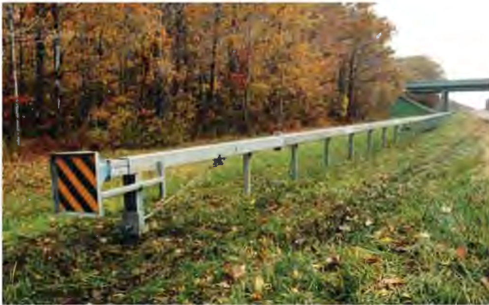
Figure 8-19. Bursting Energy Absorbing Terminal (BEAT™)
