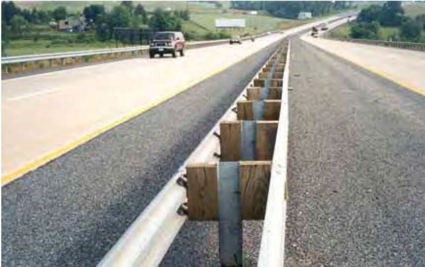
Figure 6-10. Strong-Post W-Beam Median Barrier
