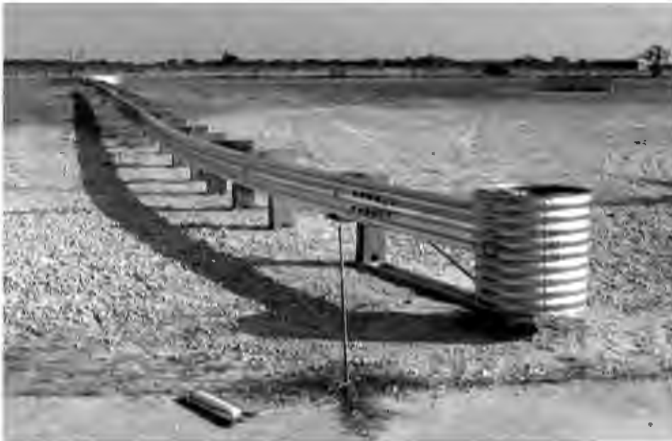
Figure 8-7. Eccentric Loader Terminal (ELT)
