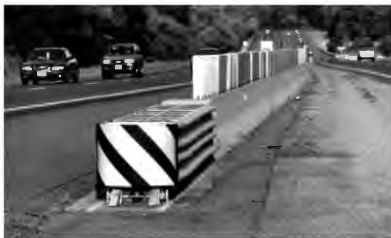
Figure 8-29. Trinity Attenuating Crash Cushion (TRACC™)
