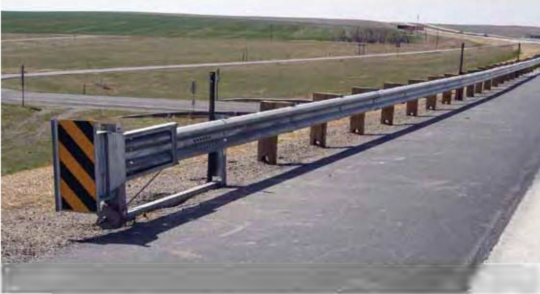
Figure 8-12. Extruder Terminal (ET-Plus™)
