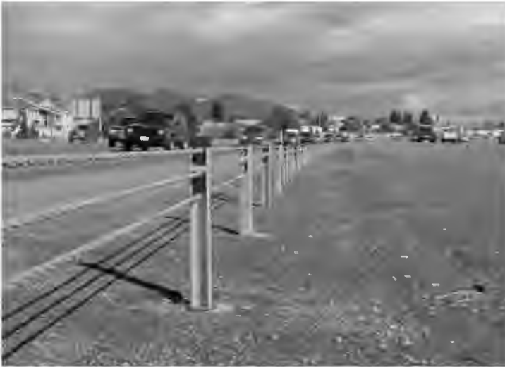
Figure 6-5. The Cable Safety System (CASS)
