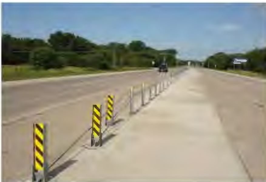
Figure 8-5. CASS™ Cable Terminal (CCT)
