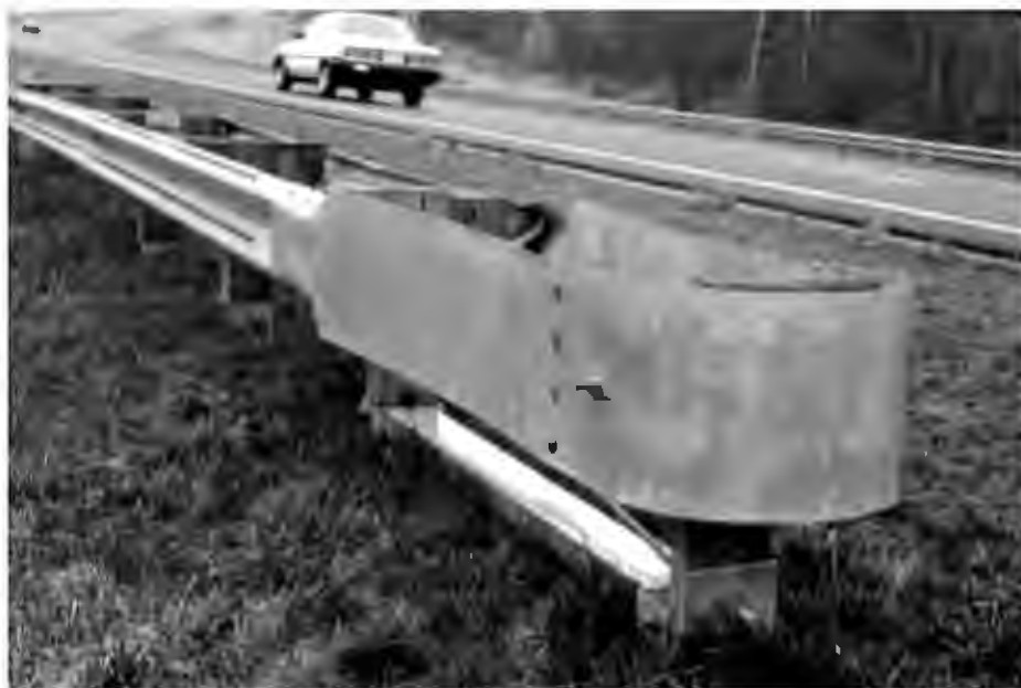
Figure 8-15. Crash Cushion Attenuating Terminal (CAT-350™)
