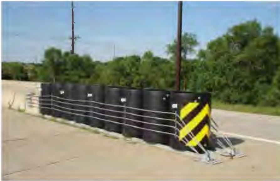
Figure 8-36. Reusable Energy-Absorbing Crash Terminal (REACT 350®)
