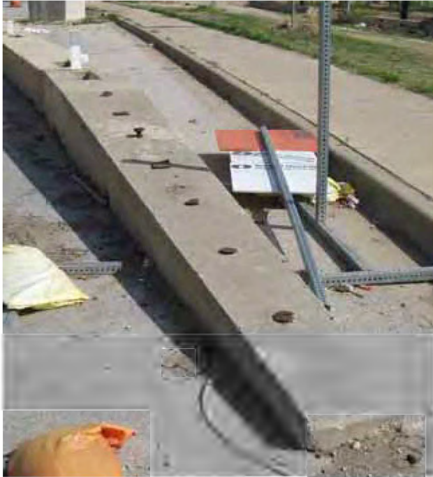
Figure 9-22. Slope-End Treatment for Low-Profile Portable Concrete Barrier
