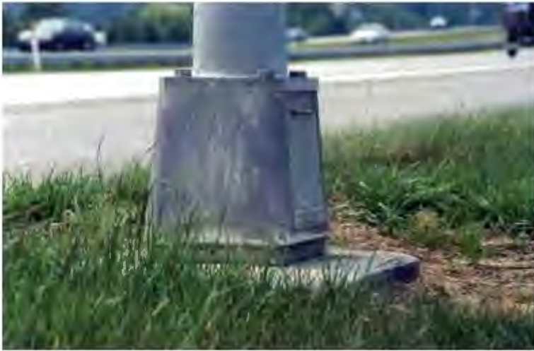
Figure 4-11. Example of a Cast Aluminum Frangible Luminaire
