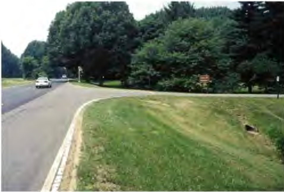
Figure 3-3. Suggested Design for Transverse Slopes
