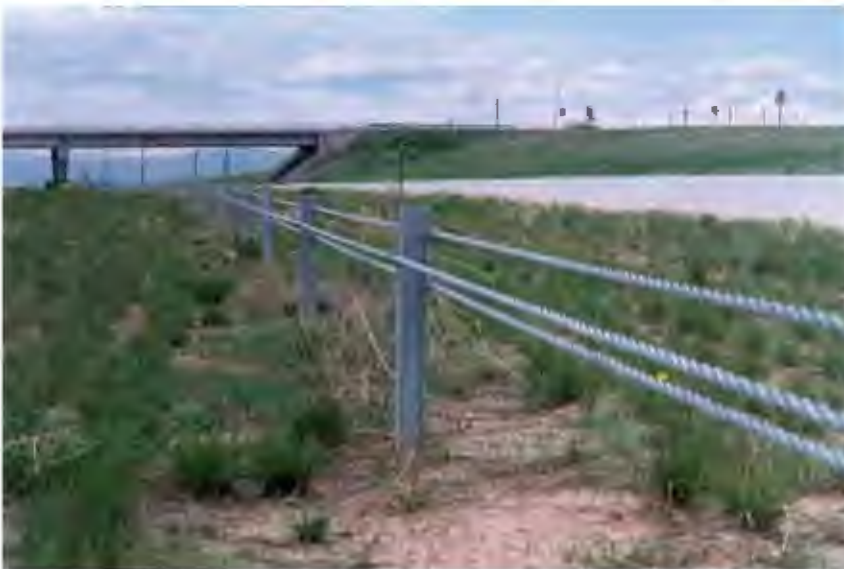
Figure 6-3. Three-Strand Cable Median Barrier
