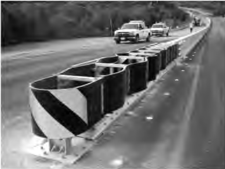
Figure 8-33. Hybrid Energy Absorbing Reusable Terminal (HEART™)
