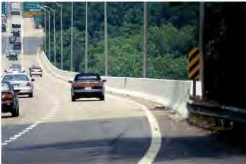
Figure 7-5. 1,067-mm [42-in.] Tall Concrete Safety-Shaped Bridge Railing
