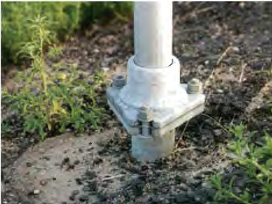
Figure 4-9. Multidirectional Slip Base for Small Signs
