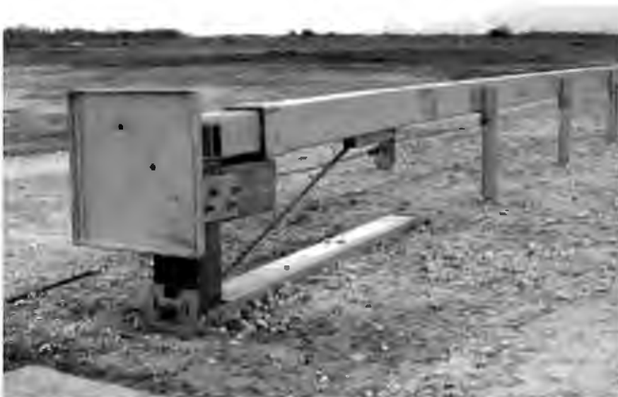
Figure 8-18. Wyoming Box-Beam End Terminal (WY-BET™)
