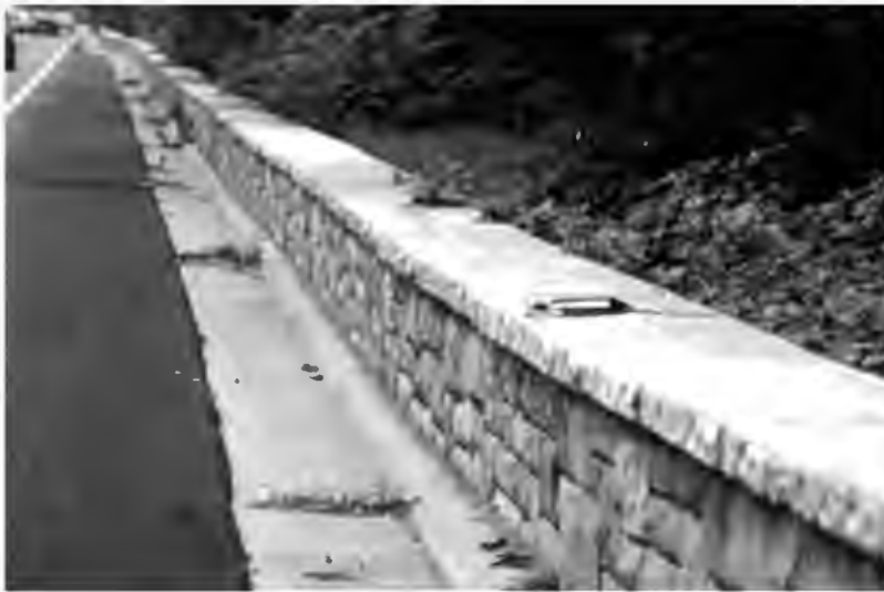
Figure 5-24. Precast Masonry Wall
