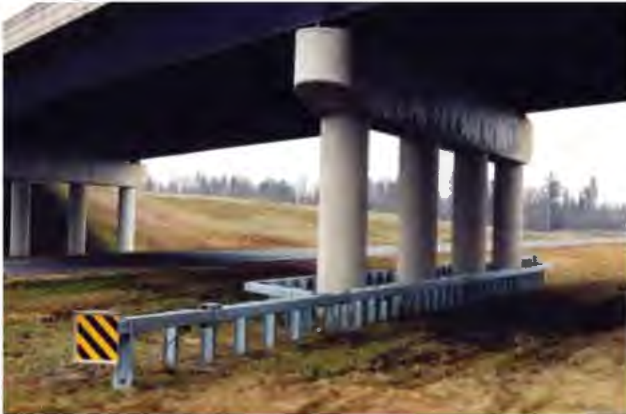
Figure 8-24. Bursting Energy Absorbing Terminal–Bridge Pier (BEAT-BP™) System
