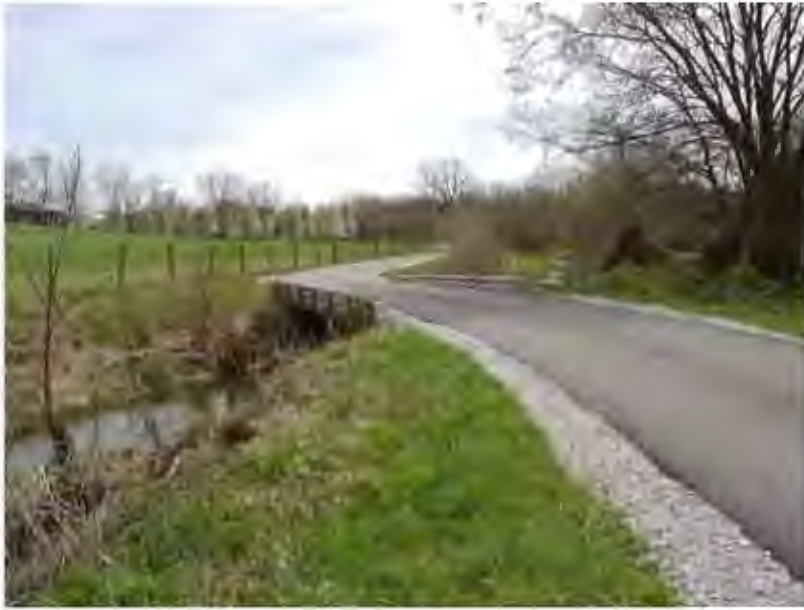
Figure 12-5. Typical Low-Volume Rural Bridge
