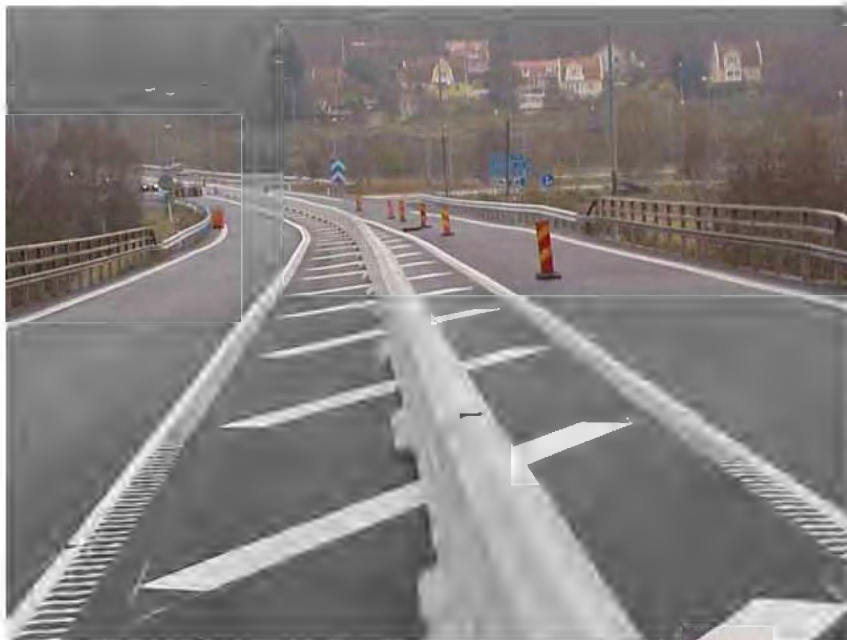
Figure 9-6. GPLINK® Pre-Cast Temporary Concrete Barrier
