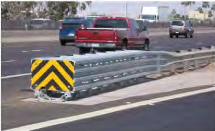
Figure 8-37. Smart Cushion Innovations (SCI-100GM) Crash Cushion
