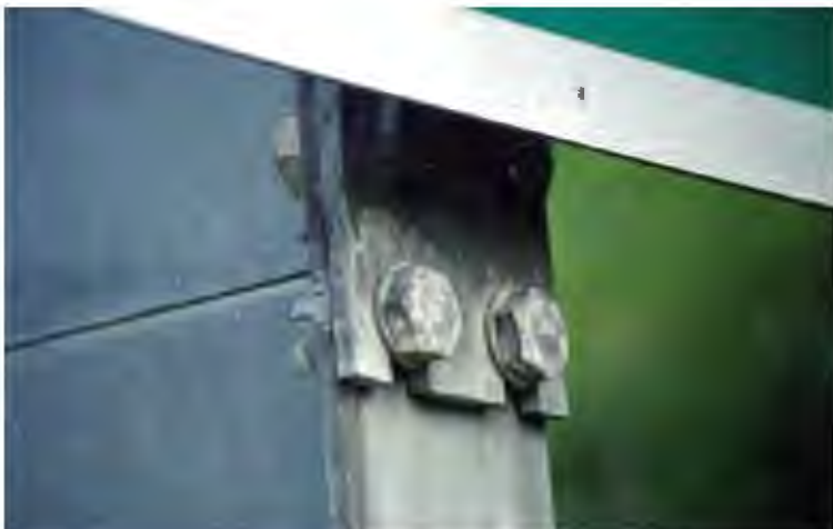
Figure 4-6. Slotted Fuse Plate Design
