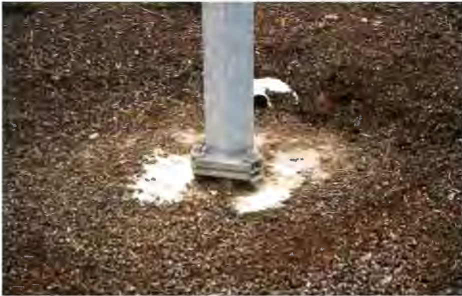
Figure 4-10. Oregon 3-Bolt Slip Base
