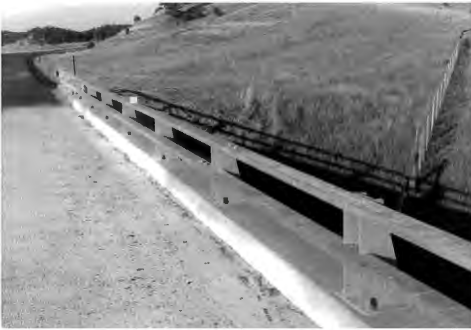
Figure 7-3. Wyoming Two-Tube Bridge Railing
