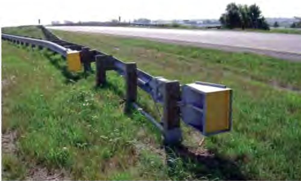
Figure 8-16. FLEAT Median Terminal (FLEAT-MT™)
