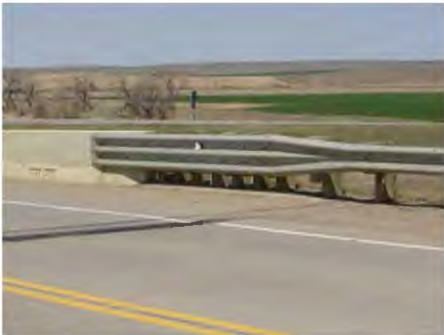
Figure 7-12. Thrie-Beam Transition to Modified Concrete Safety Shape
