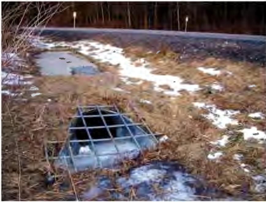
Figure 12-3. Reinforcing Steel Grate
