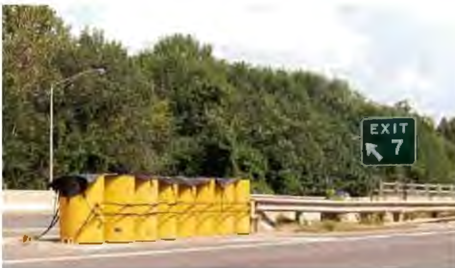
Figure 8-26. Narrow Connecticut Impact Attenuation System (NCIAS)
