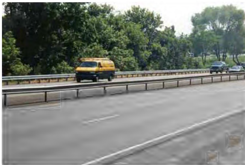
Figure 6-2. Weak-Post W-Beam Median Barrier
