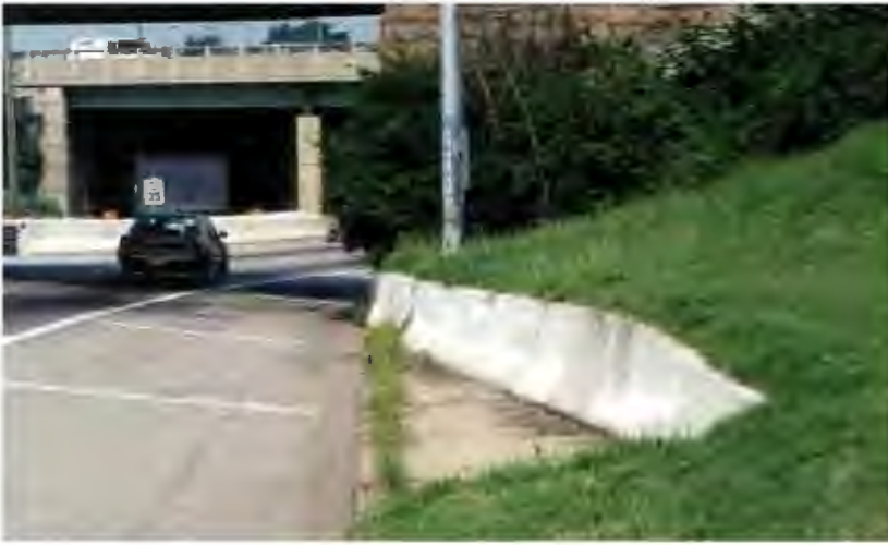
Figure 8-44. Barrier Anchored in Backslope
