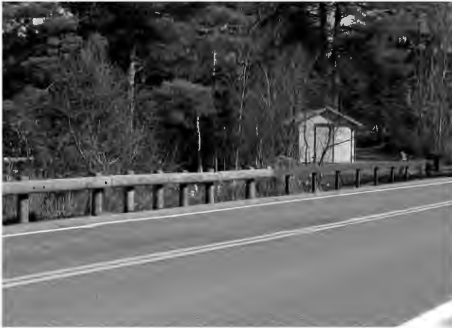
Figure 5-7. Ironwood Aesthetic Guardrail
