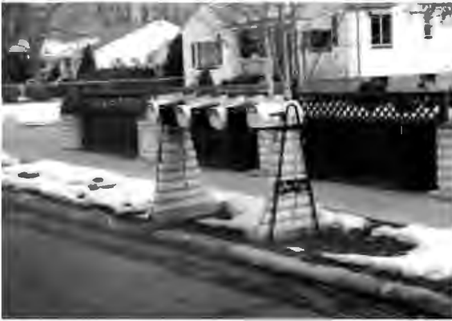
Figure 11-3. Examples of Hazardous Multiple Mailbox Installations
