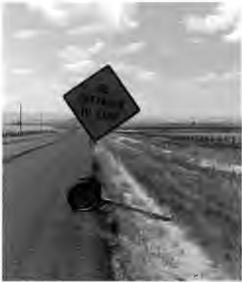
Figure 9-38. Montana Wheeled Portable Sign Support
