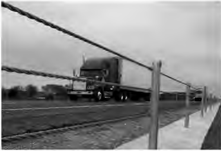
Figure 6-8. Gibraltar Cable Barrier System
