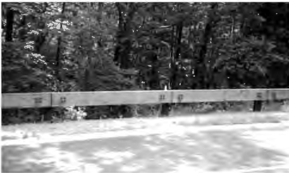
Figure 5-17. Merritt Parkway Aesthetic Guardrail
