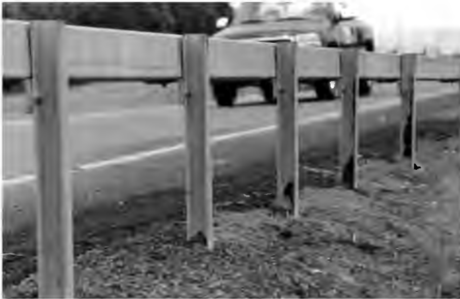
Figure 5-8. Weak-Post Box Beam Guardrail
