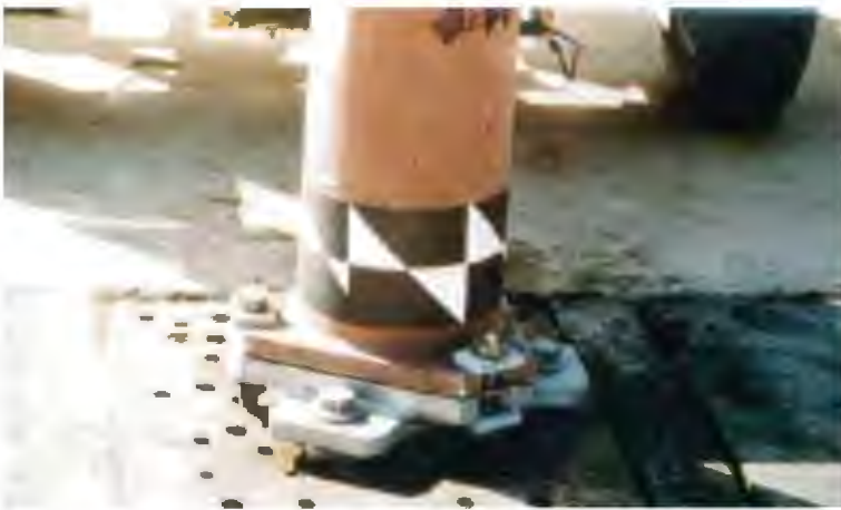
Figure 4-12. Example of a Luminaire Slip Base Design
