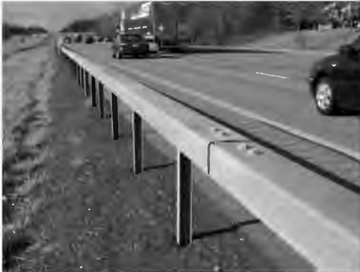
Figure 6-9. Box-Beam Median Barrier
