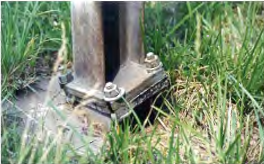
Figure 4-8. Unidirectional Slip Base for Small Signs
