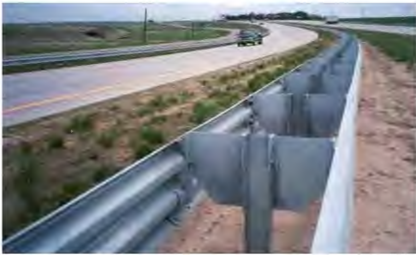
Figure 6-11. Modified Thrie-Beam Median Barrier
