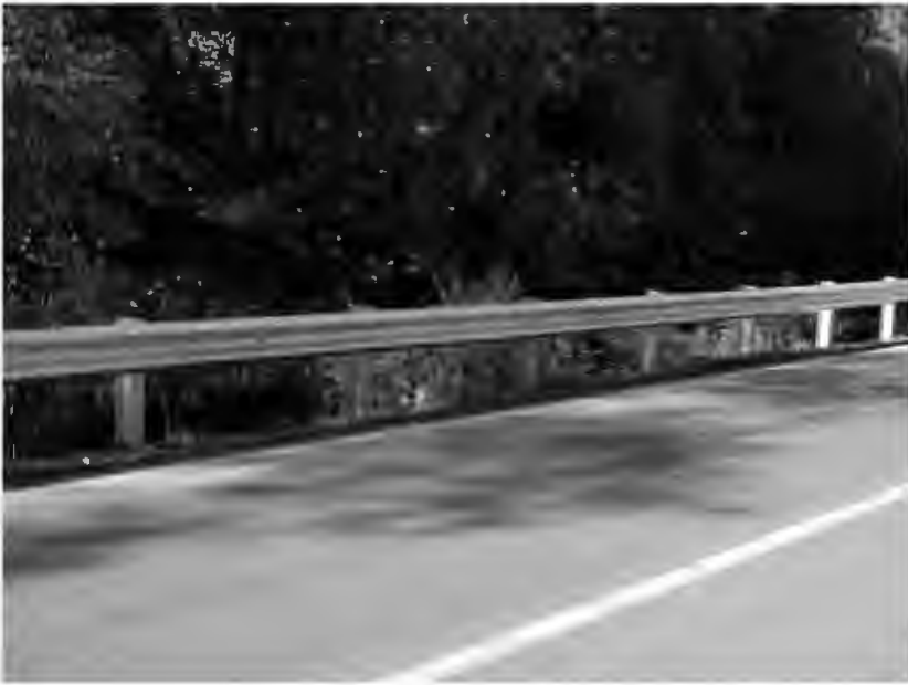
Figure 5-12. Trinity T-31™ Guardrail System
