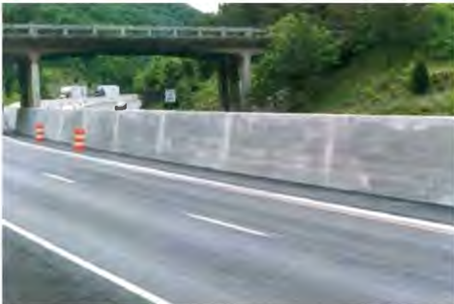
Figure 6-14. Single-Slope Concrete Median Barrier
