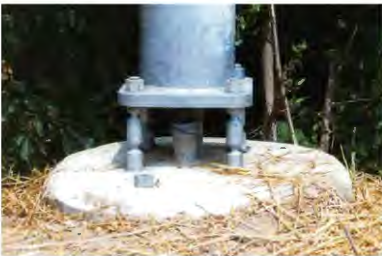
Figure 4-13. Example of a Frangible Coupling Design
