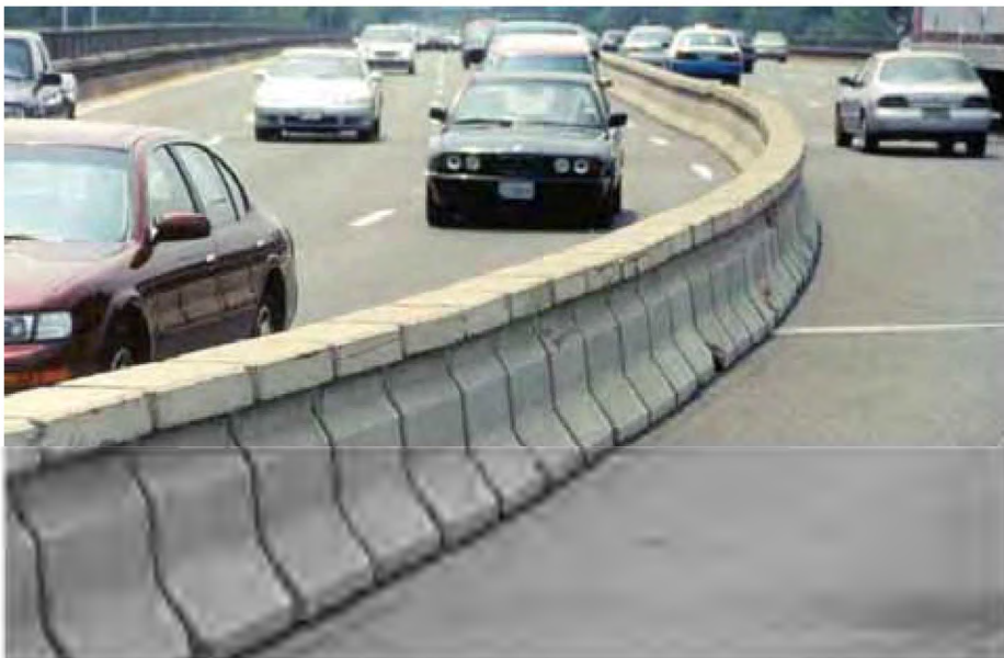
Figure 6-15. Standard Quickchange® Moveable Barrier System
