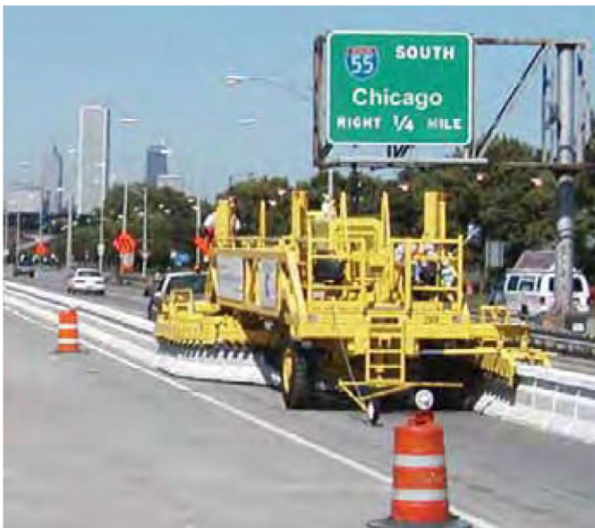
Figure 9-18. Quickchange® Barrier System
