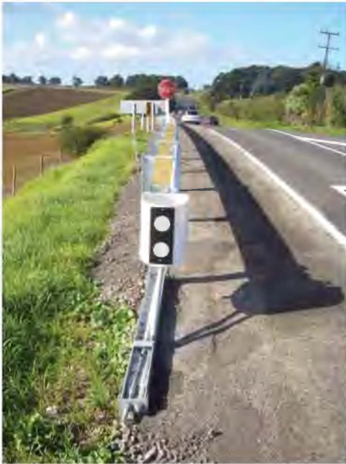
Figure 8-11. X-Tension Guardrail End Terminal
