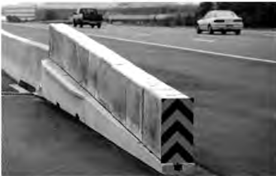
Figure 8-22. Advanced Dynamic Impact Extension Module (ADIEM™)
