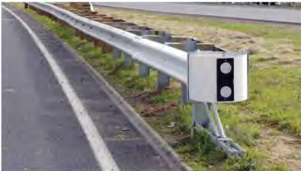
Figure 8-17. X-Tension™ Median Attenuator System (X-MAS)
