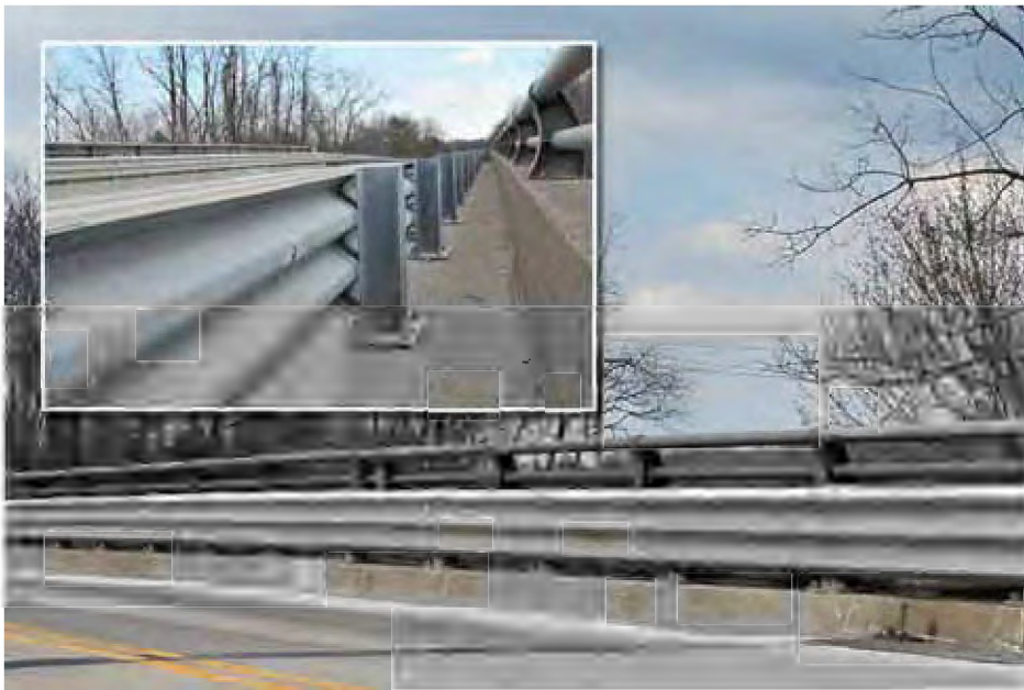
Figure 7-10. Delaware Thrie-Beam Retrofit
