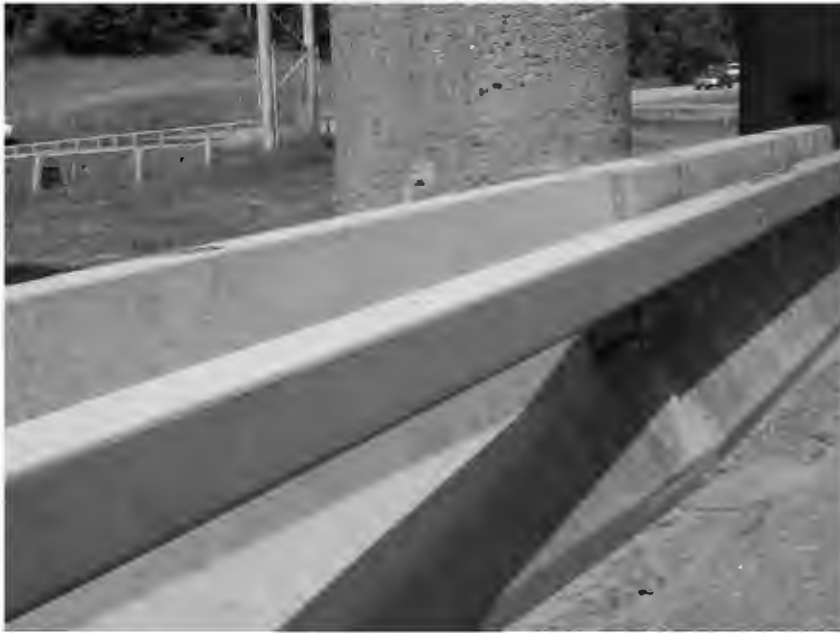
Figure 6-12. New York Modification of Concrete Barrier
