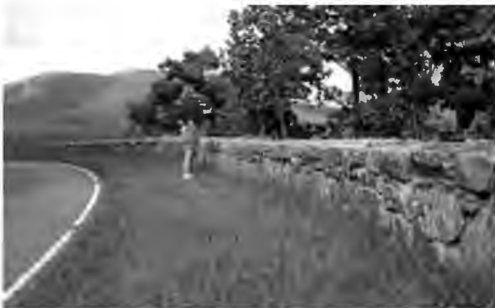
Figure 5-23. Stone Masonry Wall
