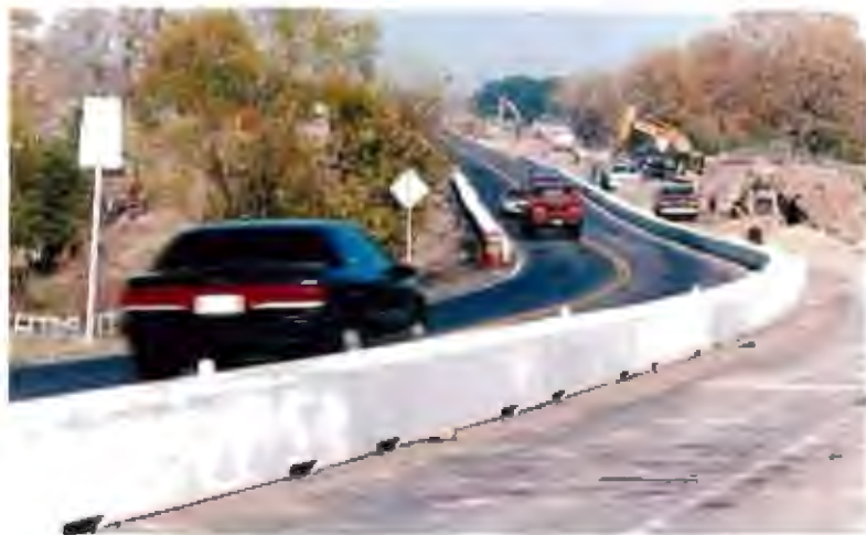
Figure 9-19. Low-Profile Barrier System
