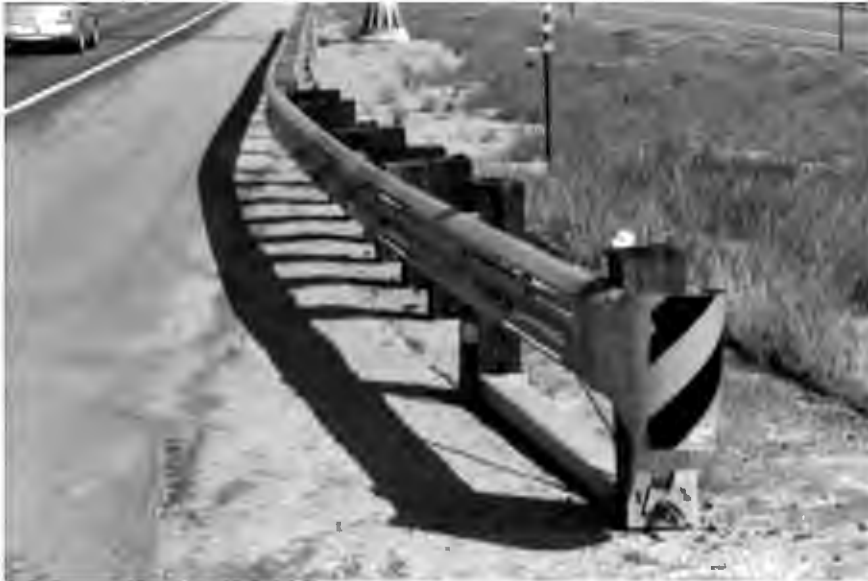
Figure 8-10. Slotted Rail Terminal (SRT-350™)
