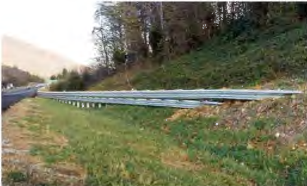
Figure 8-6. W-Beam Guardrail Anchored in Backslope
