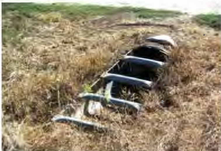
Figure 3-12. Safety Treatment for Parallel Drainage Pipe
