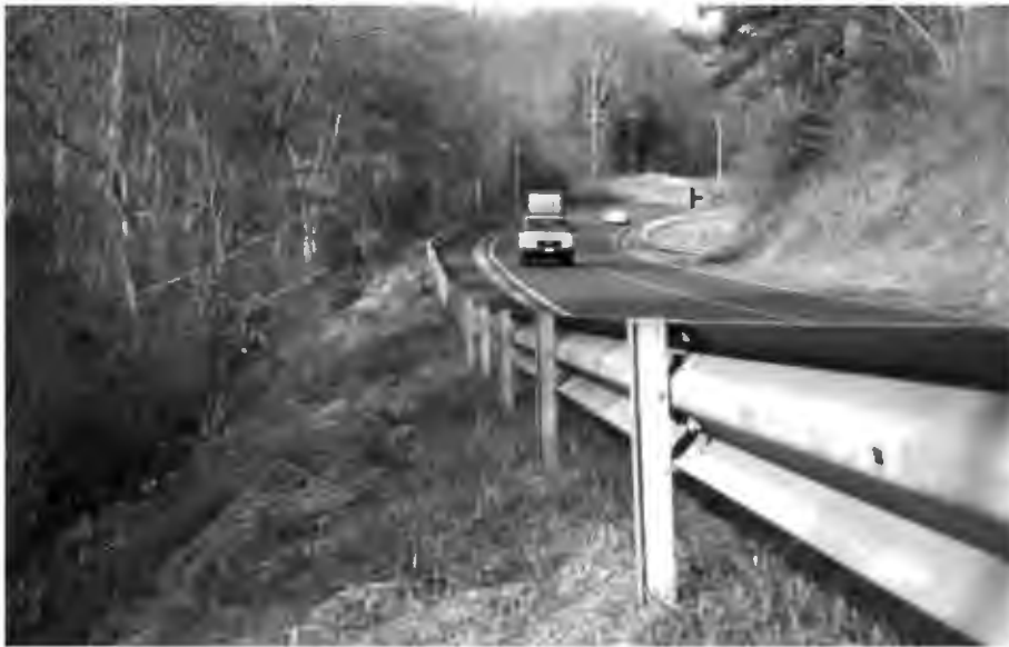
Figure 5-6. Weak-Post W-Beam Guardrail
