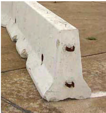
Figure 9-1. Iowa Temporary Concrete Barrier
