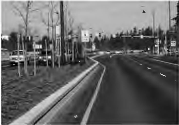
Figure 5-19. Low Profile Barrier
