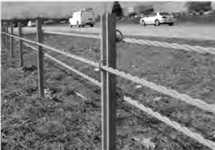
Figure 6-6. NU-CABLE™ High-Tension Cable System
