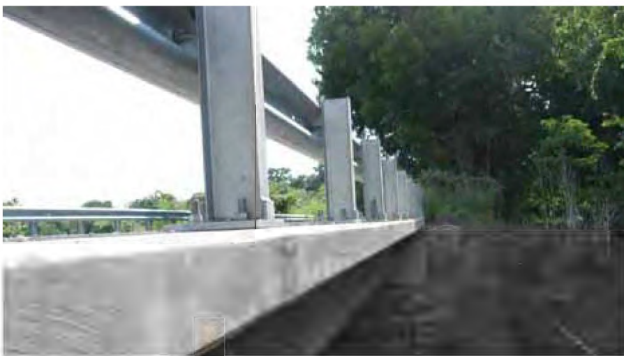
Figure 7-2. Texas T-6 Railing
