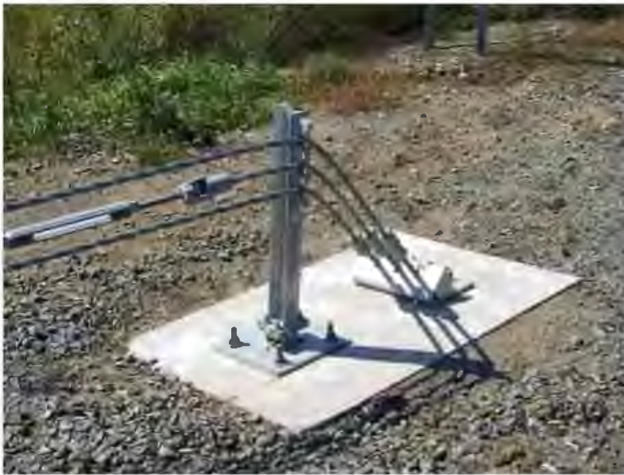
Figure 8-4. Three-Strand Cable Terminal
