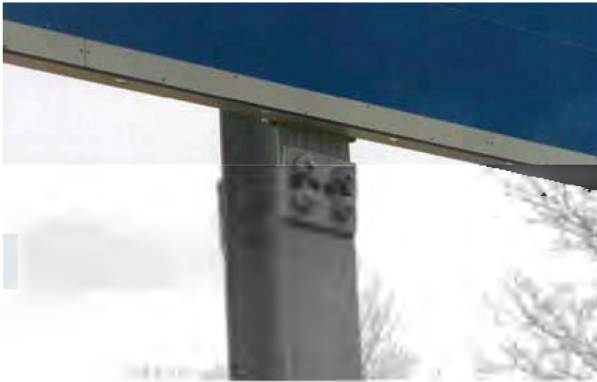
Figure 4-7. Perforated Fuse Plate Design
