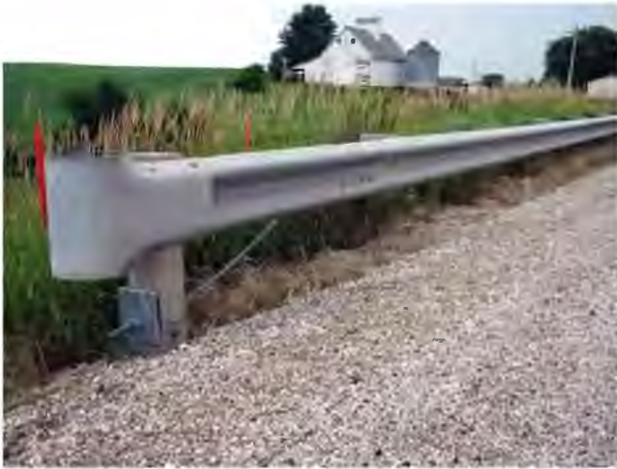
Figure 8-1. Trailing End W-Beam Guardrail Anchorage
