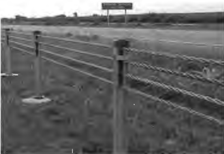
Figure 6-7. Safence Cable Barrier System
