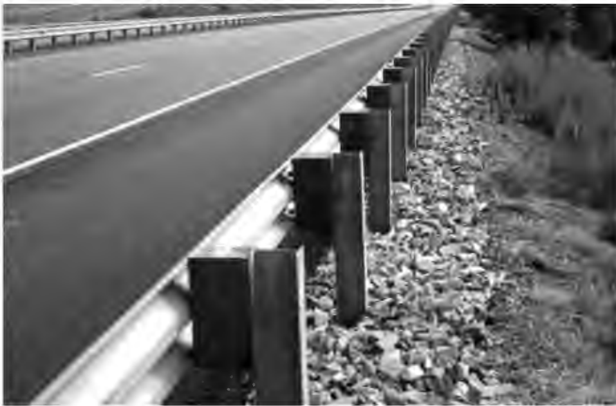
Figure 5-9. Steel-Post W-Beam Guardrail with Wood Blockouts
