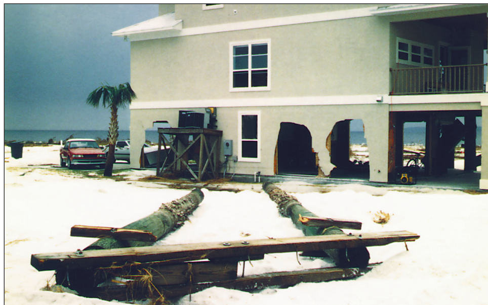
Figure 1-12. Pier pilings were carried over 2 miles by the storm surge and waves of Hurricane Opal (1995) before coming to rest against this elevated house in Pensacola Beach, Florida.
