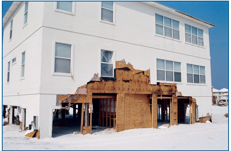
Siding on the non-breakaway portions of this elevated building was extended over breakaway enclosure walls and was damaged when breakaway walls failed under flood forces.
