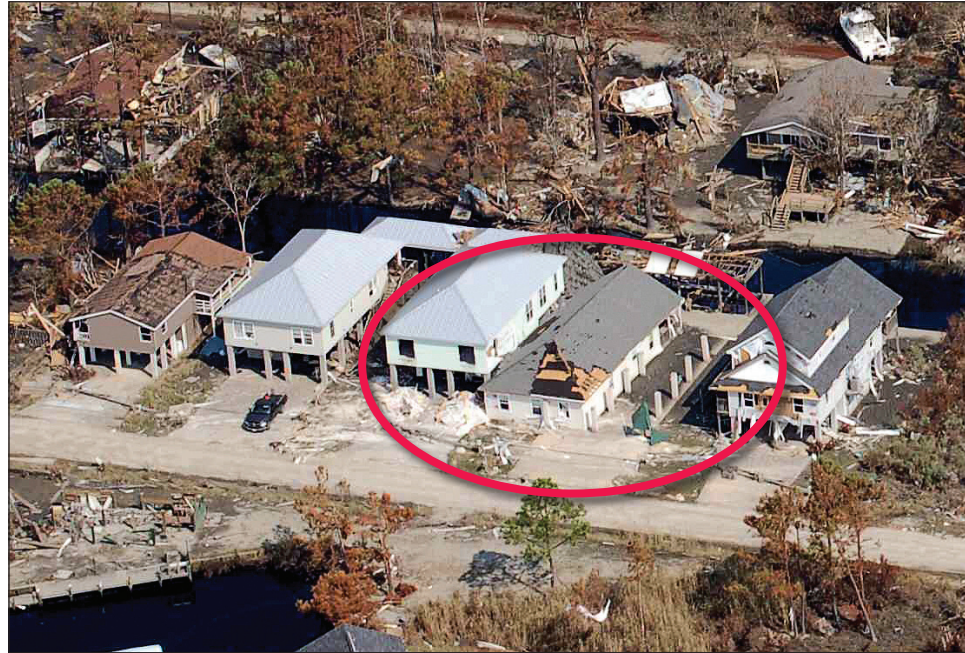
Figure 1. Damage to residential properties as a result of Hurricane Katrina's winds and storm surge. Note the building that was knocked off its foundation (circled).
