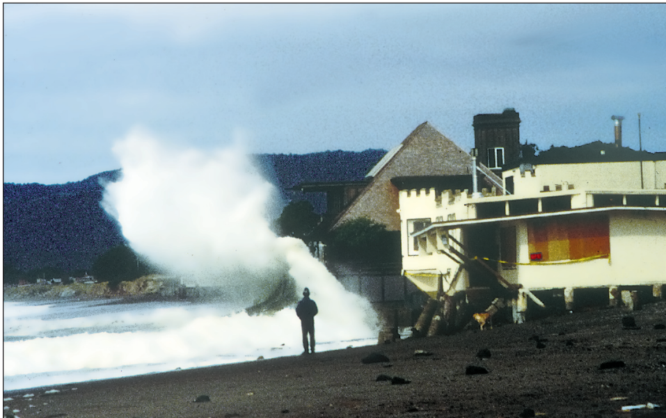
Figure 1-10. Storm waves breaking against a seawall in front of a coastal residence at Stinson Beach, California
