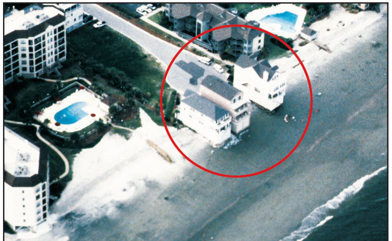
Figure 1. Well-built but poorly sited building.
