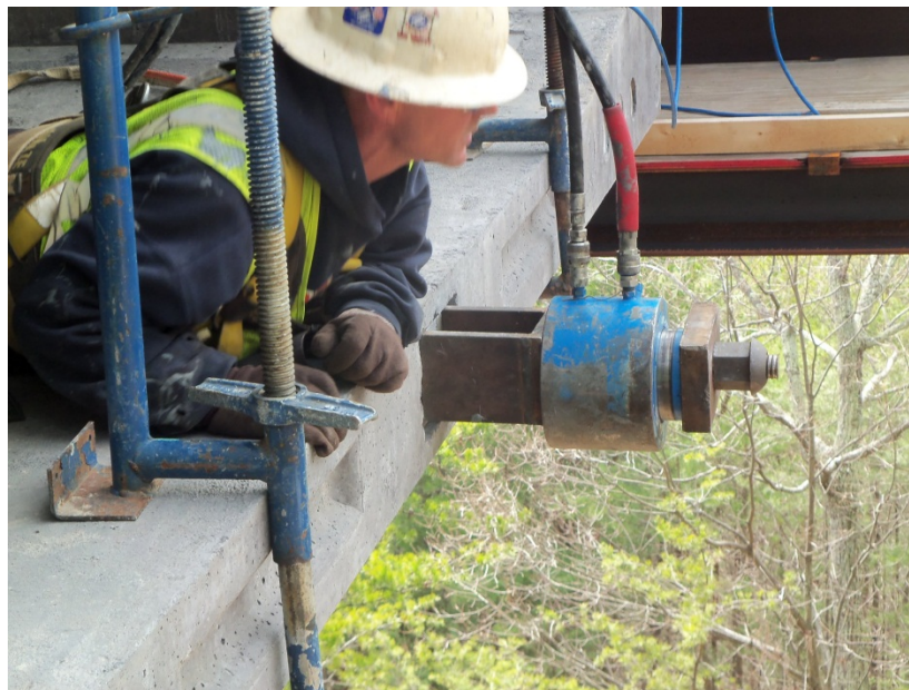
Figure 1.36 - Stressing Temporary Bar in Bottom Slab of the Foothills Parkway Bridge No. 2
