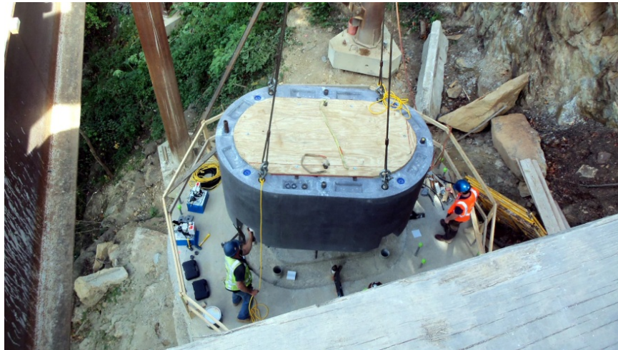
Figure 1.32 - Precast Hollow Segmental Piers, Foothills Bridge No. 2
