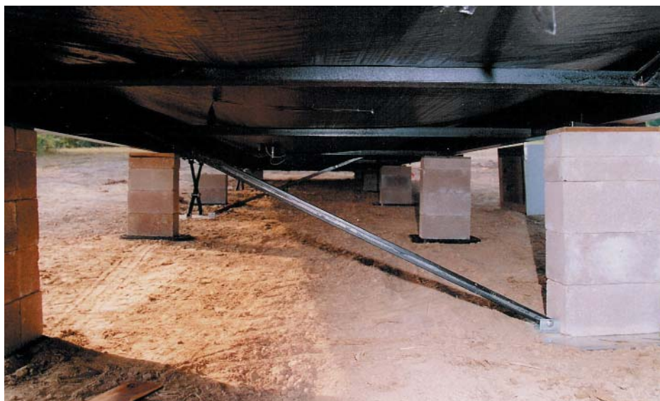
Figure 4.6 Lateral and longitudinal (rear system) protection shown under home.
