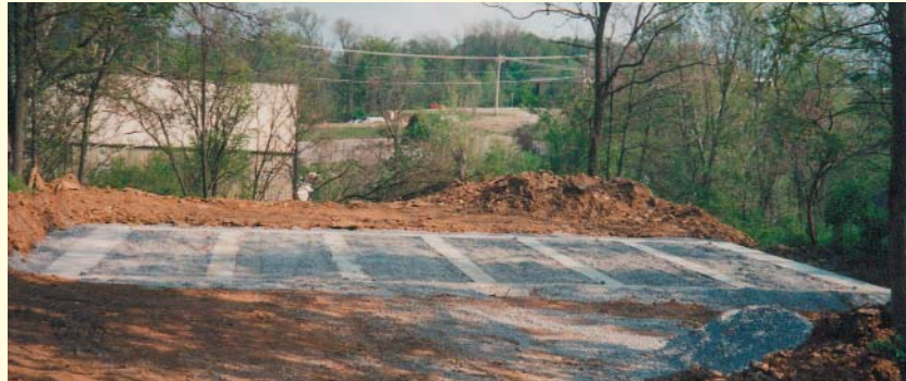
Figure 3.25 Open cells filled with crushed rock.
