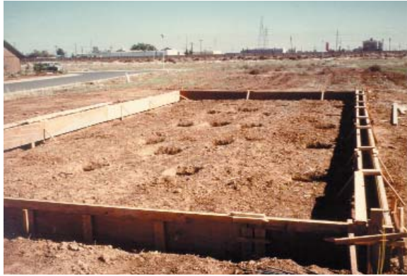
Figure 3.14 Forms ready for concrete pour.
