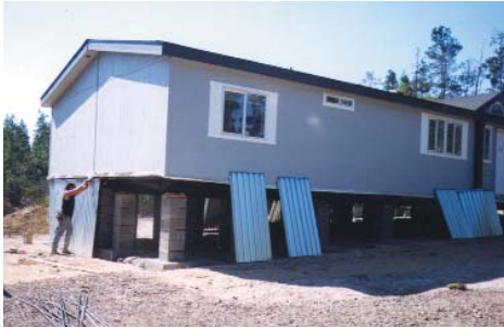
Figure 4.10 A "kit" of panel lengths matches each installation.
