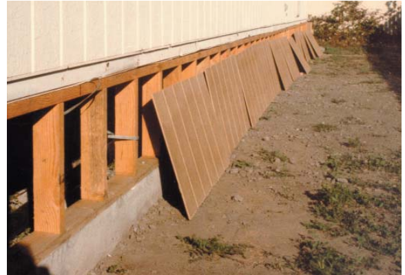
Figure 3.15 Ponywall construction method.
