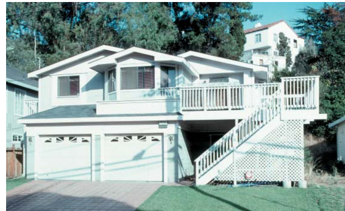
Figure 3.62 Garage/basement on upslope lot in Oakland, California.
