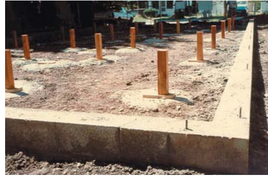
Figure 1.3 Some foundations use a combination of interior piers and perimeter walls to support the home.
