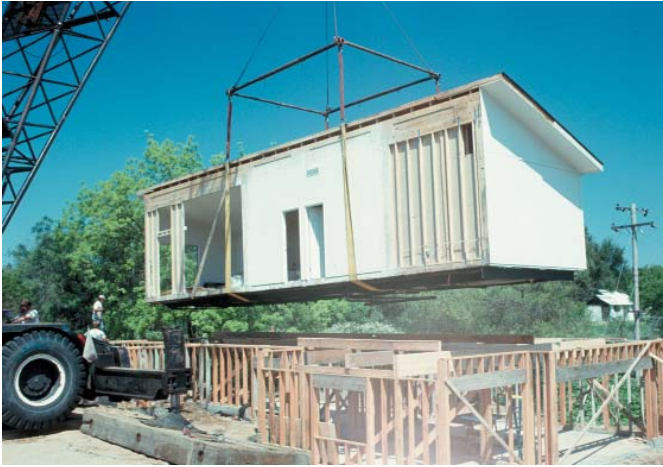
Figure 3.66 Above-ground basement with garage.
