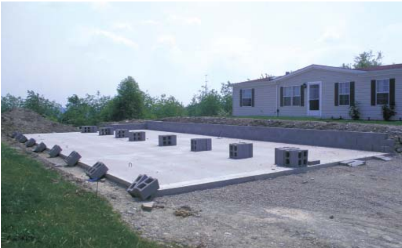
Figure 3.46 The simple design of slabs minimizes the time required for fork work and provides a level base for the home.
