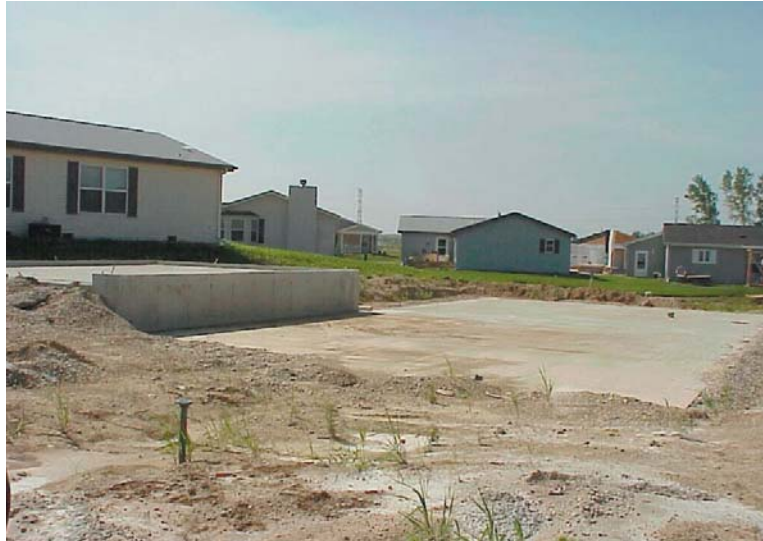
Figure 3.51 Side-by-side slabs for a house and garage. The elevated garage foundation will keep the house and garage floors near each other vertically.
