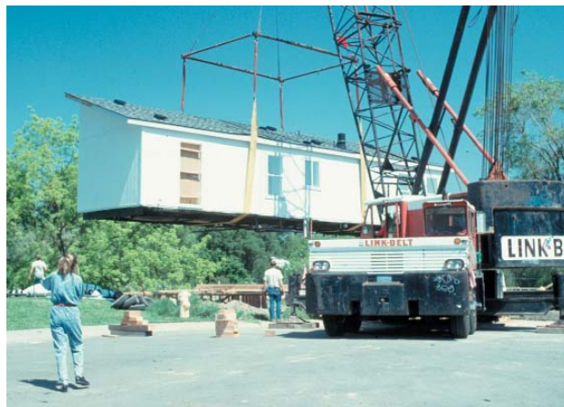
Figure 3.17 Installing a home with a crane.
