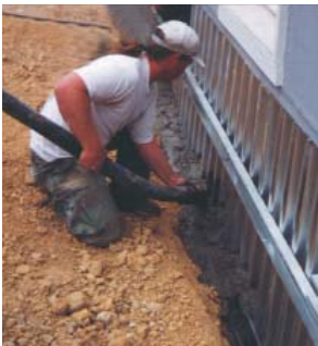
Figure 4.12 Concrete added to the trench.
