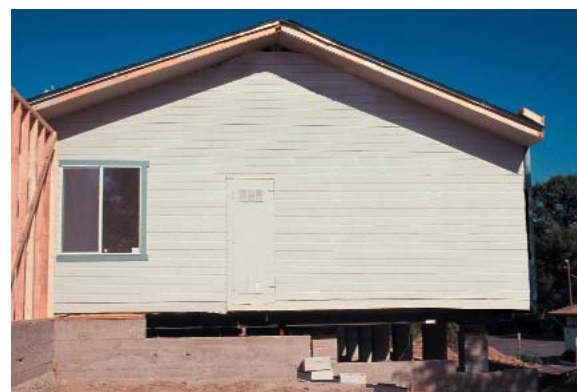
Figure 3.9 Stepped foundation.
