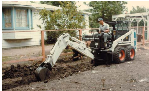
Figure 3.12 Excavating for perimeter footings with a backhoe.
