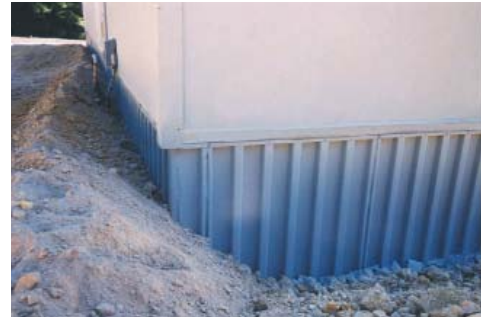
Figure 4.14 The coated panels can safely be backfilled.
