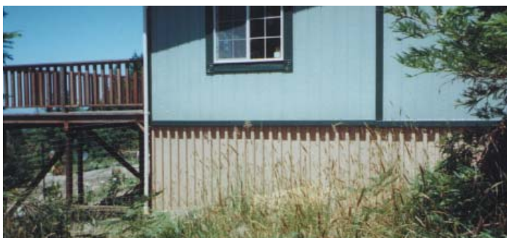
Figure 4.19 View site foundations (with decks) cost less.
