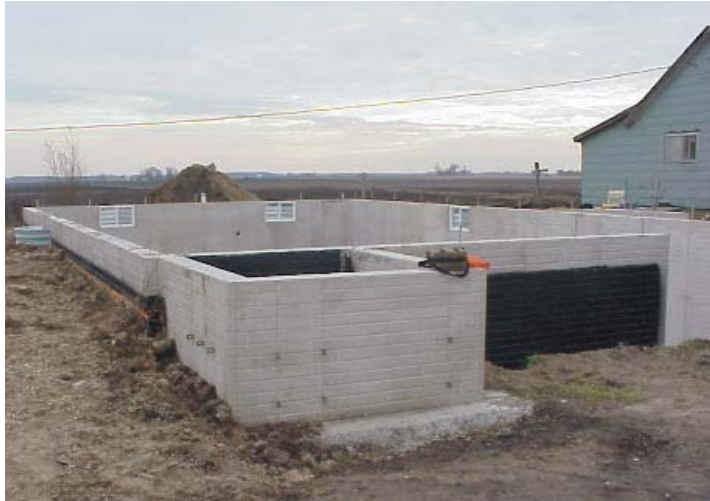
Figure 3.63 Basement showing backfill to create drainage slope.
