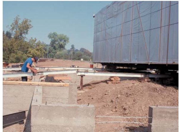
Figure 3.18 Installing a home with a roller system.
